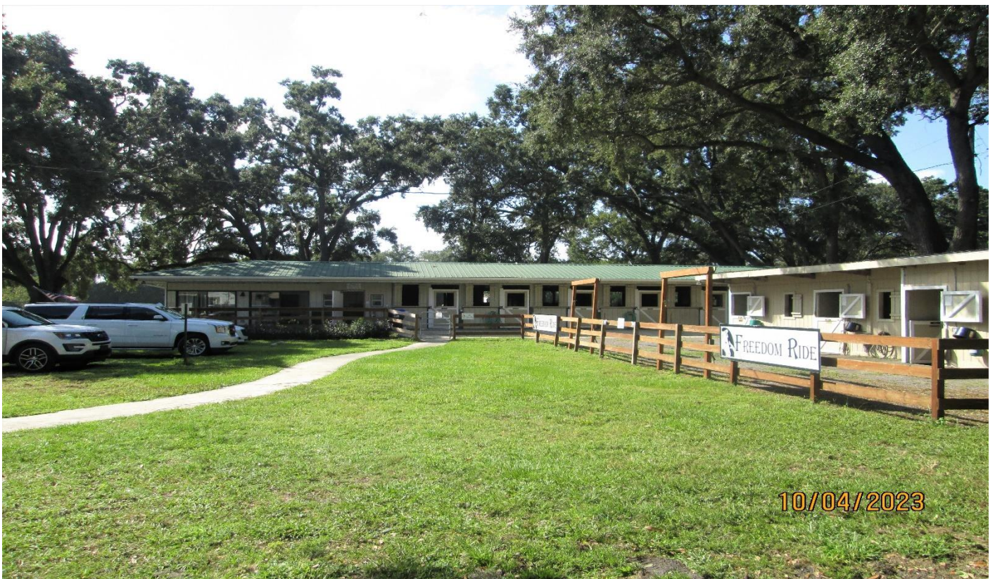
Facing south towards existing horse stable
