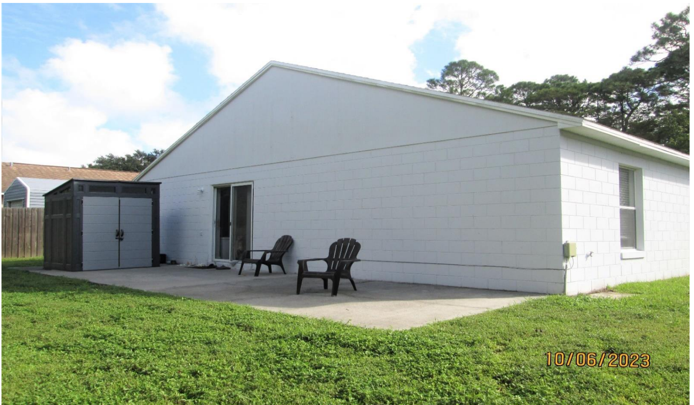
Rear yard, facing northeast towards proposed location of addition
