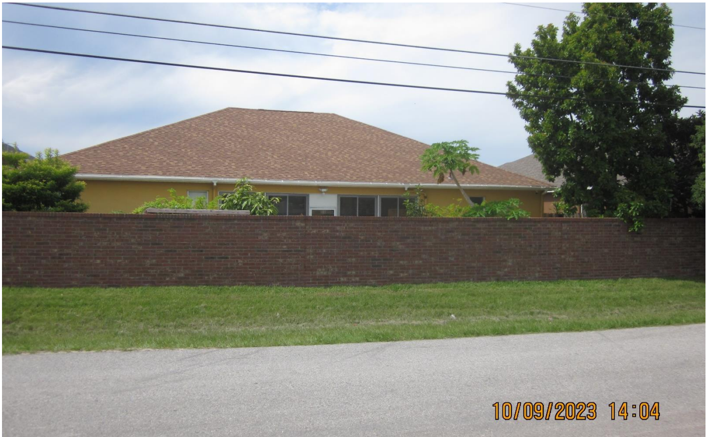
Adjacent homes to the west
