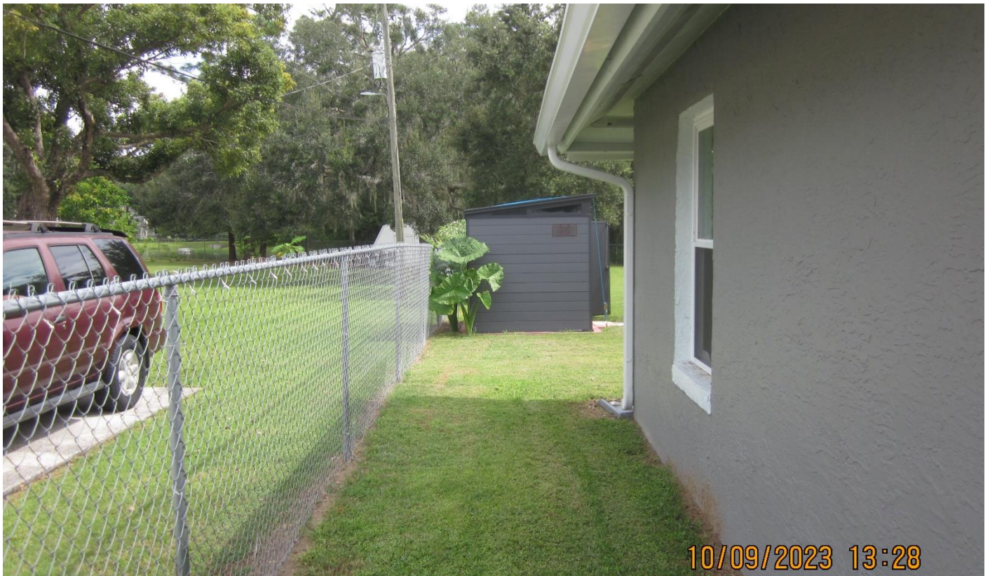
Existing 7 ft. north side setback facing east
