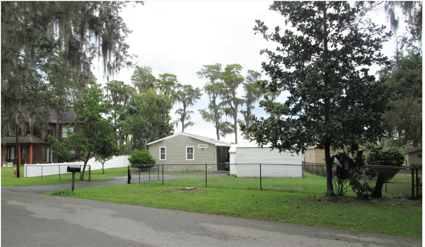
Facing northwest from Arrowhead Blvd. towards front of subject property
