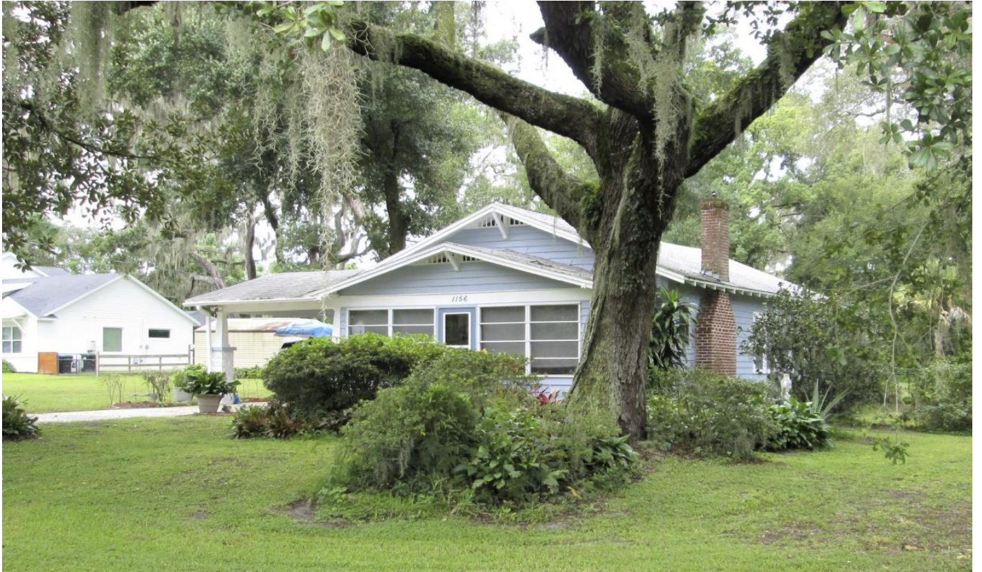
Existing house subject to Variances, facing west from Mill Street
