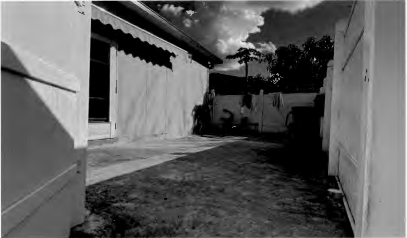
Side yard, facing northeast towards addition (note concrete pavement)
