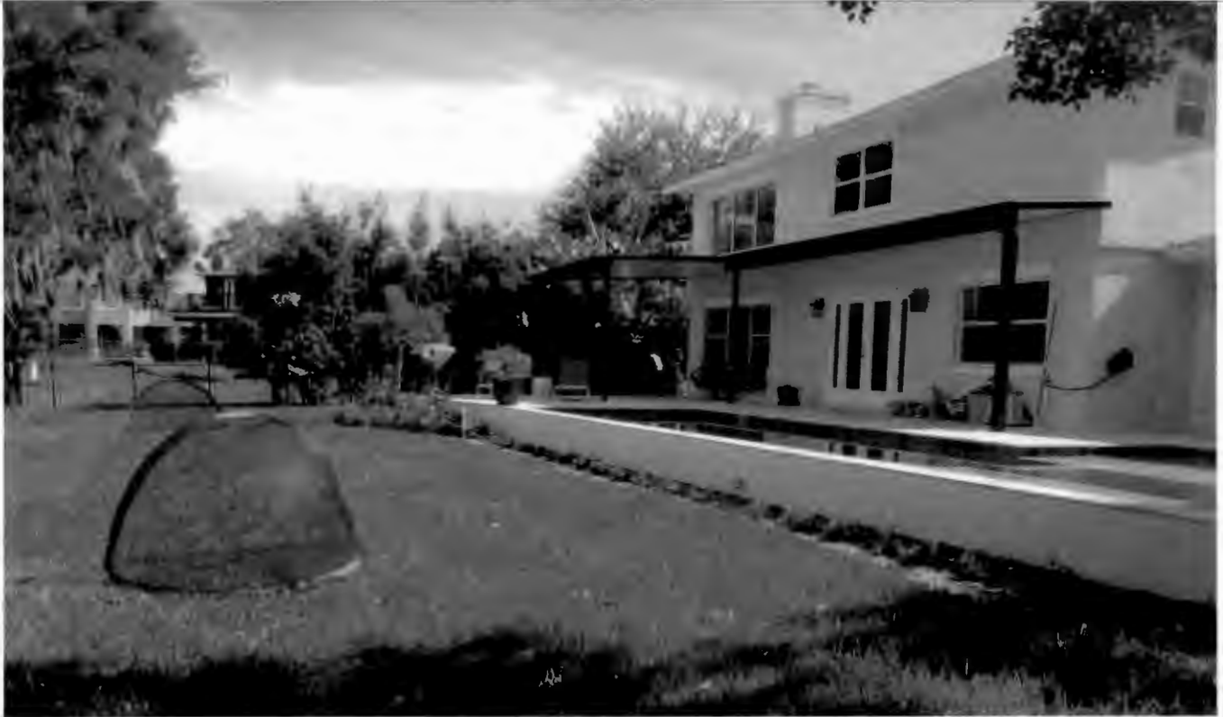
Covered porch facing east
