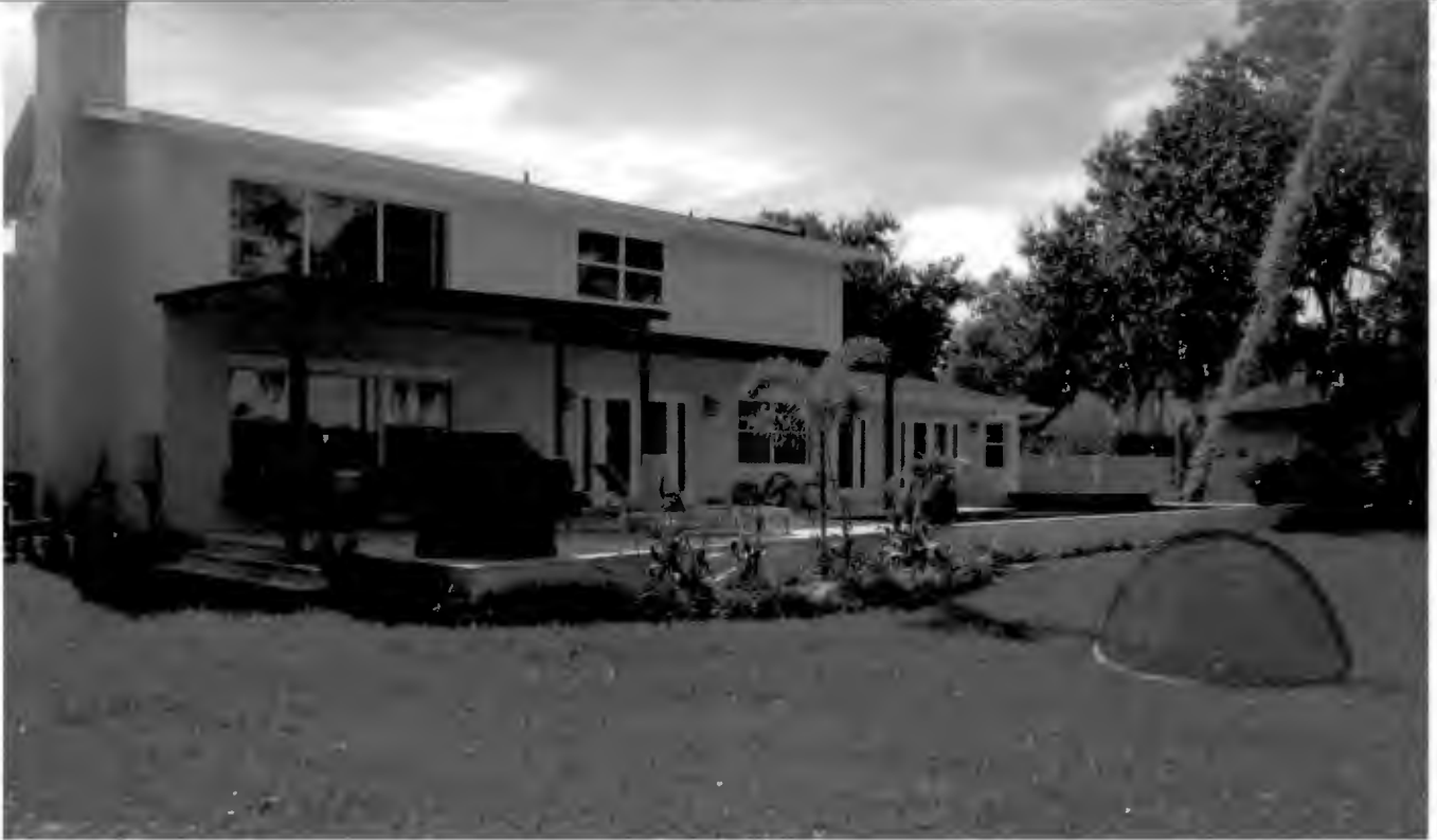
Covered porch facing south
