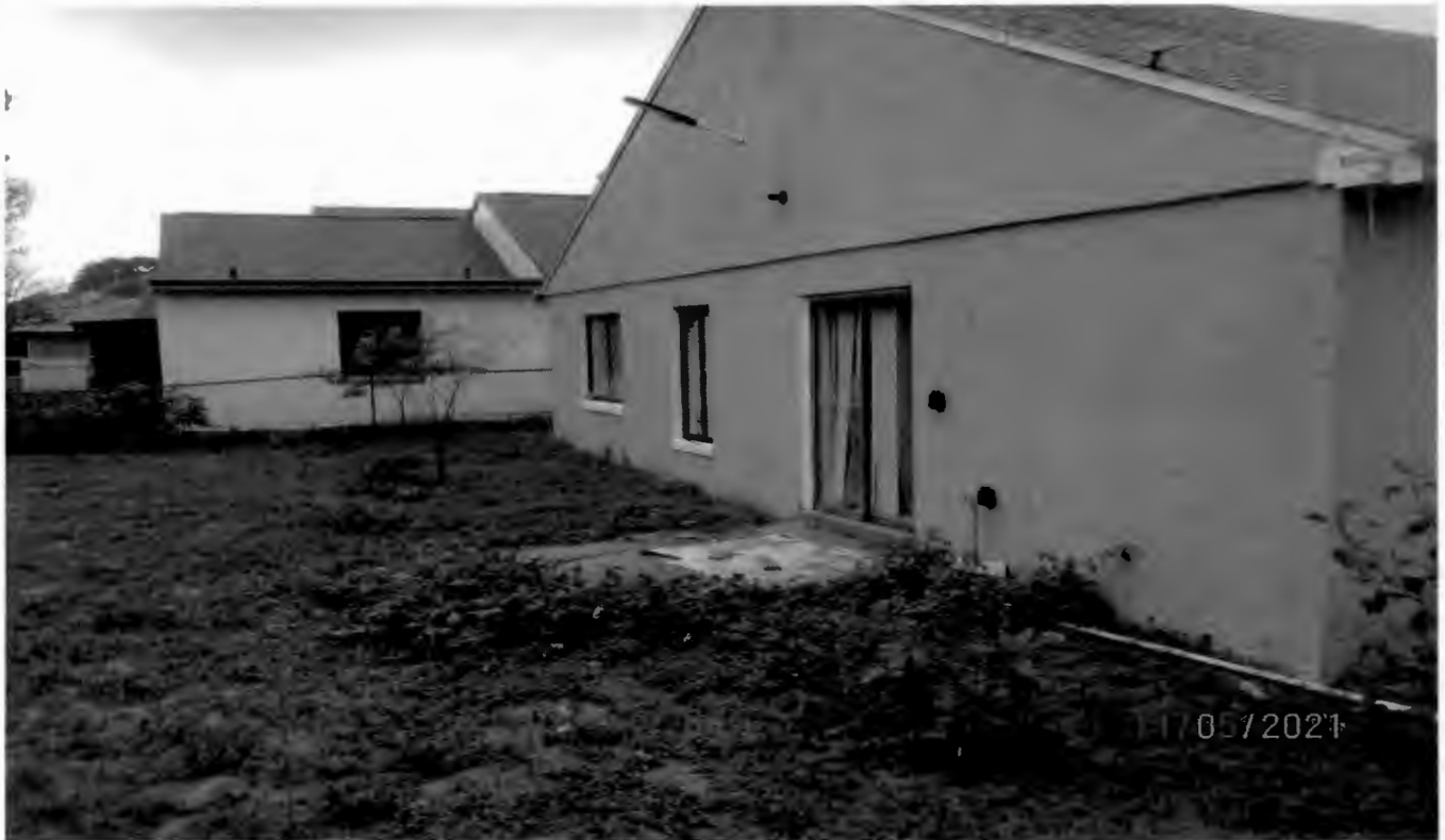
Location of proposed addition facing south
