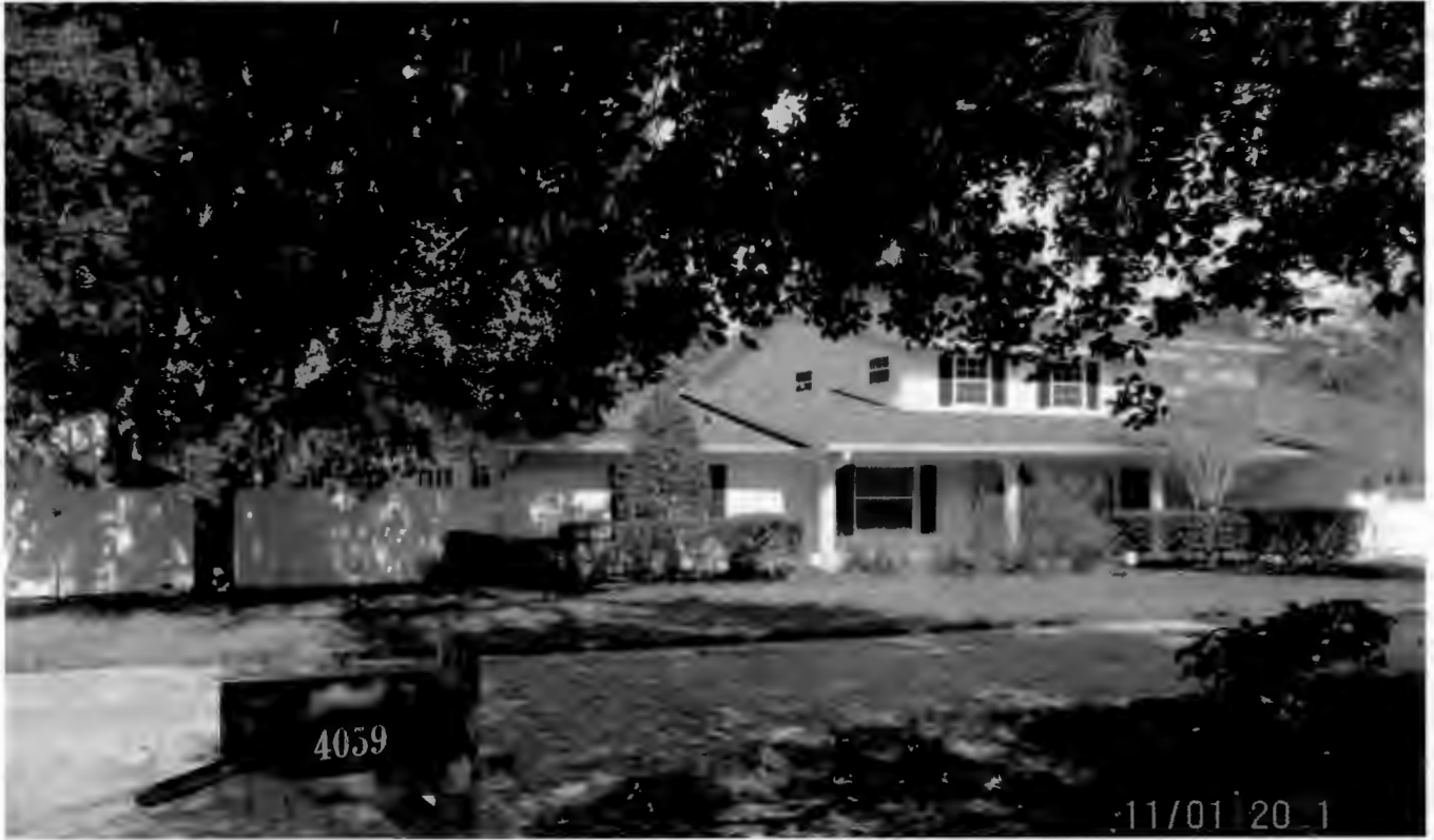
Front from Cool Water Ct. facing north
