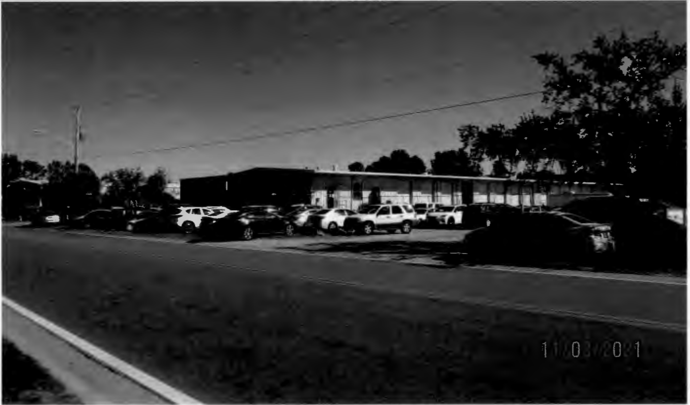
Facing northeast towards subject property and proposed billboard along Rocket Blvd.
