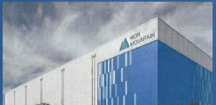
IMDC Miami Data Center
