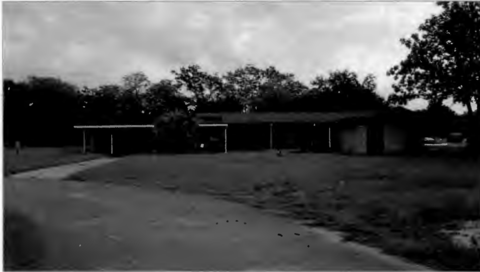
Subject Site – Church
