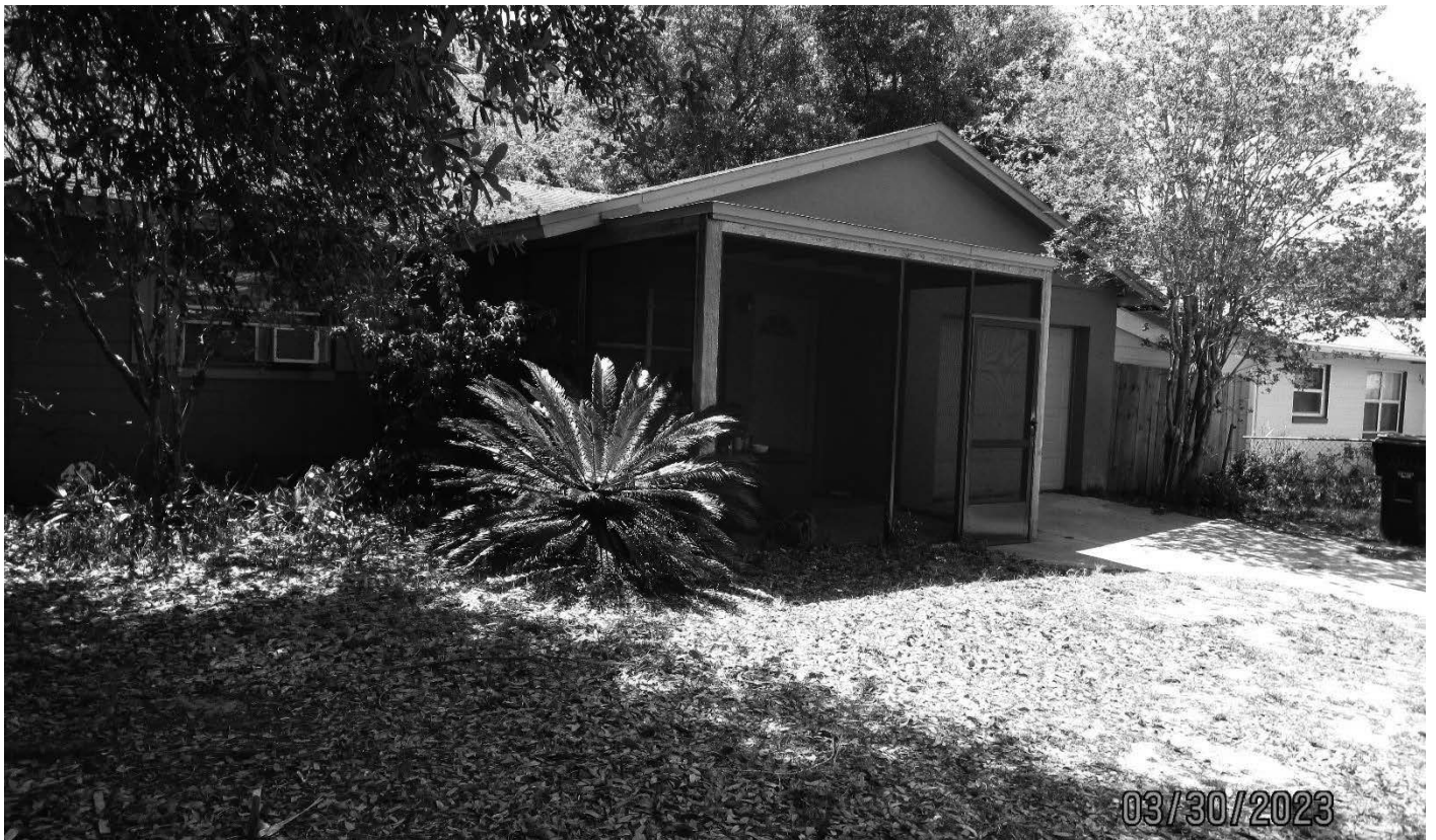
Addition facing west
