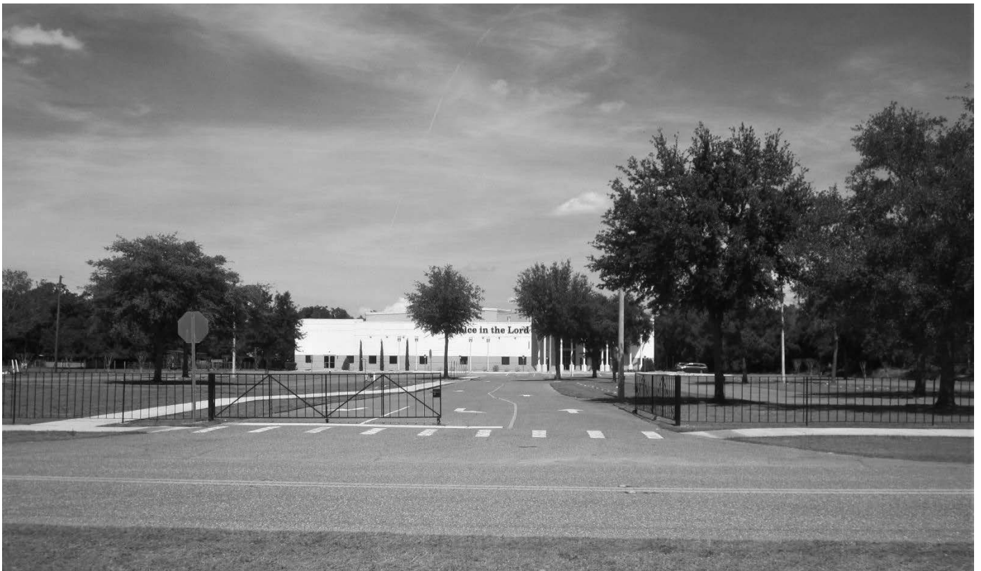
Facing north from Gilliam Rd. towards front of subject property
