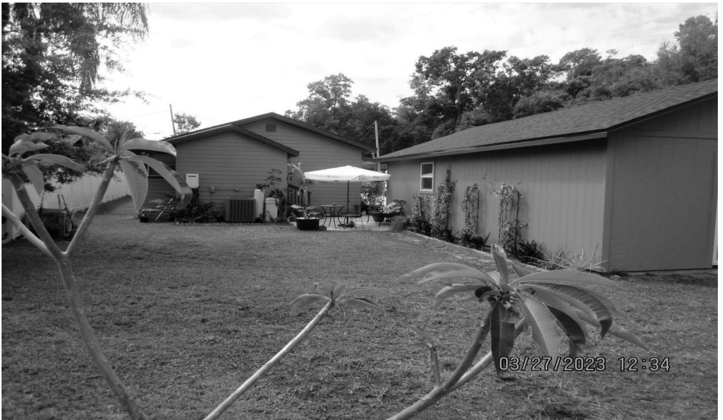
Rear yard, facing south toward the rear of the residence and side of proposed ADU
