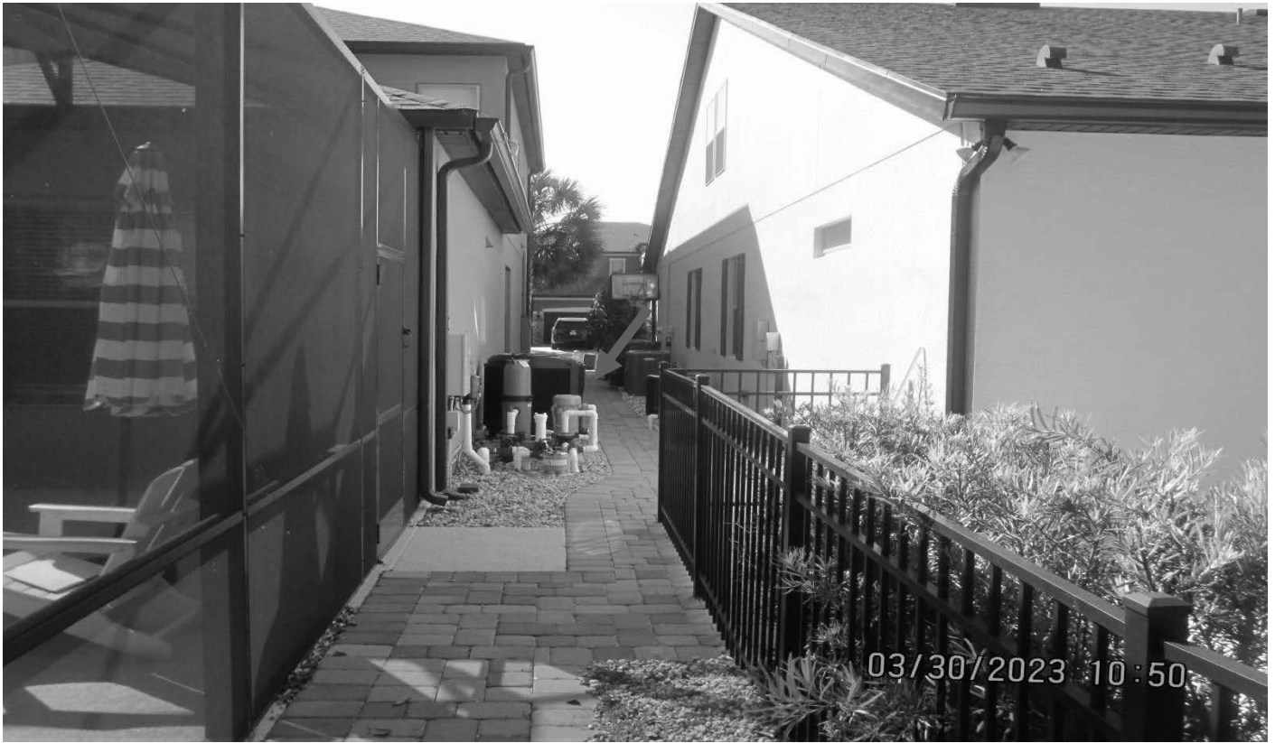
West side – Existing pool equipment location, facing south
