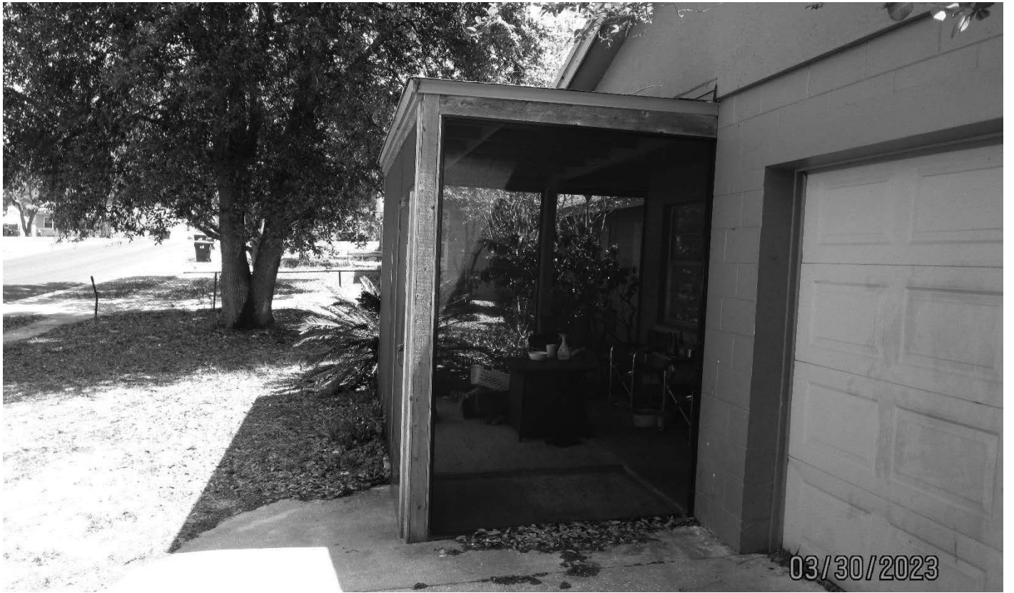
Addition facing east
