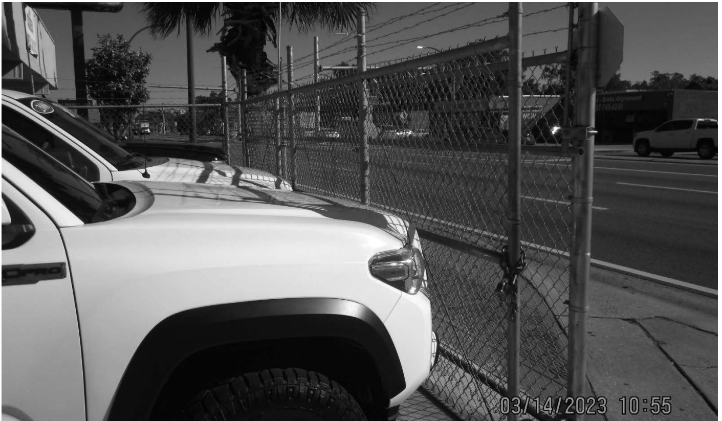
Fence and gate along S. Orange Blossom Trl. facing northeast
