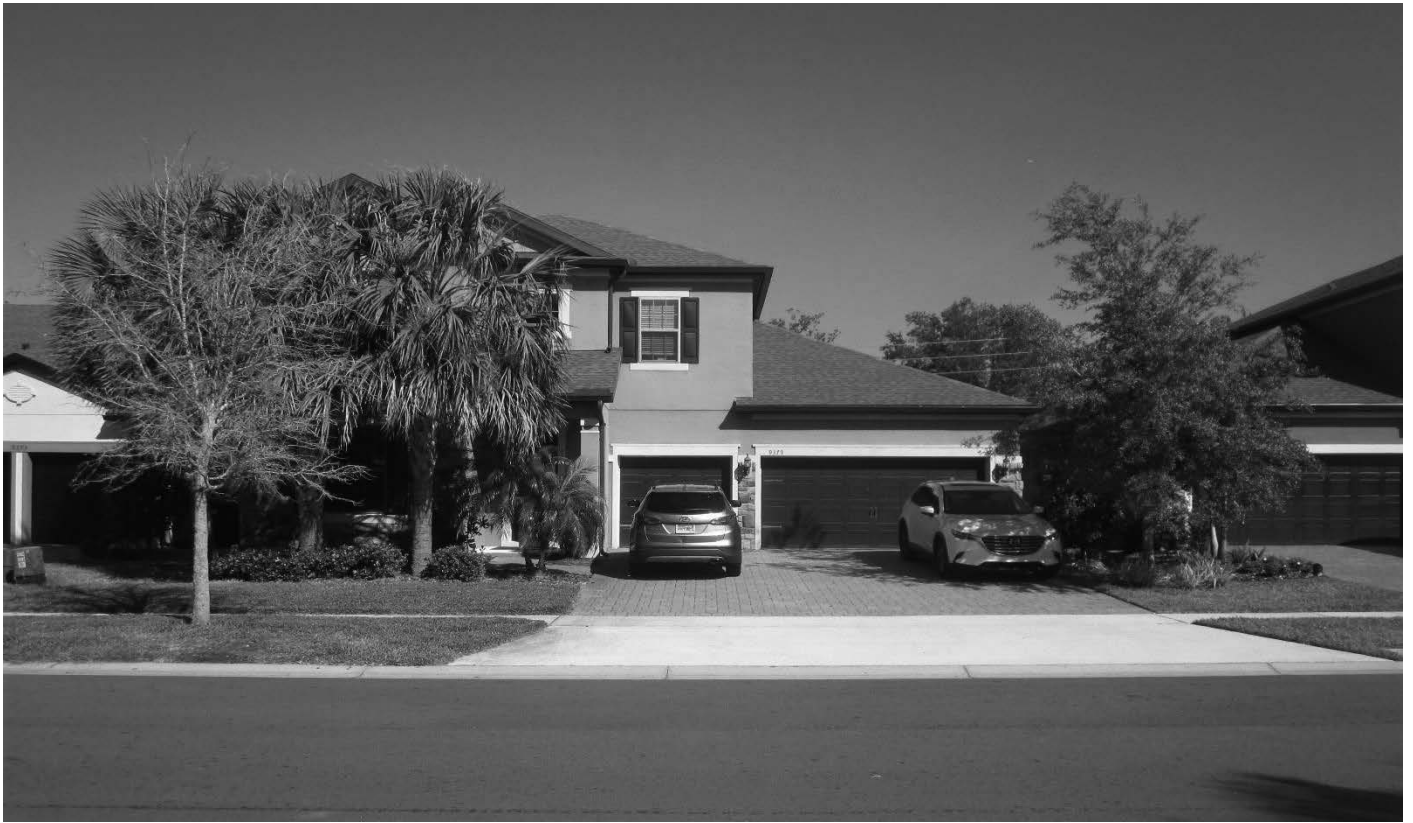
Facing north from Royal Estates Blvd. toward the front of subject property
