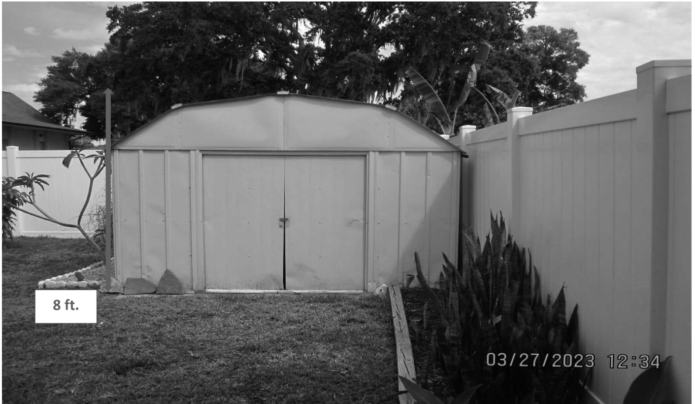
Rear yard, facing south toward the front of the shed (Vairance #3)
