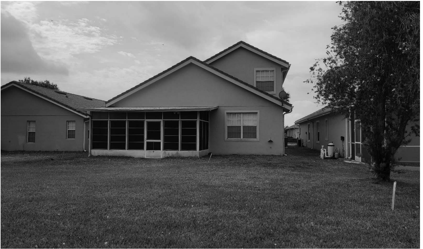
Facing south towards rear of subject property; existing screen room
