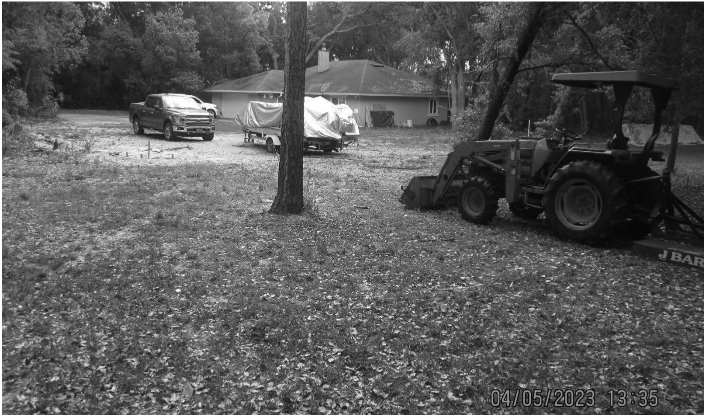
Garage location facing east
