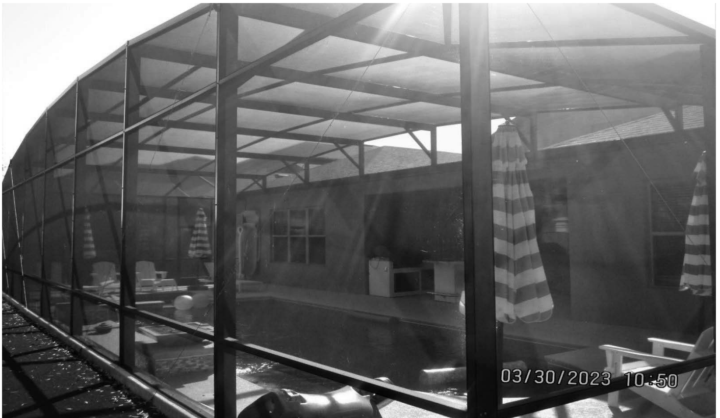
West side - Rear yard with pool/spa and screen enclosure, facing east
