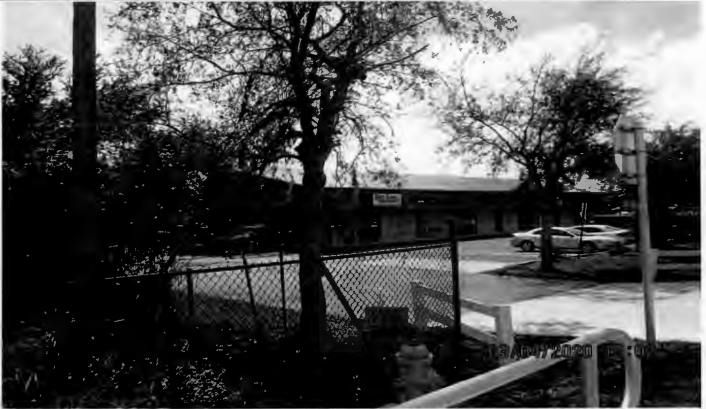
Adjacent business abutting west side of site, looking southwest
