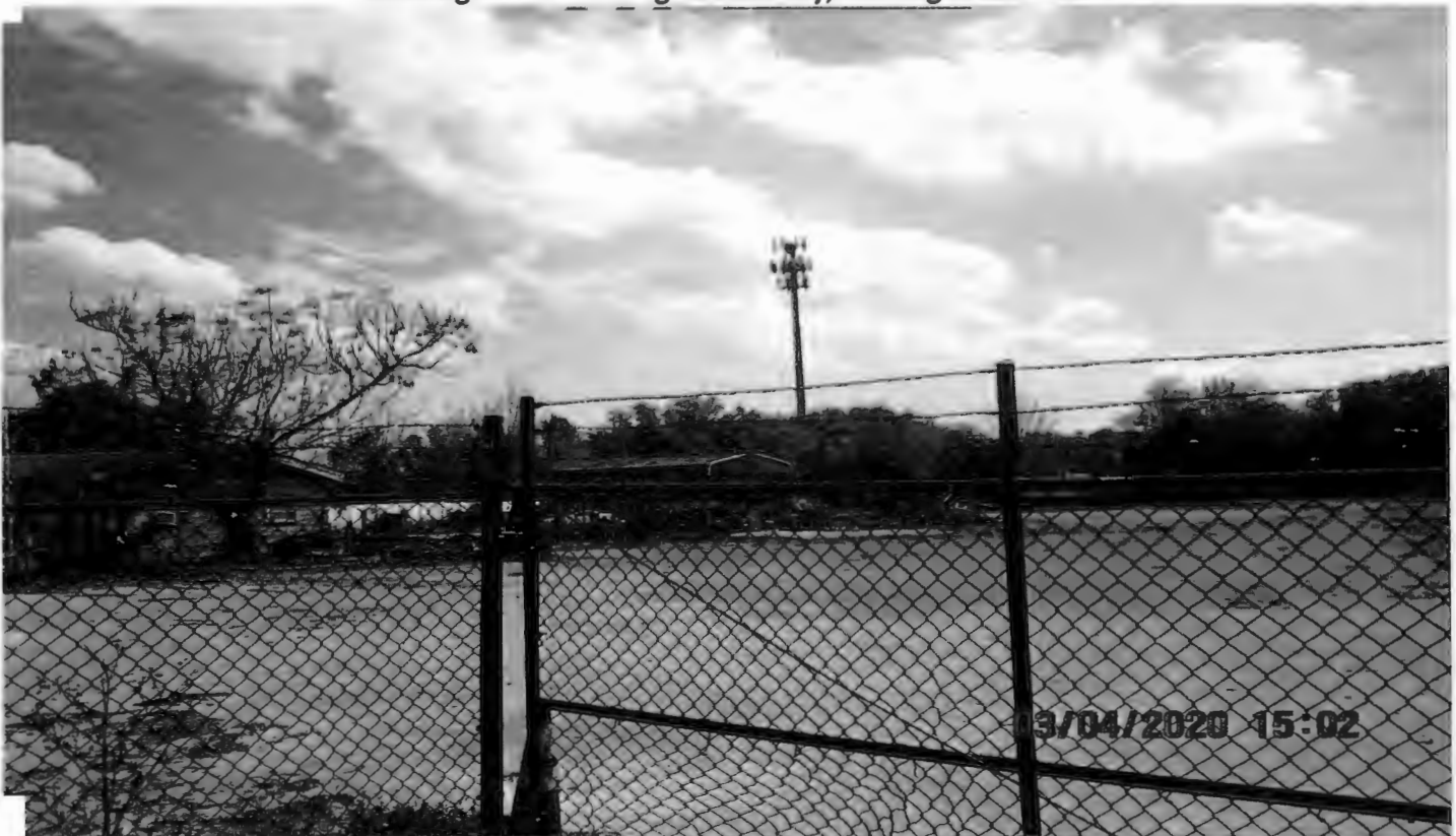
Site work yard with adjacent cell tower in background, looking southeast
