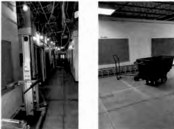
Figure 4. Lila Mitchell Center After Renovations
