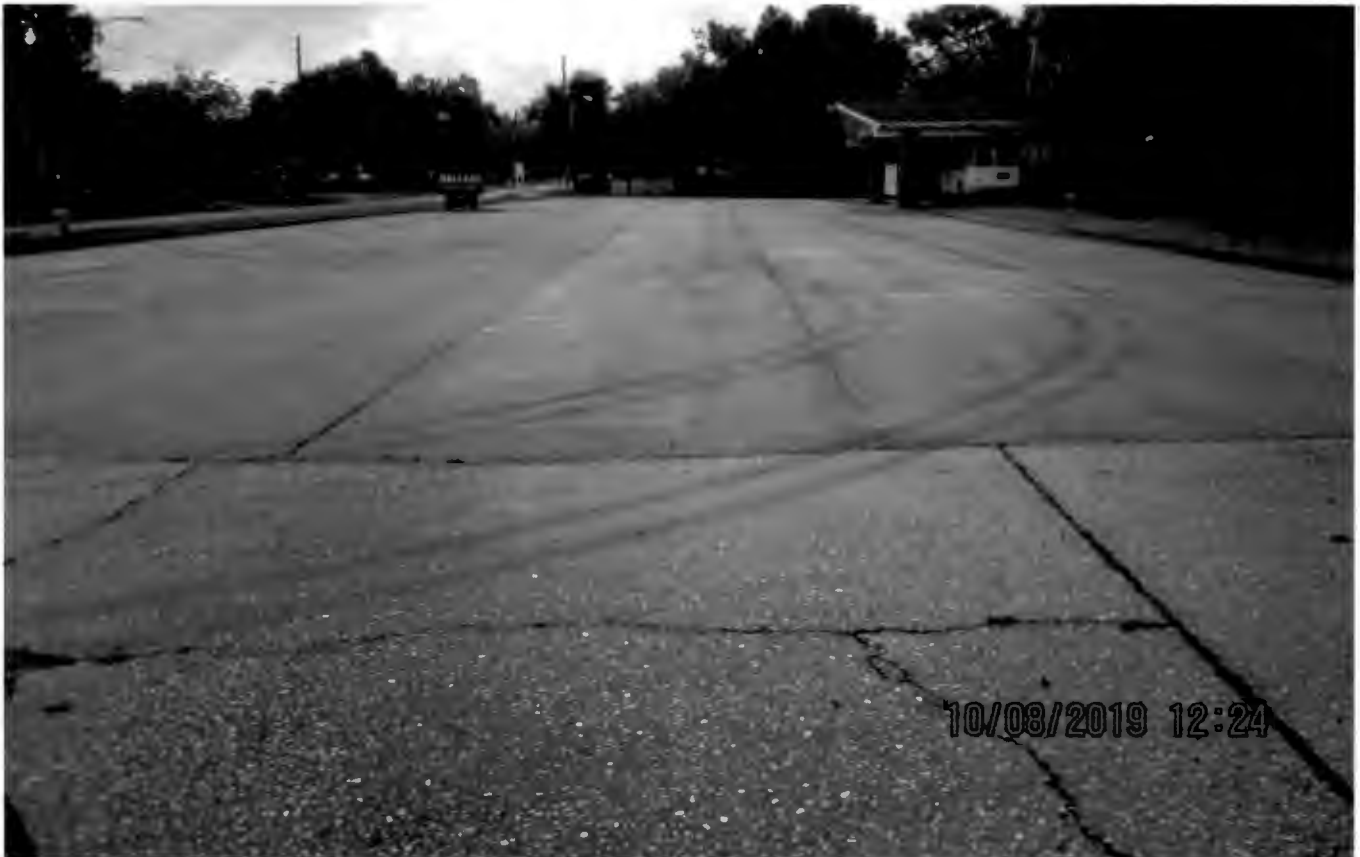
Front Parking Lot
