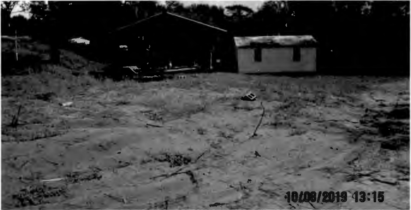
Pole Barn and Shed that will be removed
