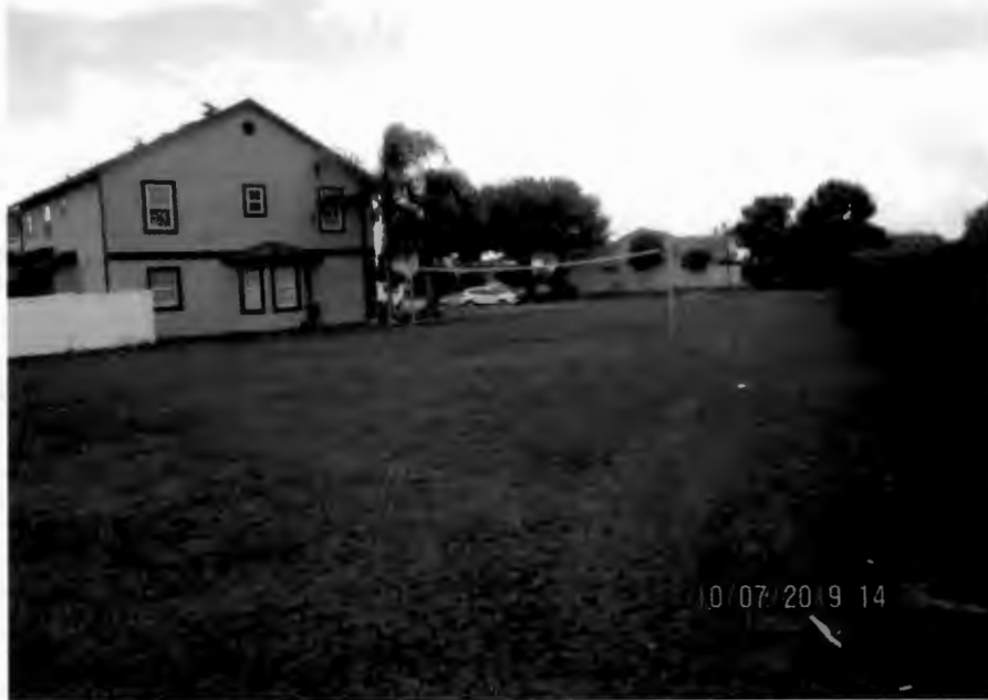
Subject Property Looking Southeast. Bay Window to Left
