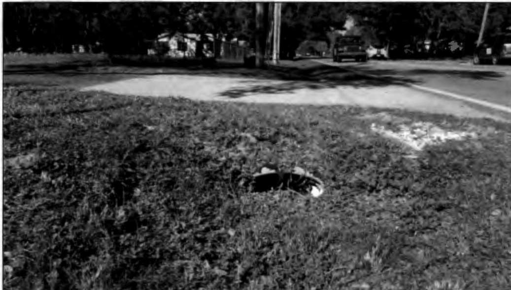
Figure 3.11: Drainage Features Along Southbound Roadside Ditch
