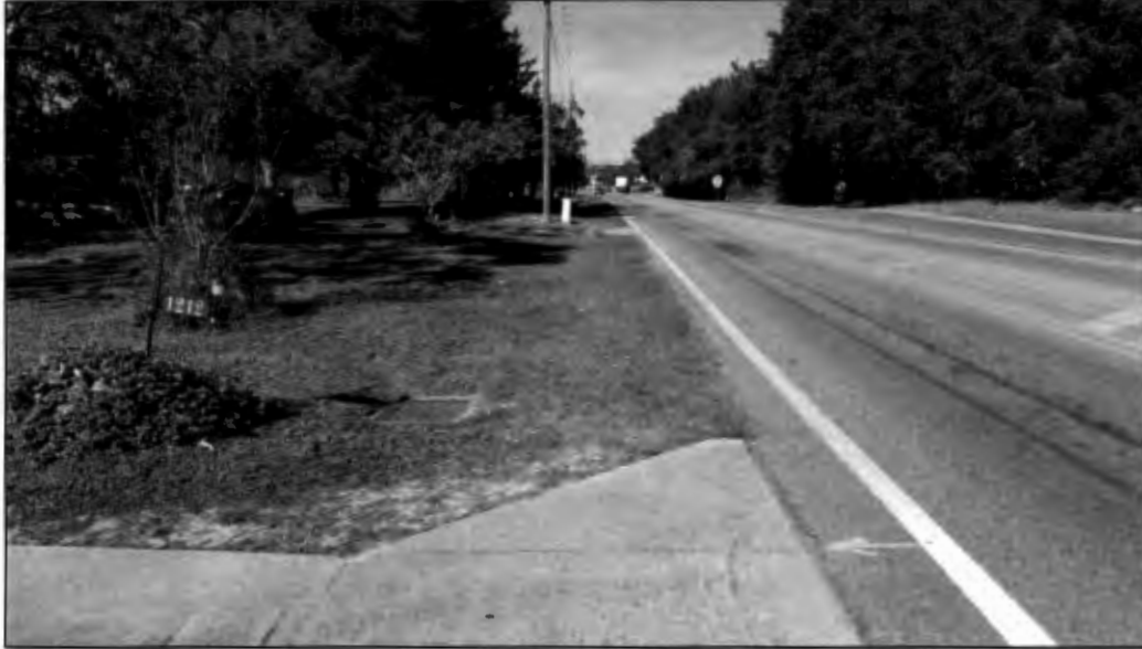
Figure 3.12: Drainage Features Along Southbound Roadside Ditch
