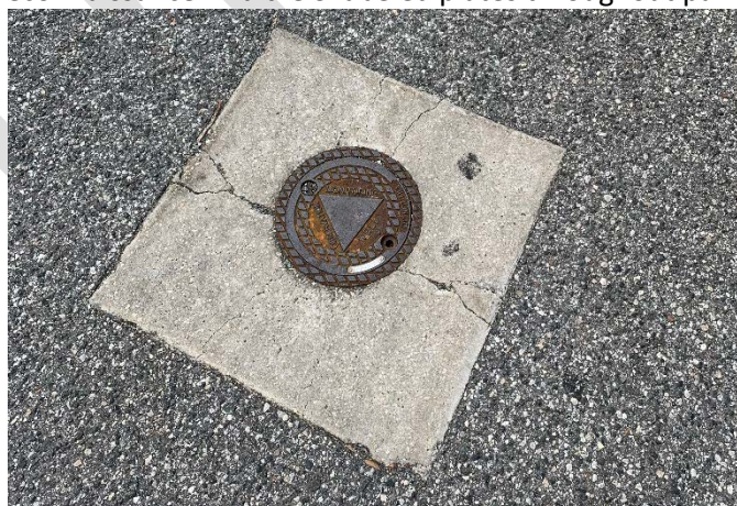
Site No. 24 – Walgreens Site Reconnaissance: Multiple monitoring wells throughout parking lot
