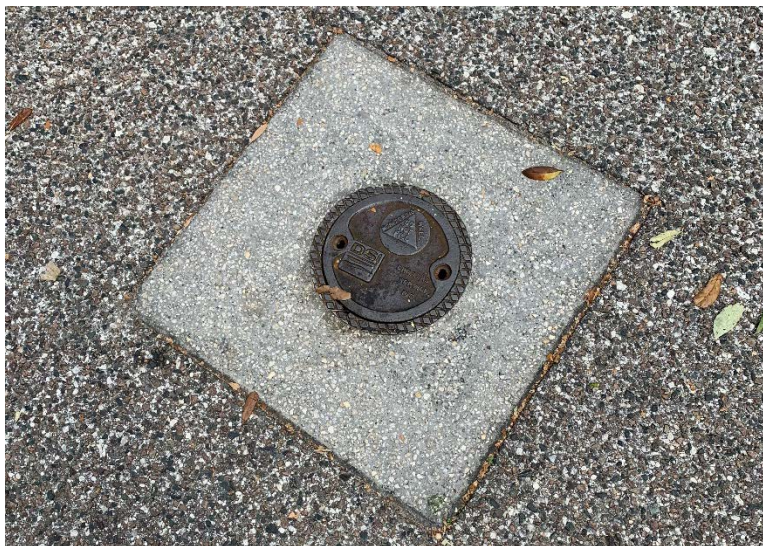
Site No. 8 – BP/Circle K Gas Station Site Reconnaissance: Multiple monitoring wells throughout parking lot
