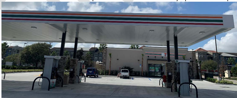
Site No. 30 – 7-Eleven Site Reconnaissance: Active 7-Eleven Gas Station
