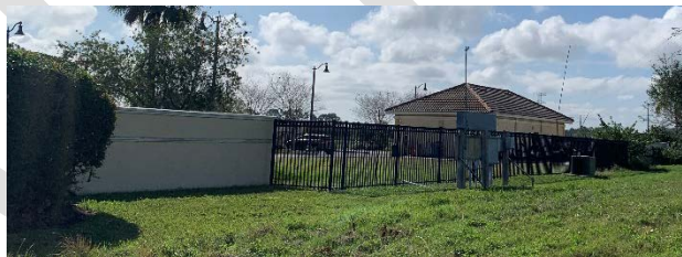
Site No. 26 – Orange County Universal PS #3995 Site Reconnaissance: Apartment Complex Utilities based on FDEP MapDirect location
