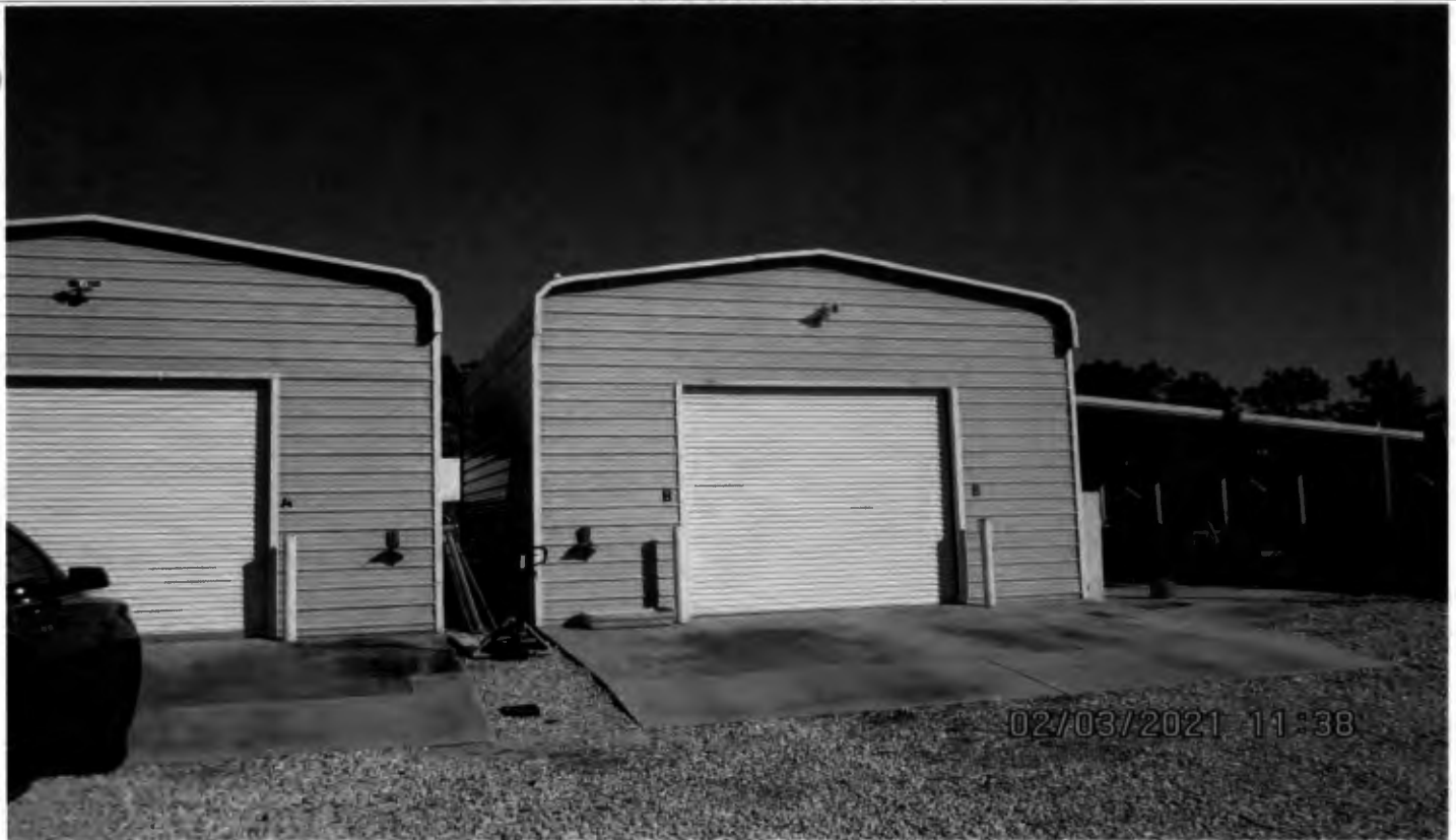
Garage requiring variance at right looking north
