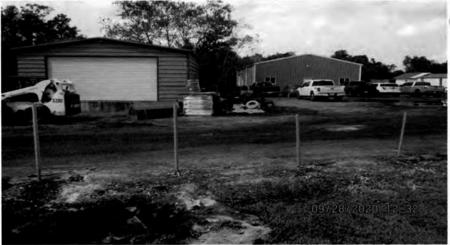
Bldg. A-633 sq. ft. shed, and Bldg. C-3,000 sq. ft. Office-Warehouse, looking west
