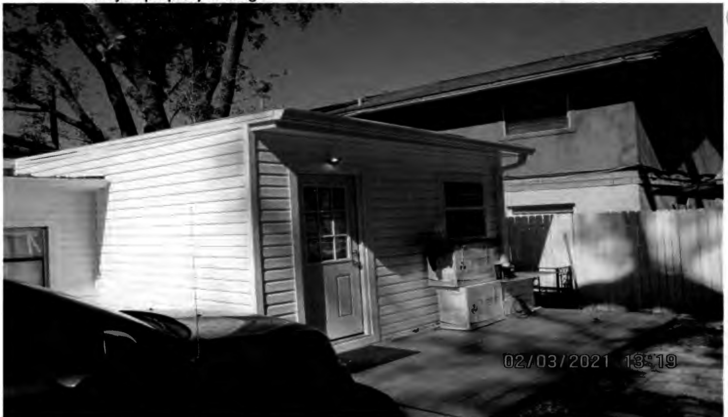
Original house left, addition right looking northwest from rear yard
