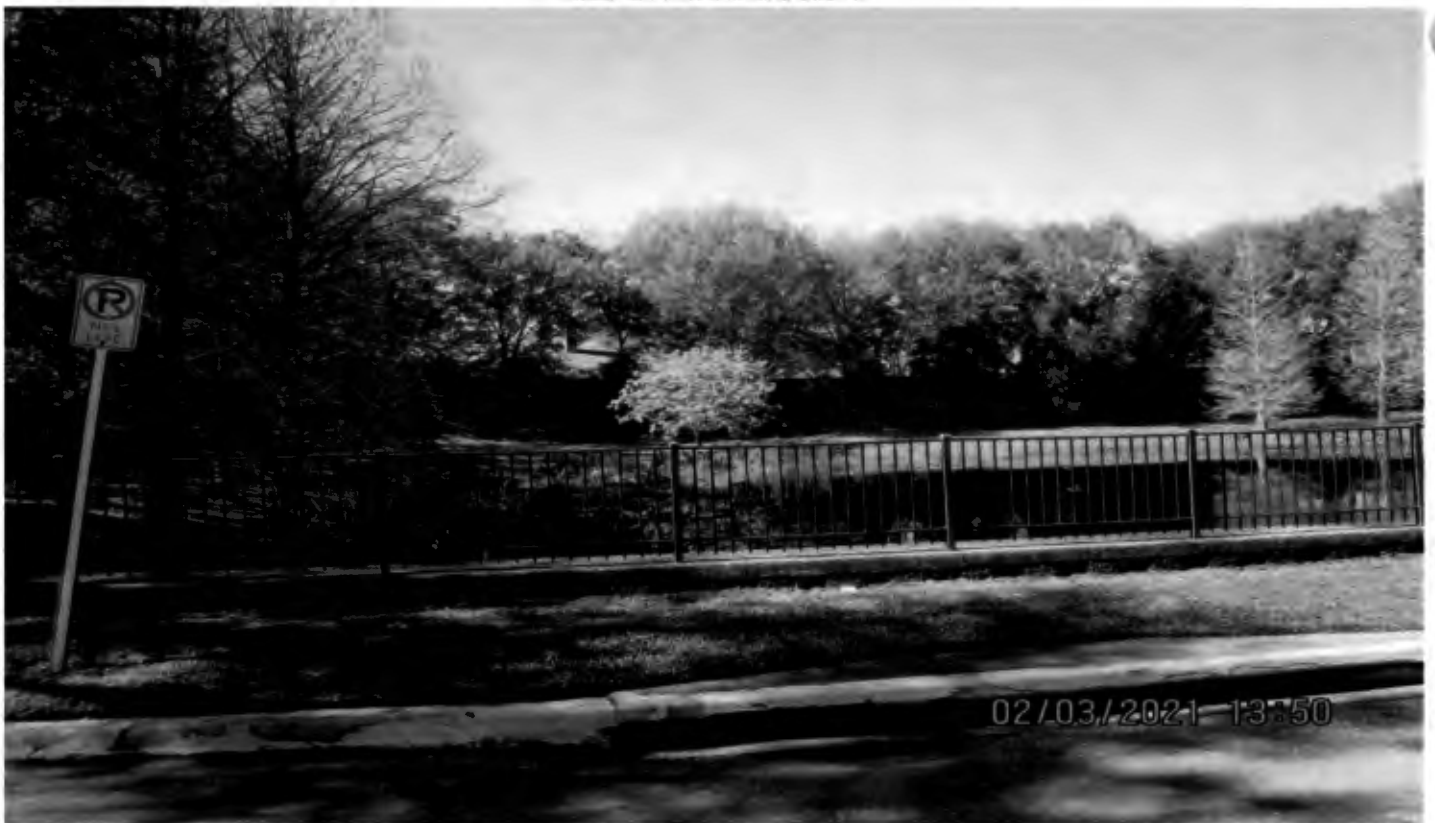
Stormwater retention pond looking west from behind hardware store
