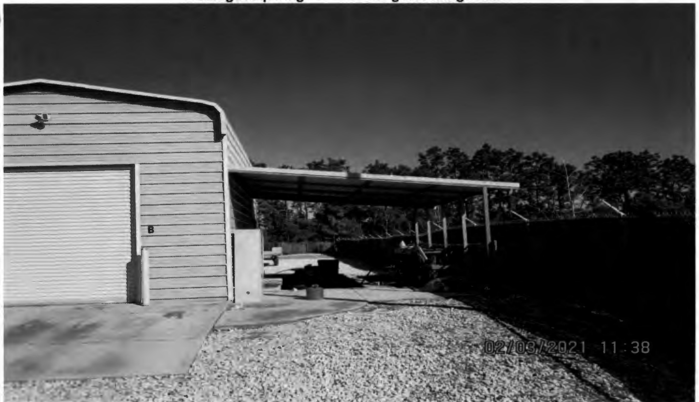
Carport proposed to be removed looking north
