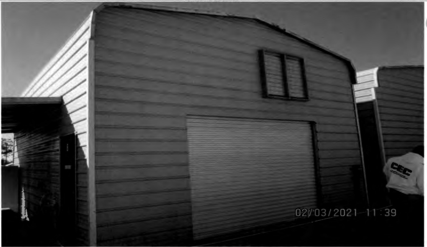
Rear of garage requiring variance looking south
