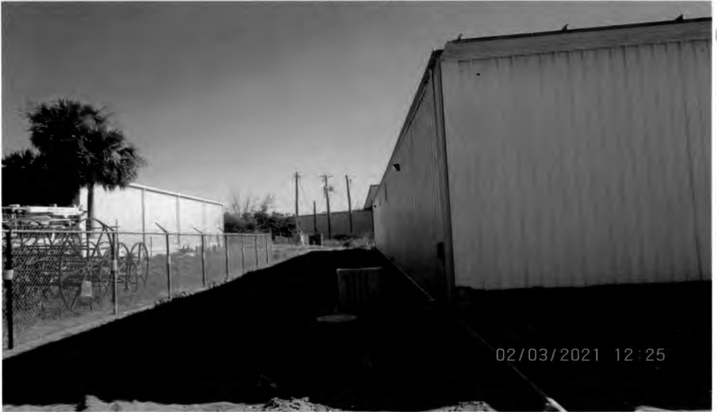
Existing deficient rear (north) setback looking east
