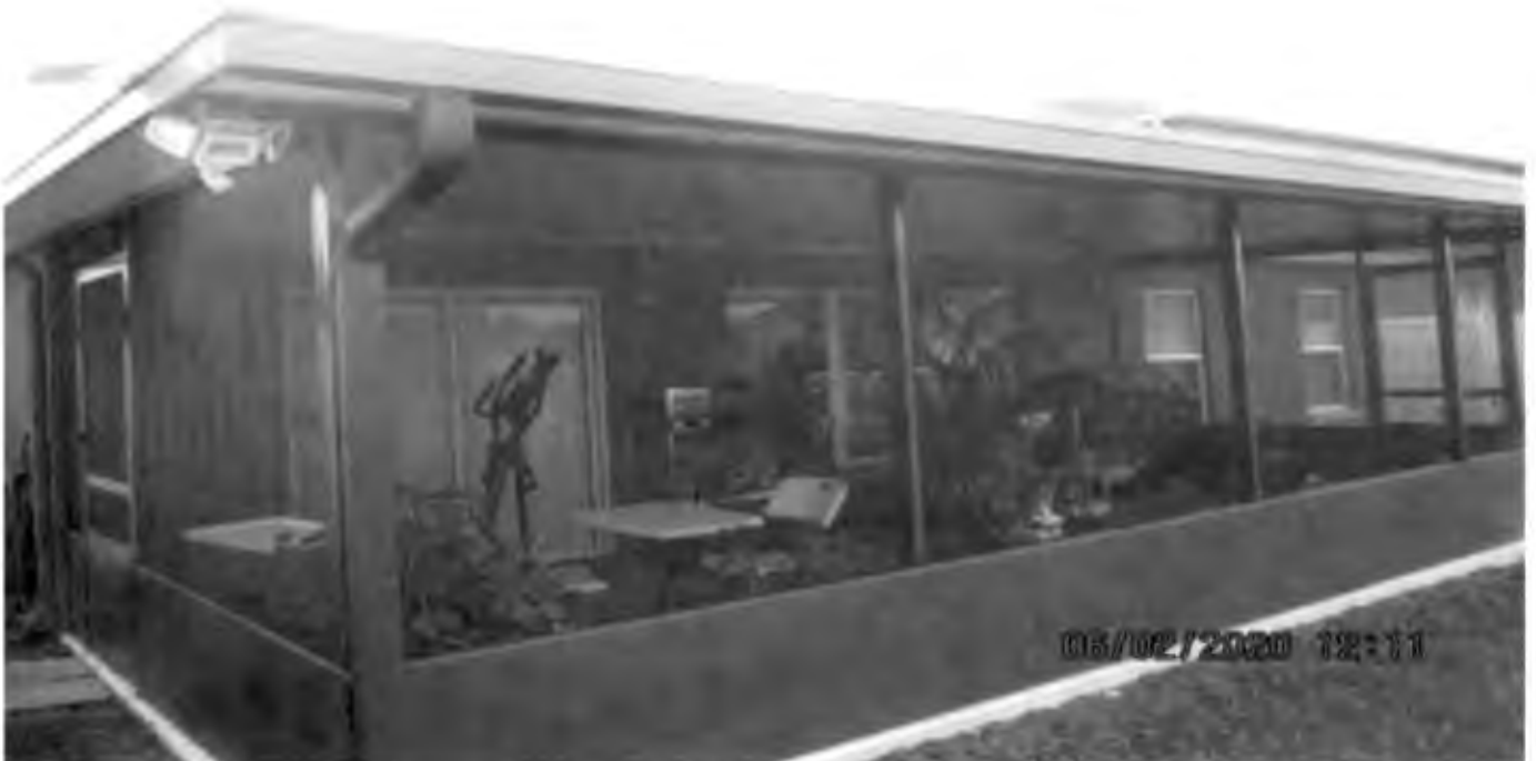
Existing screen room looking southeast
