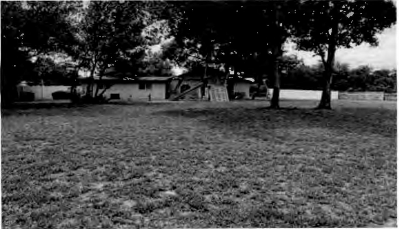
Rear of the house looking toward the proposed parking area entrance and parking area
