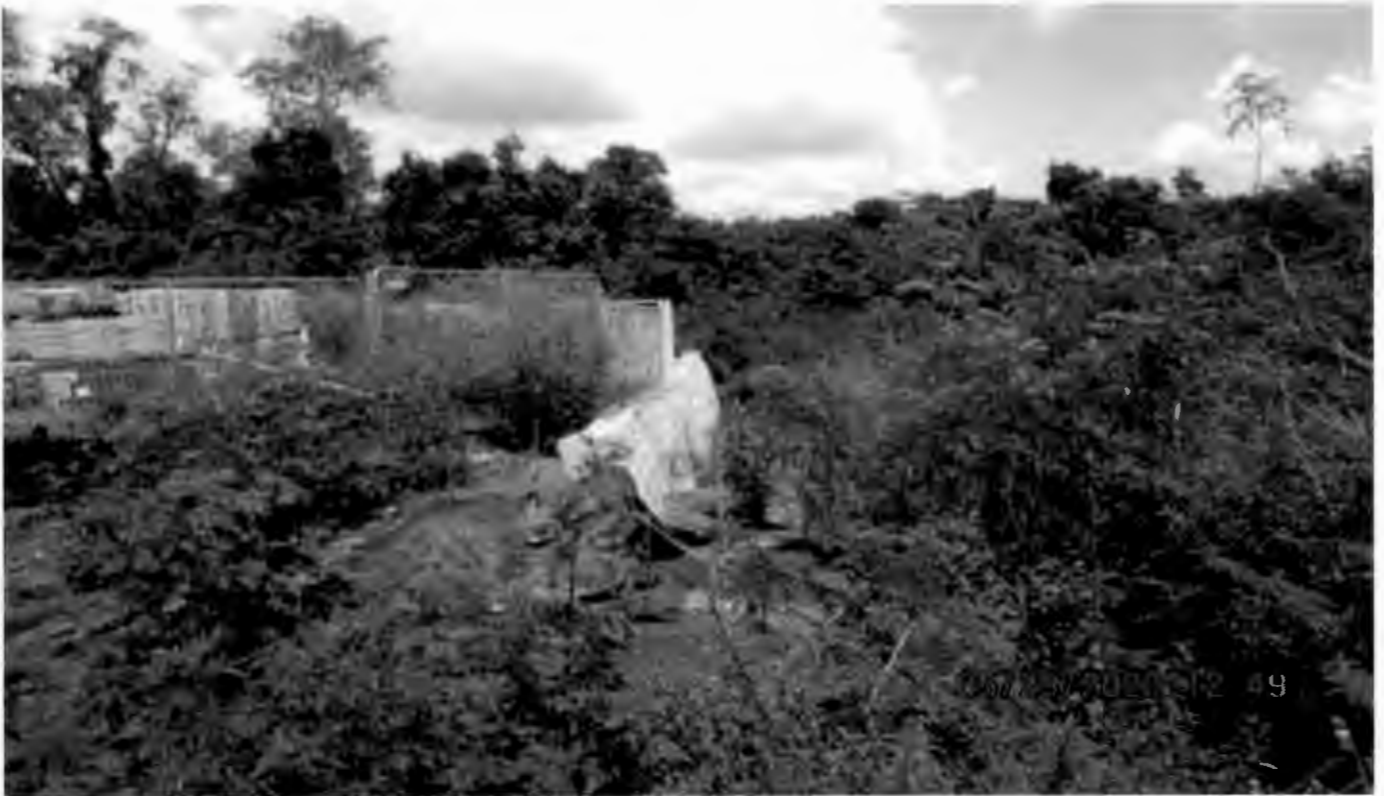
Retaining wall south of site
