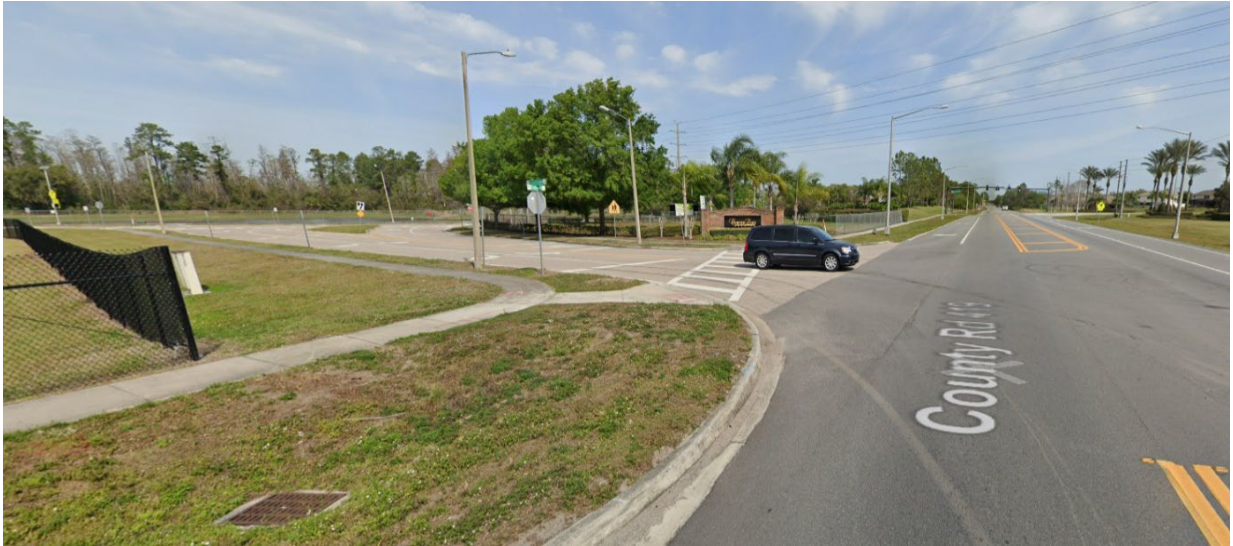
Chuluota Road and Schoolview Way showing ditch bottom inlet which drains to existing pond
