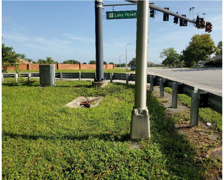
Ditch bottom inlet at southwest intersection of Lake Pickett Road and Chuluota Road, facing north
