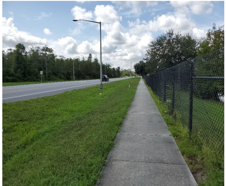
Roadside ditch facing south
