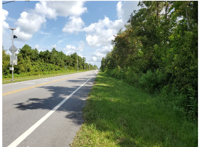
Roadside ditch facing north
