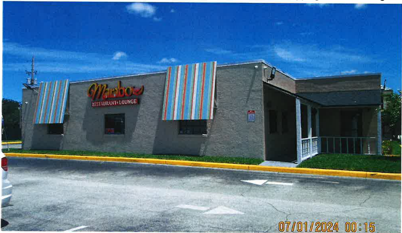
Facing north from W. Oak Ridge Rd. towards entry of subject building
