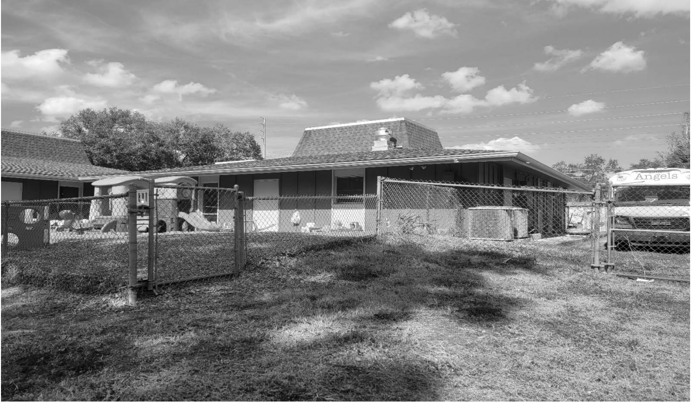
Rear yard, facing northwest towards proposed addition location
