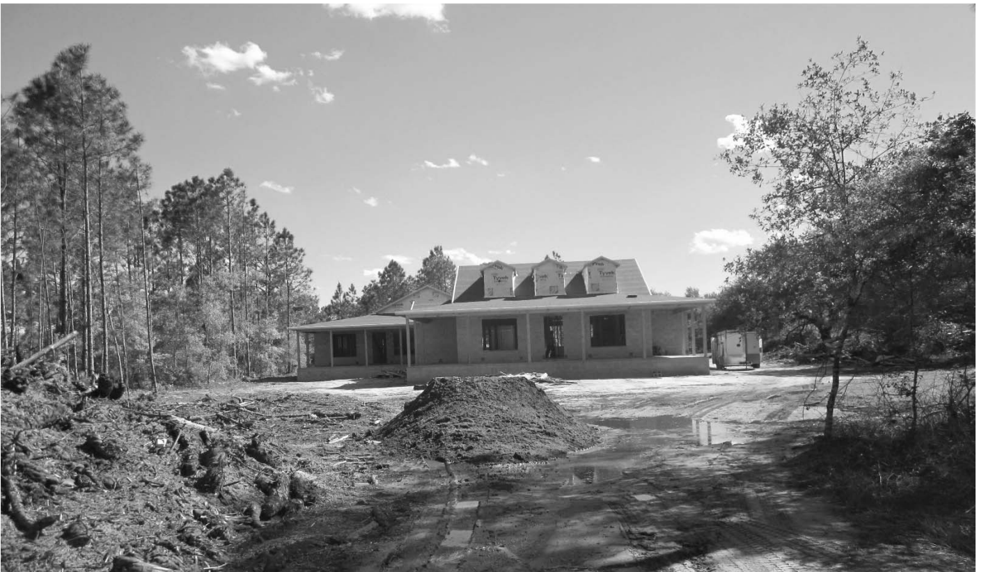
Facing south towards new main residence (under construction)
