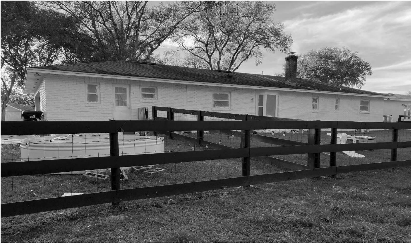
Facing west towards rear of subject property
