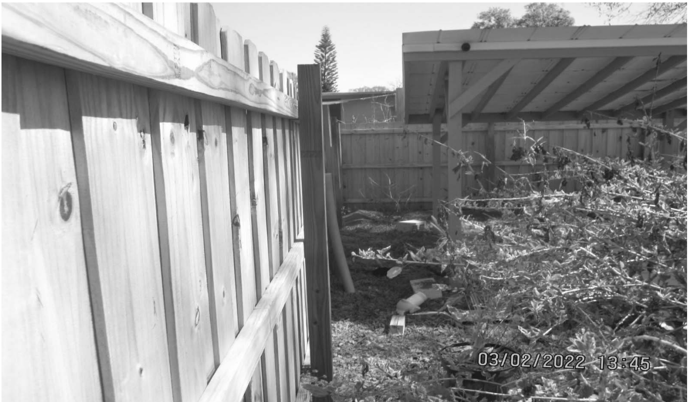
Rear yard, facing east towards side of covered patio
