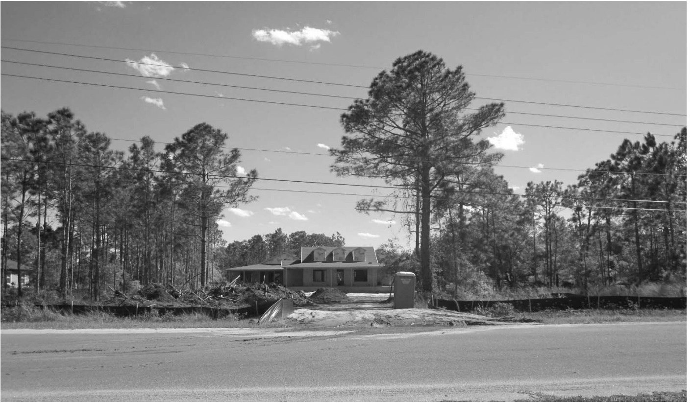
Facing south towards front of subject property
