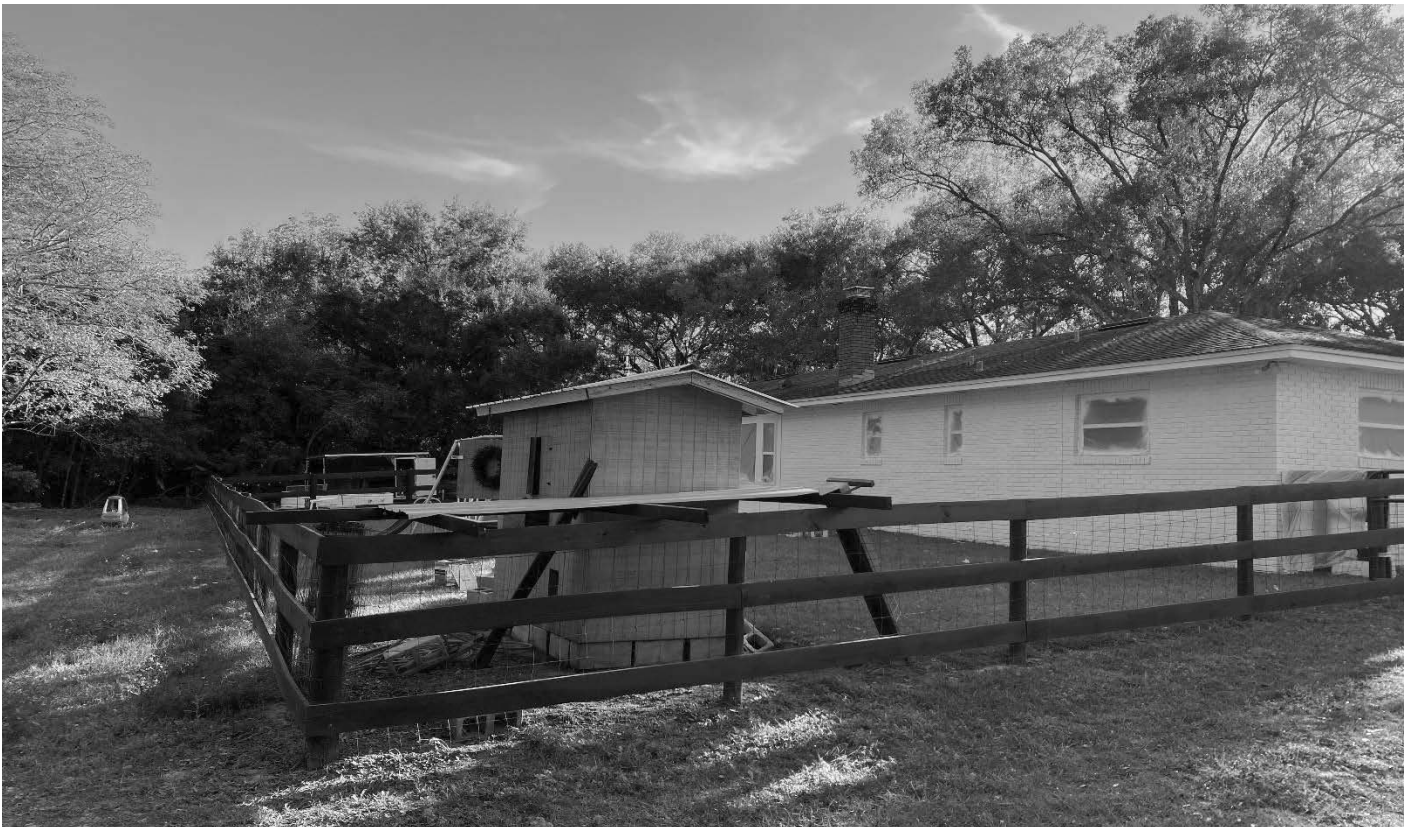
Facing south towards rear of subject property
