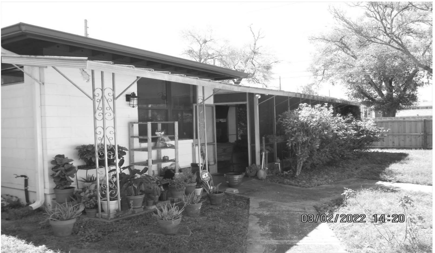
Rear yard, facing southwest towards the proposed sunroom
