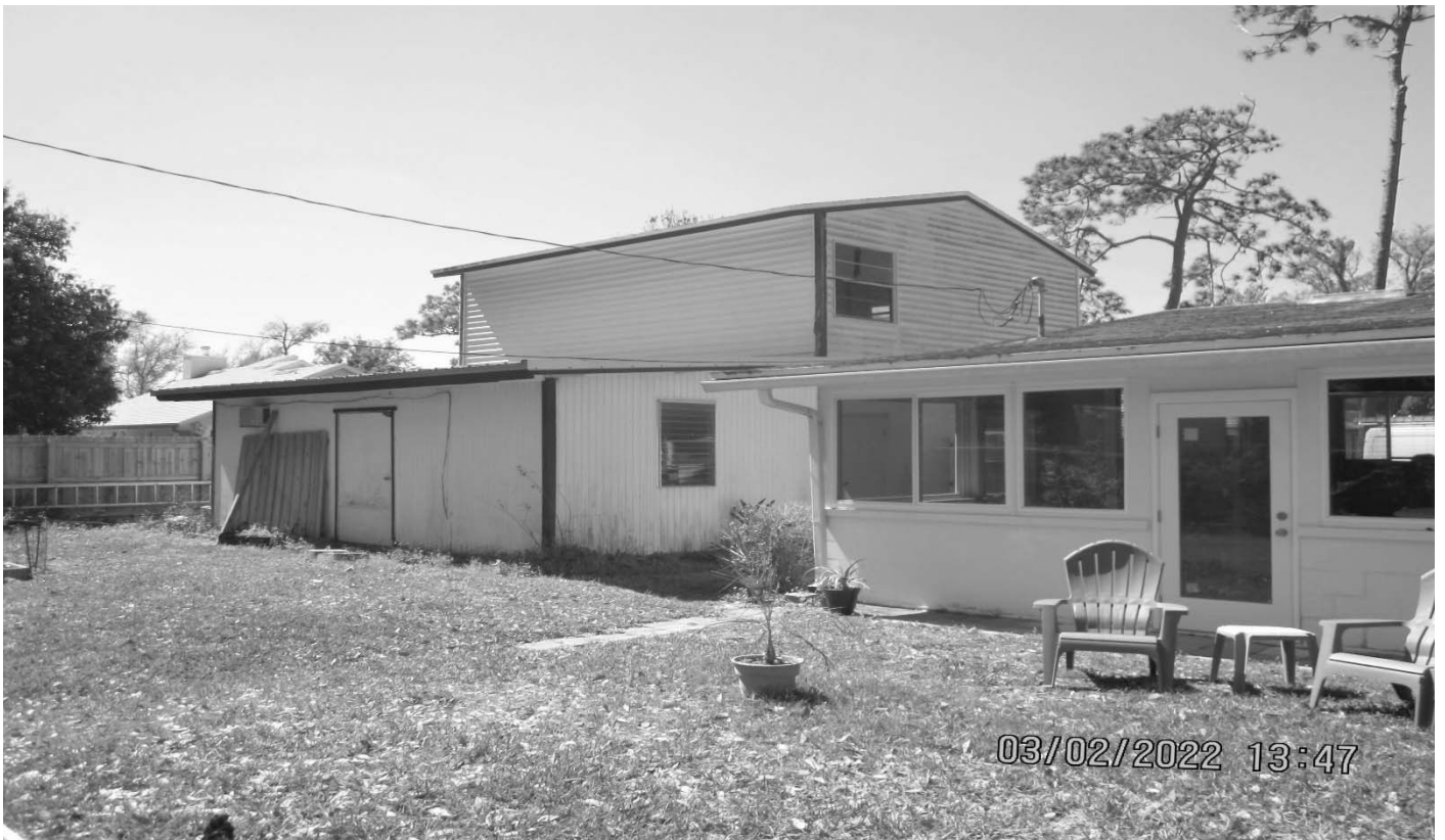
Rear yard, facing southwest towards rear of accessory structure (garage/ADU)
