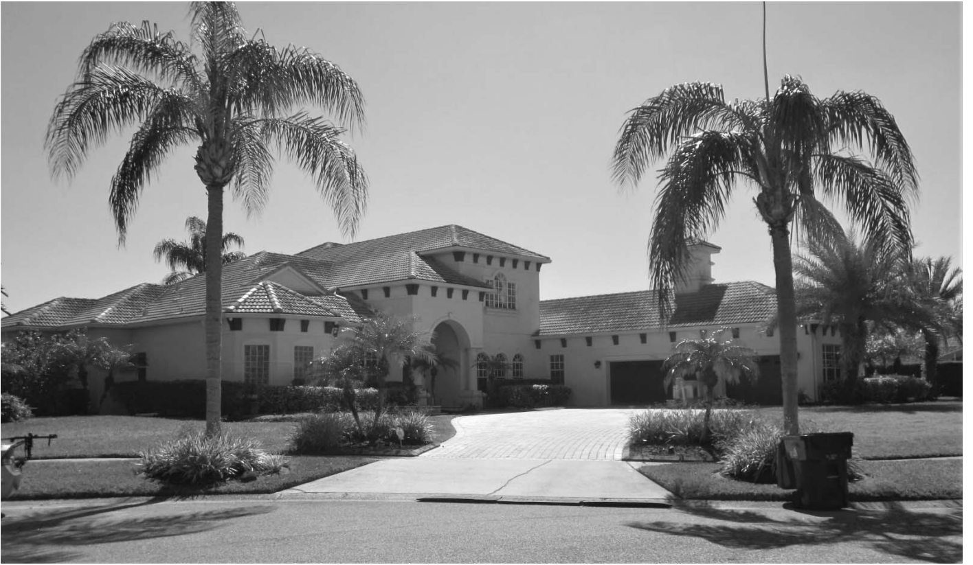
Facing south towards front of subject property
