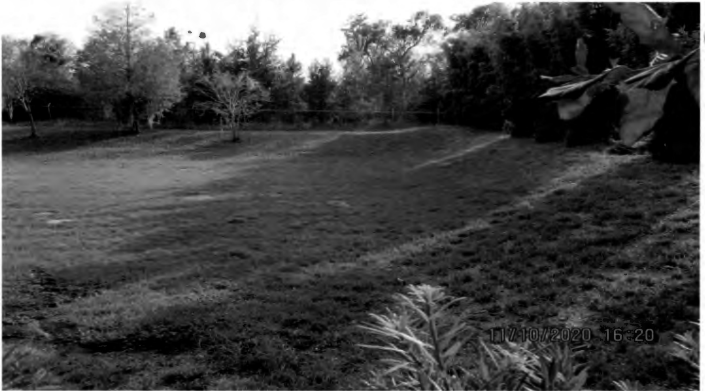
Retention pond looking south
