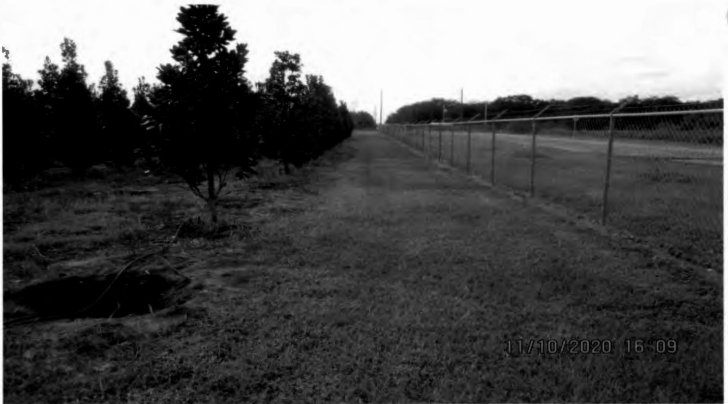
Site adjacent to Sandhill Rd. looking west
