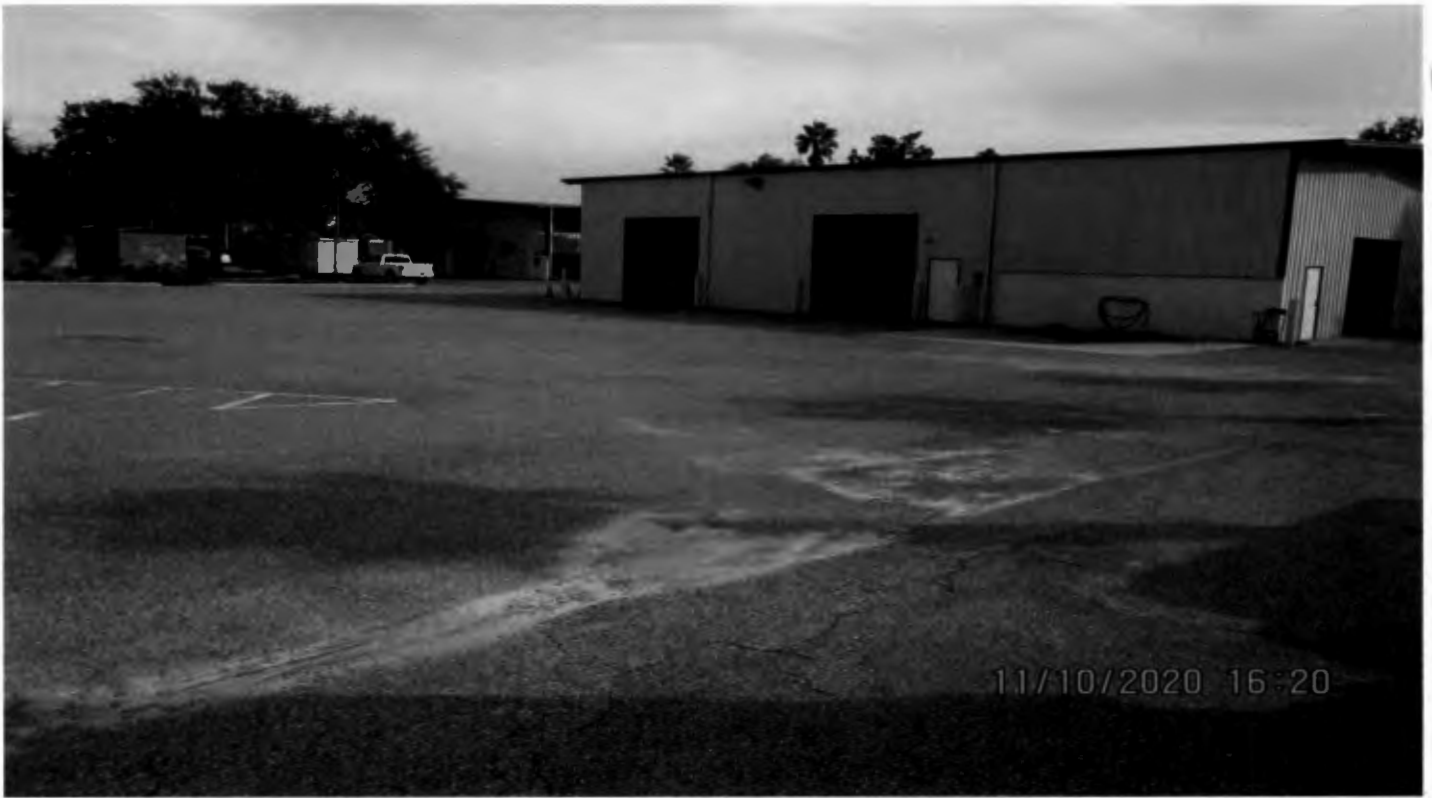
Building 4 looking south
