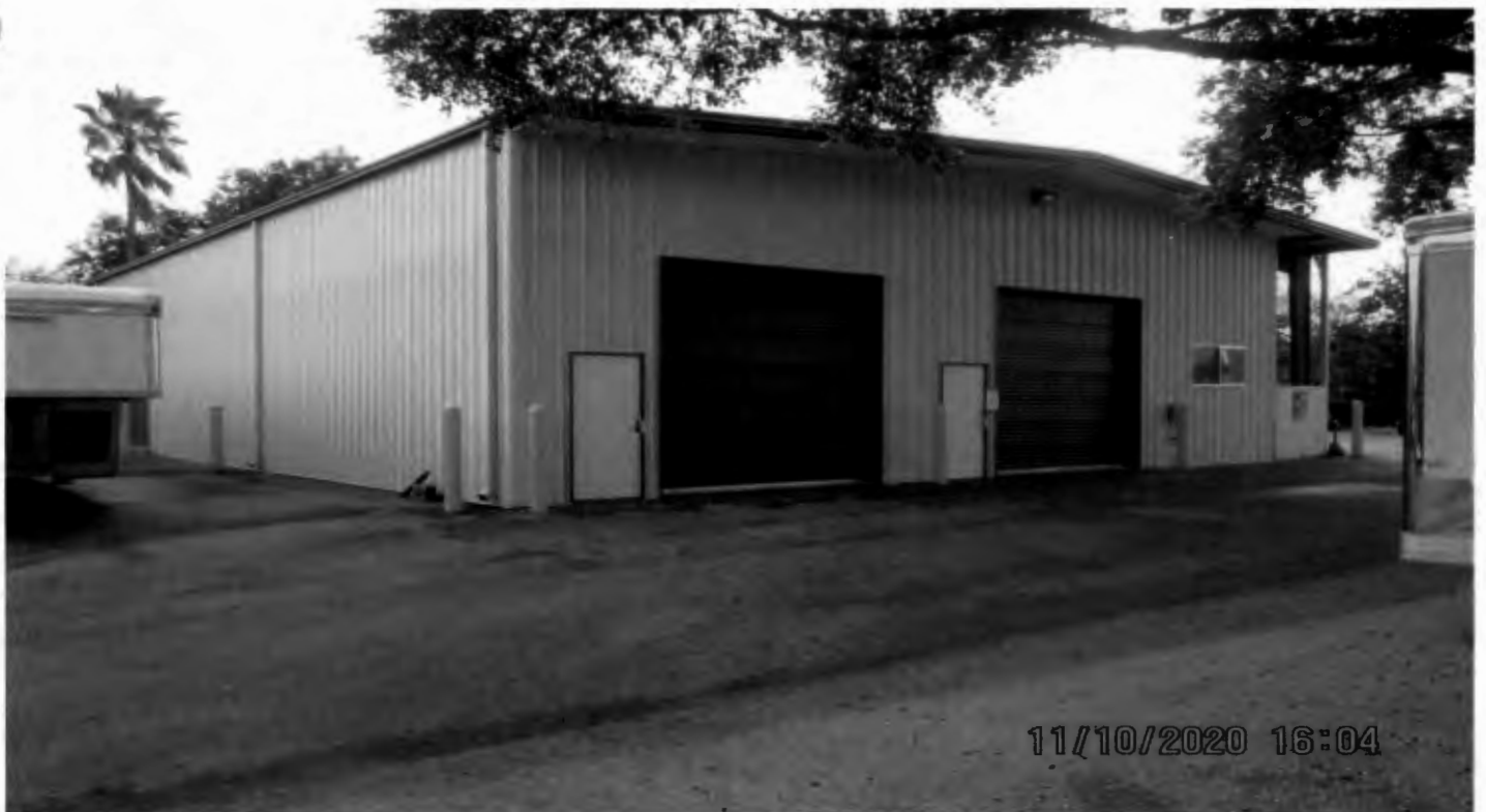
Building 3 looking southwest
