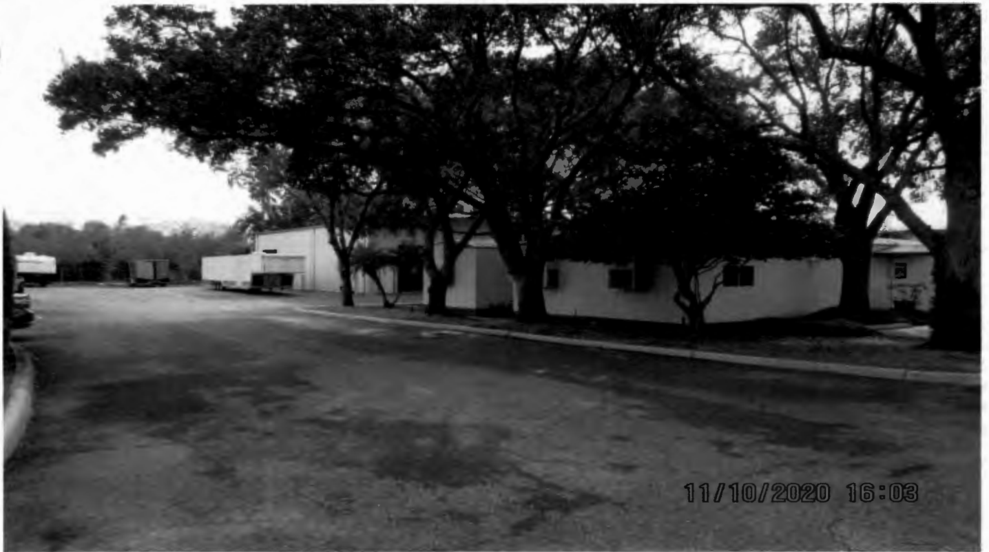
Buildings 1, 2, and 3 looking southwest
