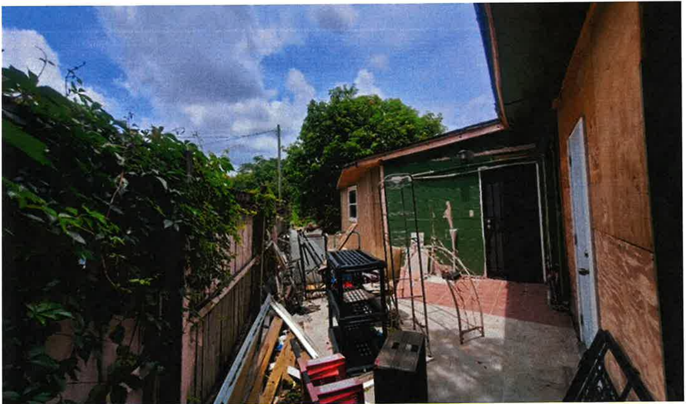
Facing north from rear yard, showing all 3 storage additions
