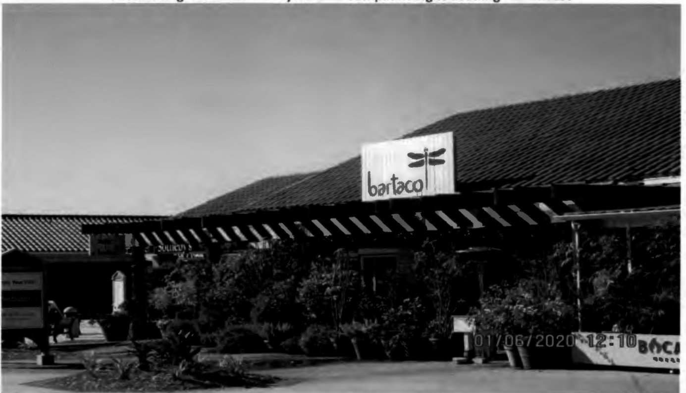
Sign Granted Variance in 2017 Looking Southwest
