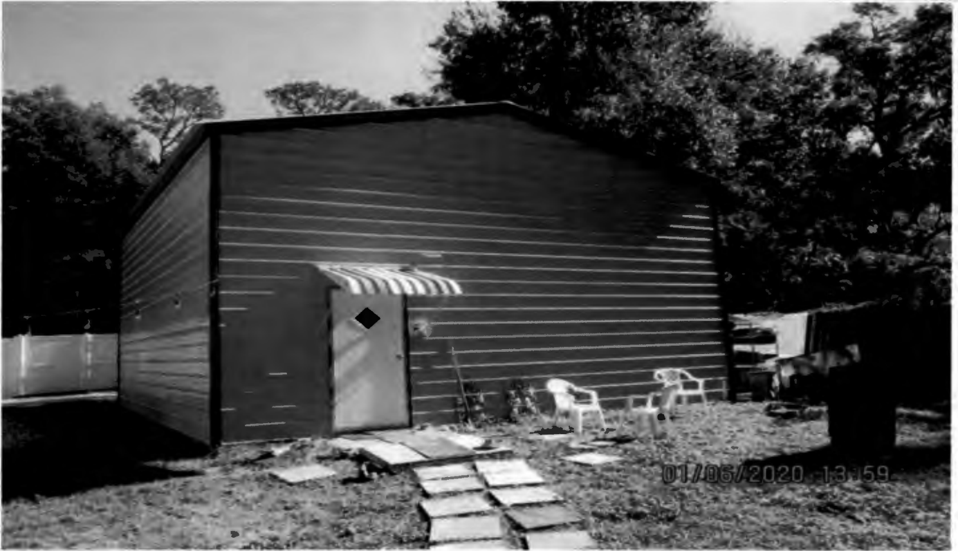
Rear of Garage Looking East
