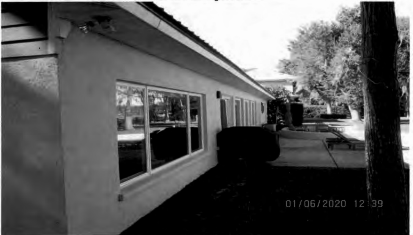
Rear of Residence Looking West
