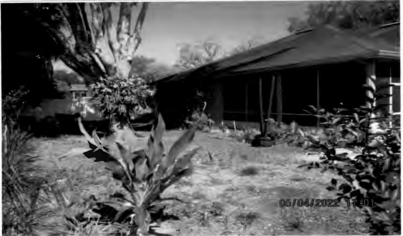
Rear yard, facing north towards proposed addition location
