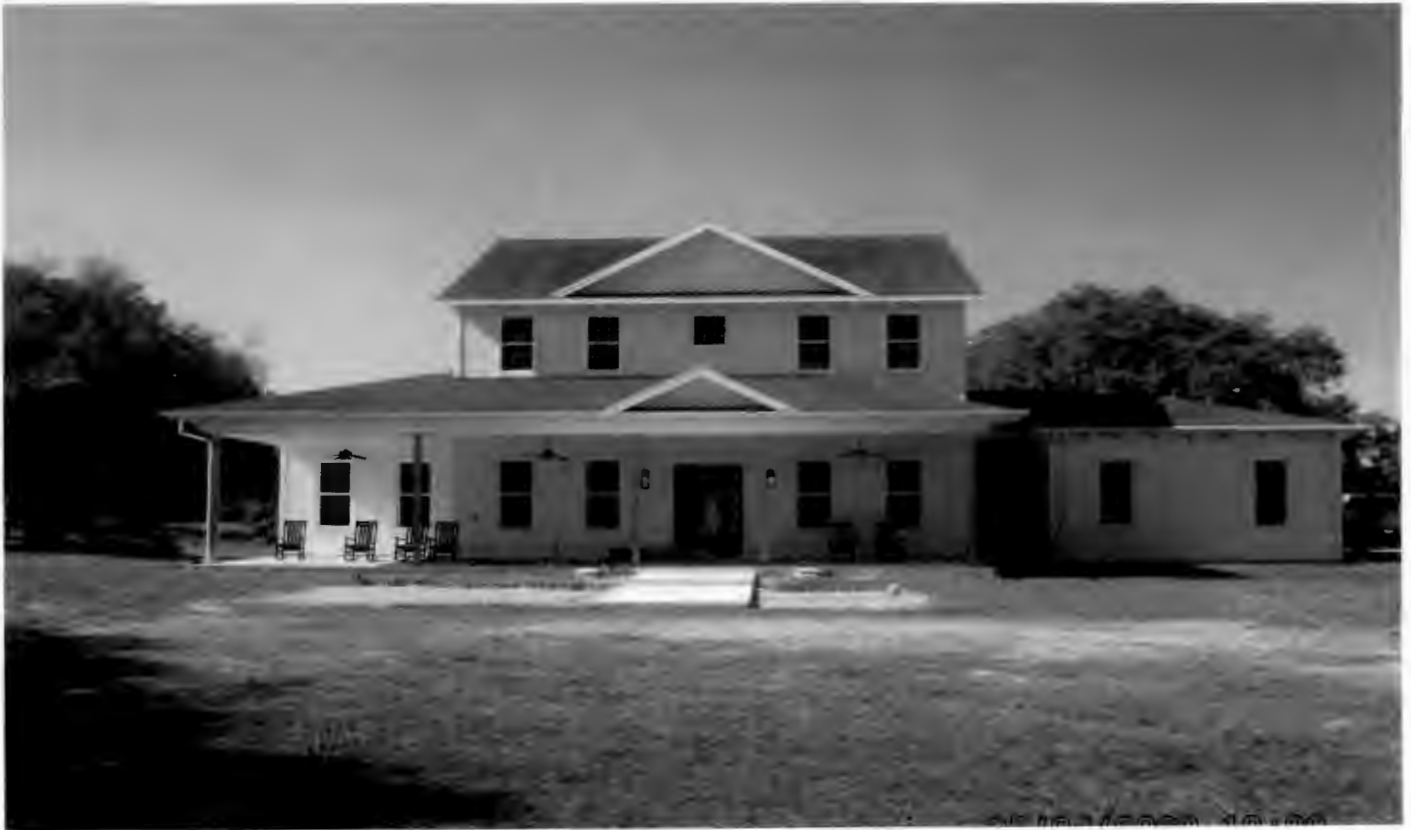
Facing south towards front of subject property
