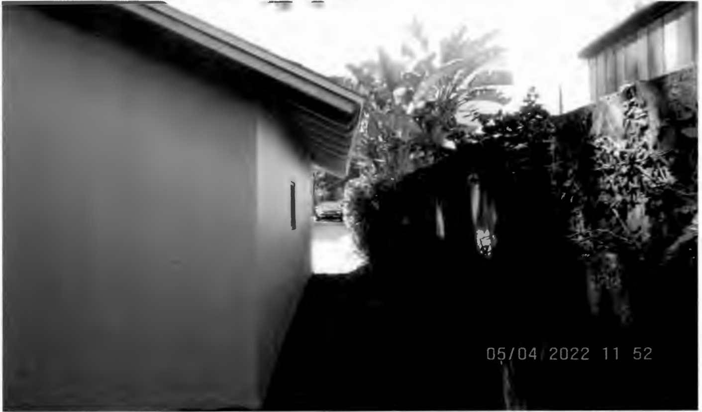
Rear yard, facing south towards side of proposed ADU
