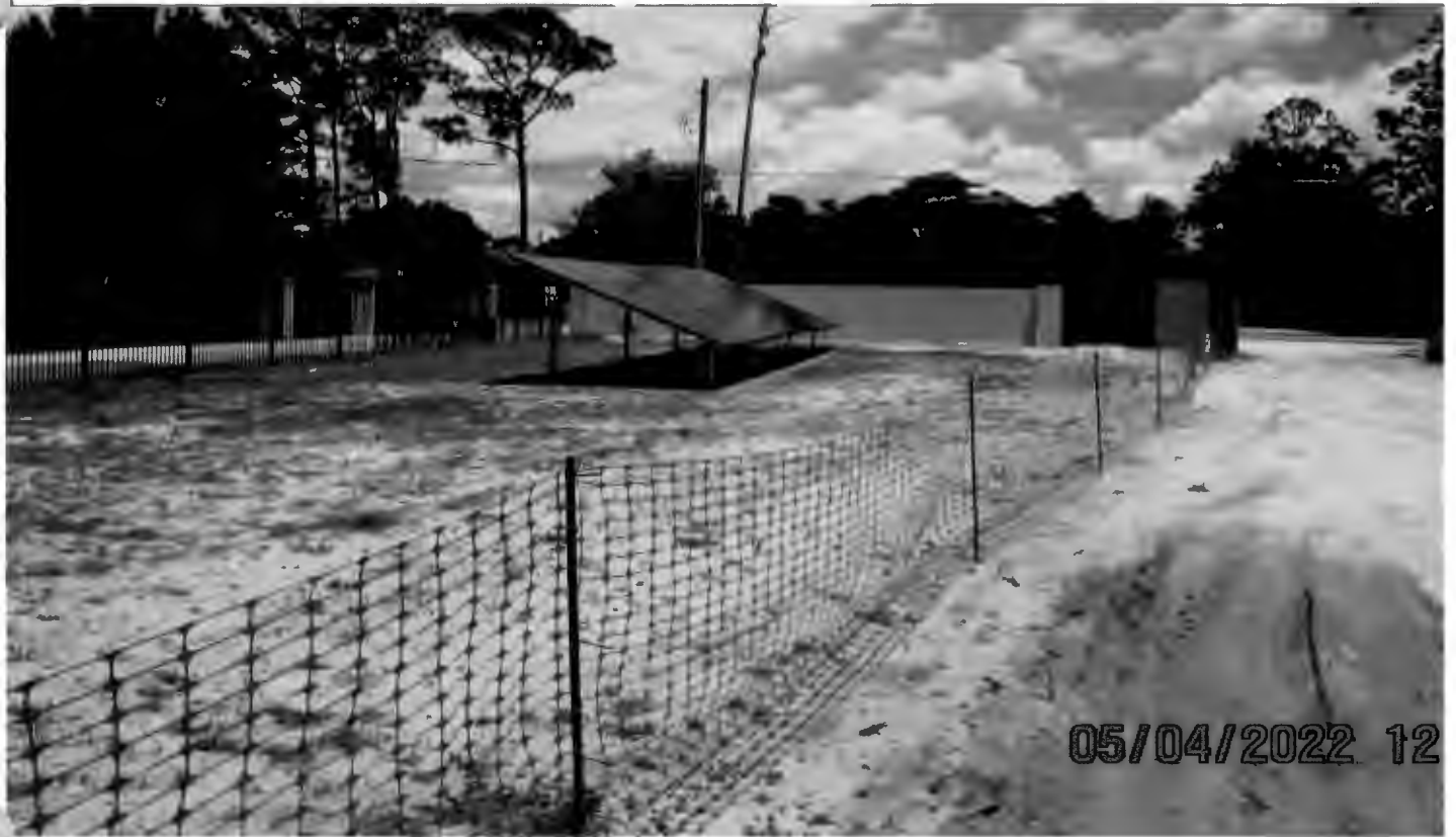
Solar panels facing east (opaque fence or wall to be installed)
