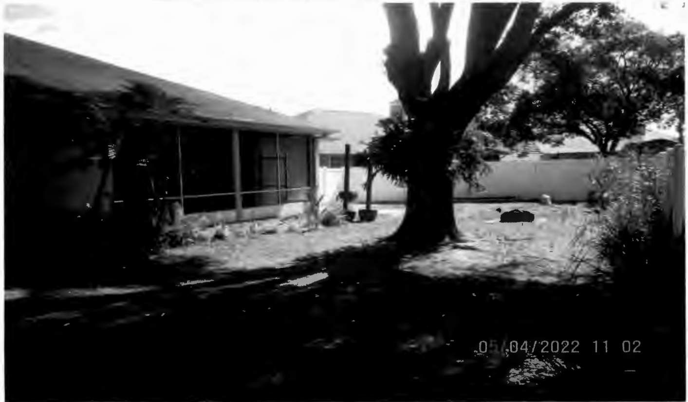
Rear yard, facing northeast towards rear of proposed addition location
