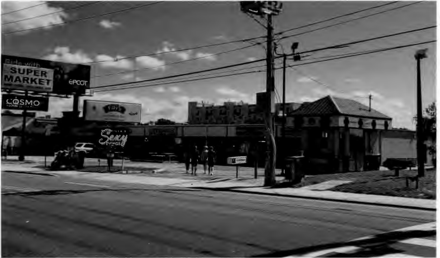
View of structure across International Drive, facing East
