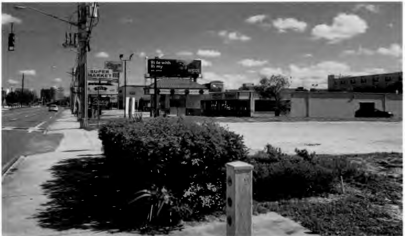
View of south side of structure, facing north on International Drive
