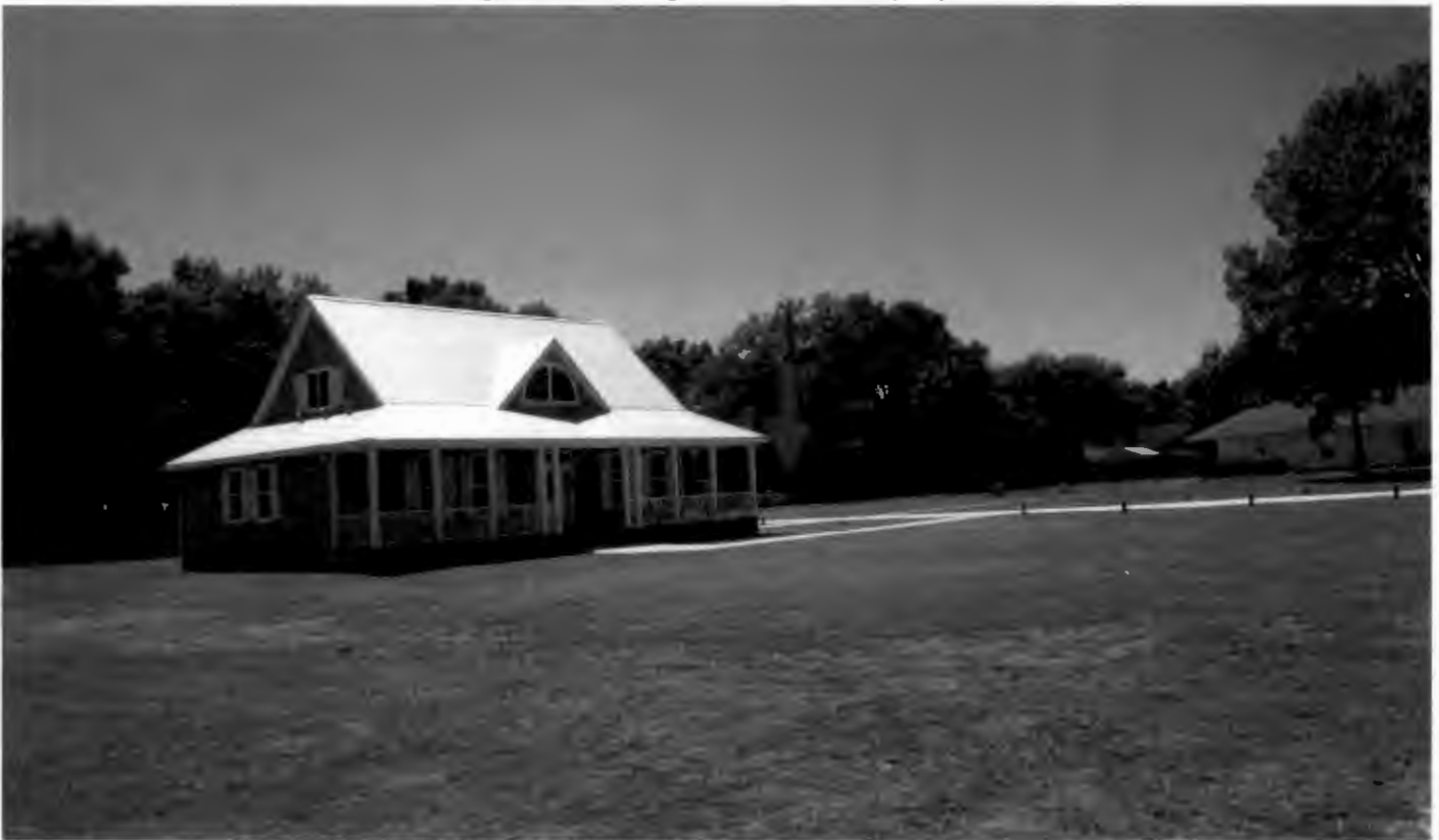
Facing southwest from north property line
