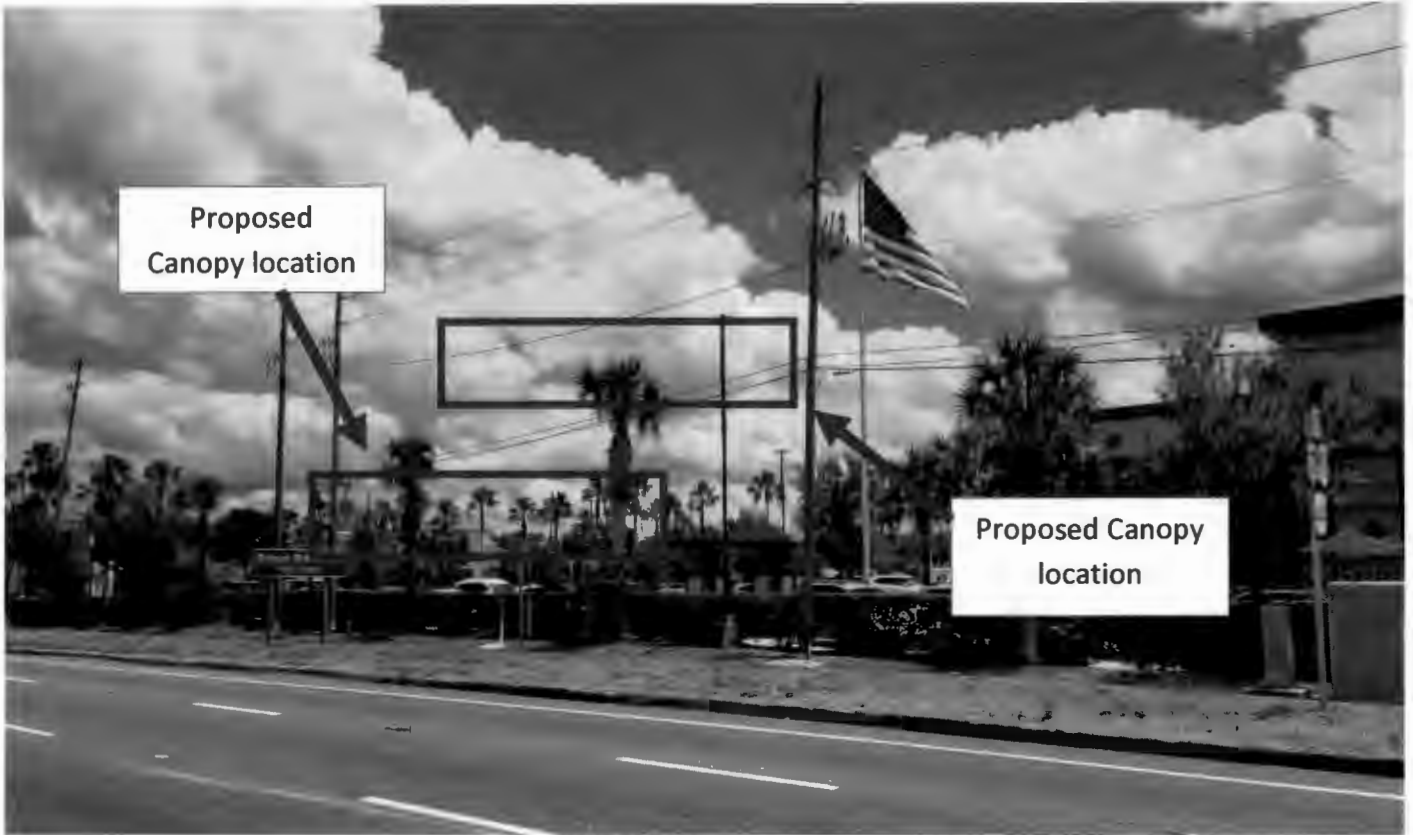
Facing southeast from W. Sand Lake Rd. towards proposed canopy location
