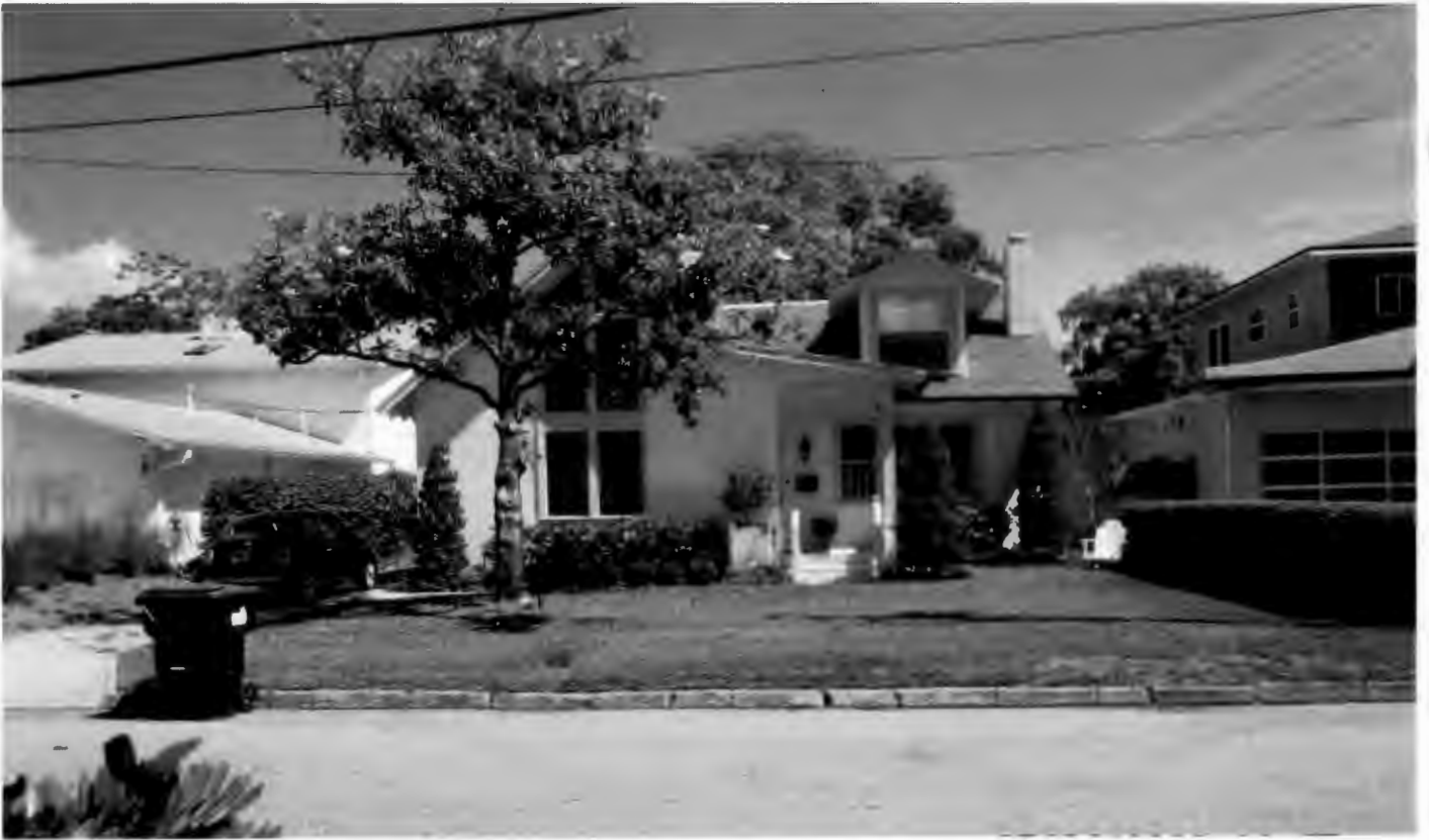
Facing north towards front of subject property
