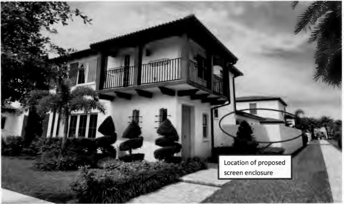
Facing southwest towards front/side of subject property
