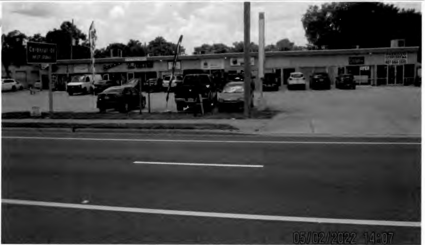
Building from N. Goldenrod Rd. facing west
