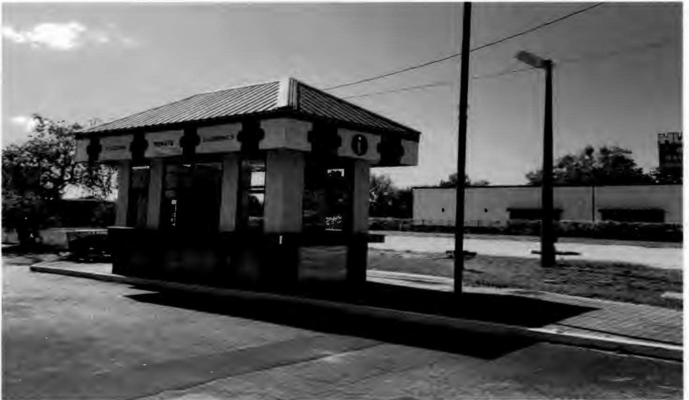
North side of structure, facing South from subject property
