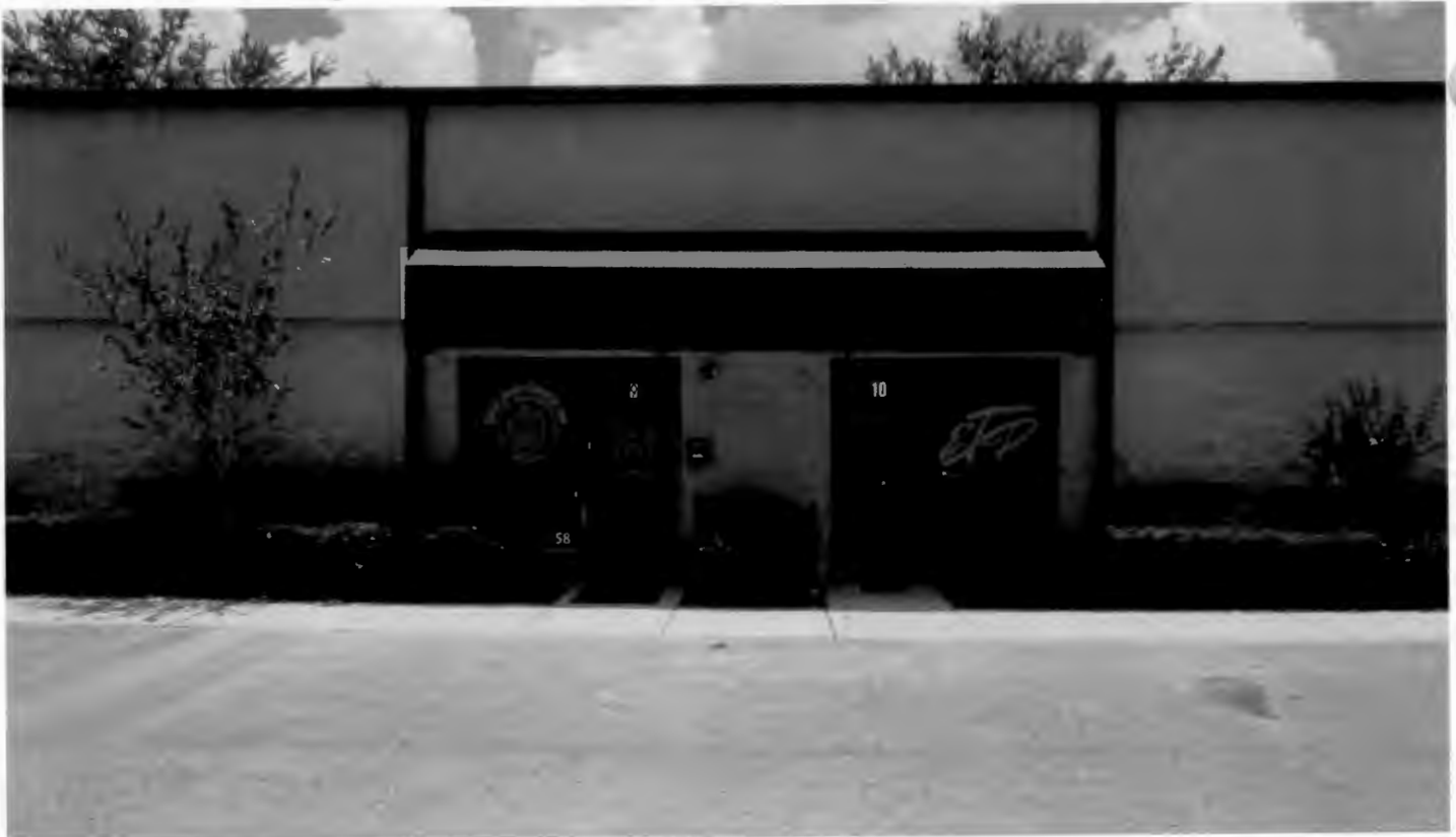
El Tabernaculo Pentecostal Church 687 ft. separation
