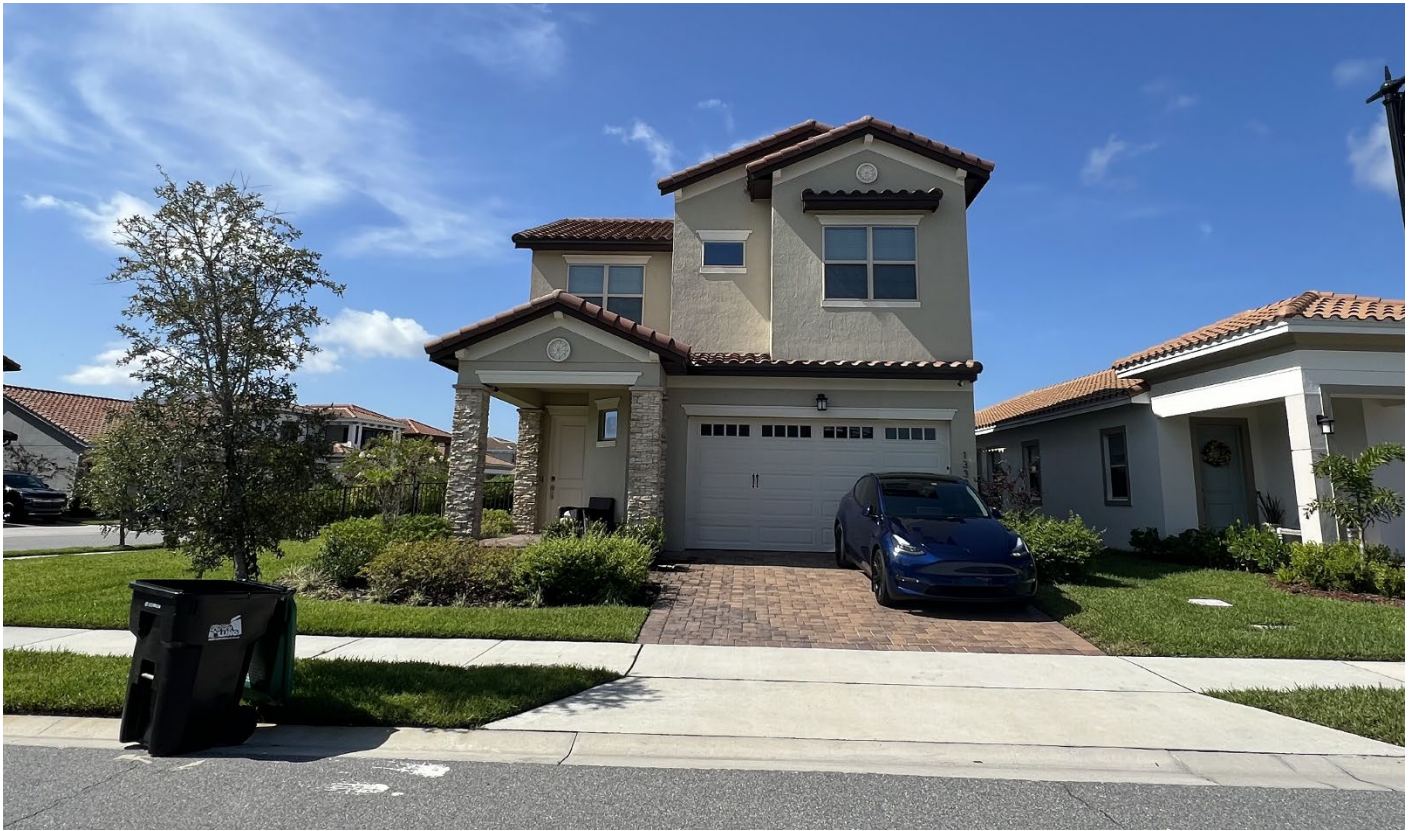
Facing south towards front of subject property
