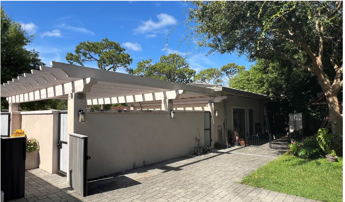
Rear yard, facing south
