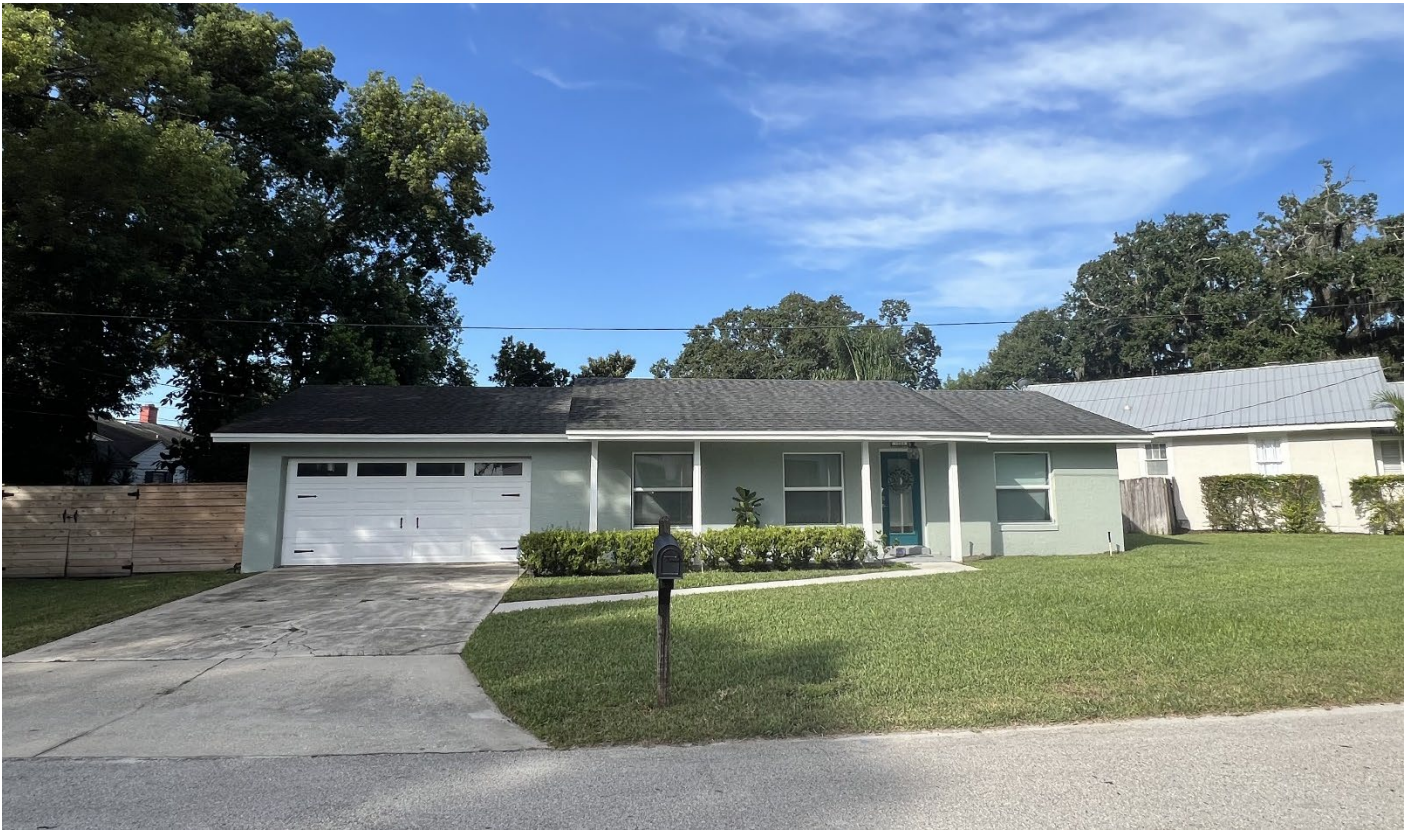
Hour Glass Dr., facing southwest towards front of subject property
