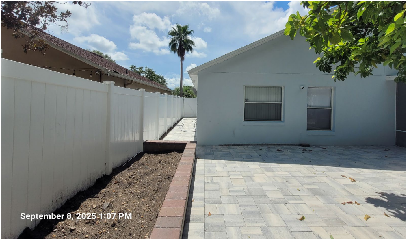
Rear yard facing south, towards pavers and rear of the residence
