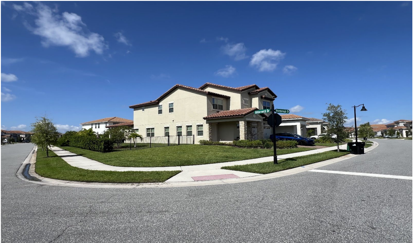
Intersection, facing southwest towards the side of the subject property
