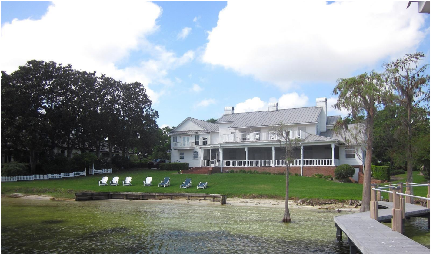
Boat dock, facing west towards proposed pool/deck location to be attached at rear of existing residence
