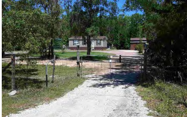
Structure elevated above grade with crawl space
