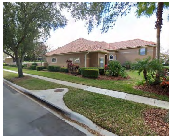
Drainage feature along road
