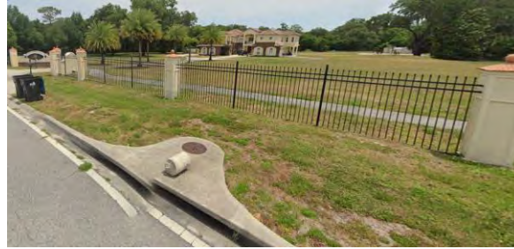
Storm drain along roadway
