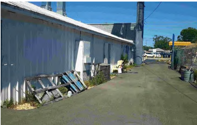
HVAC unit not elevated
