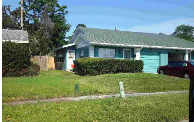
Drainage swale between lots
