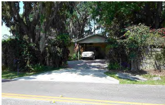
Drainage feature along road and under driveway
