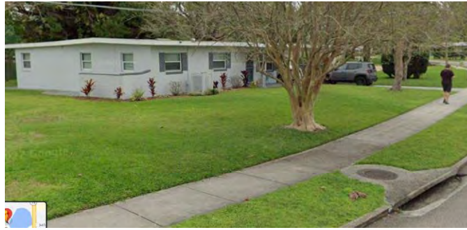
Storm drain along roadway
