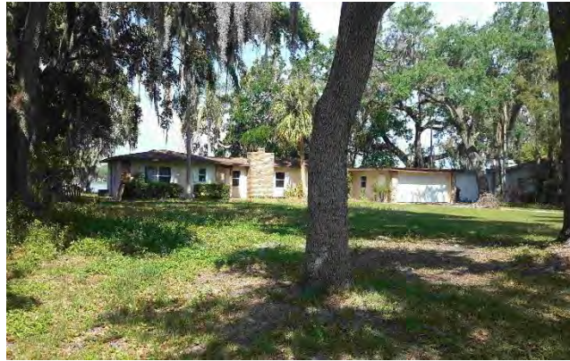
HVAC unit not elevated
