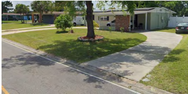
Curb for drainage
