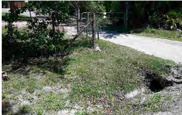
Drainage ditch along roadway
