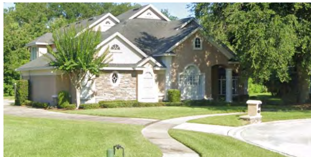
Newer home with gutters
