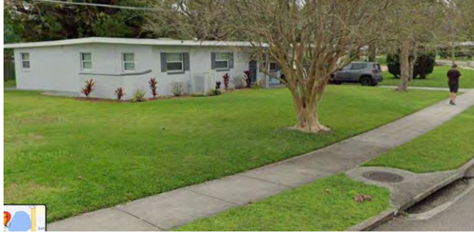
Storm drain along roadway
