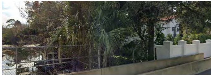
House backs up to creek
