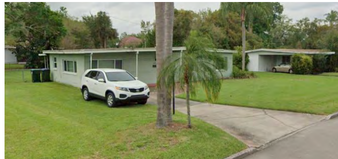
Driveway slightly below grade
