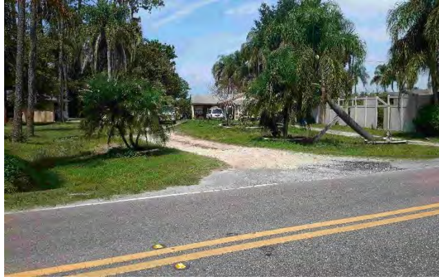
Drainage swale in front yard
