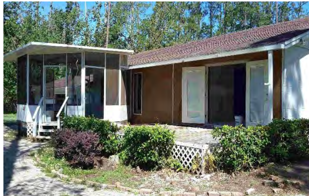
Elevated deck and slab-on-grade foundation
