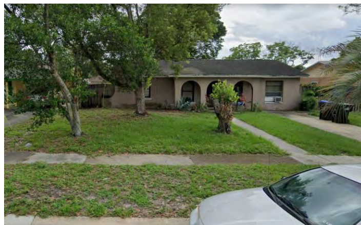
Masonry home without gutters
