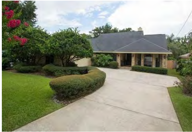
House below grade
