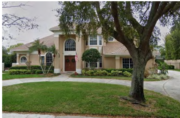
Two story home with adequate gutters
