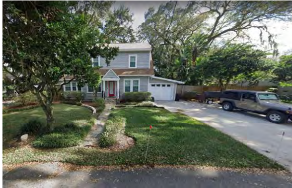
Elevated home with vents
