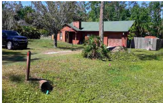
Drainage feature in front of property near roadway
