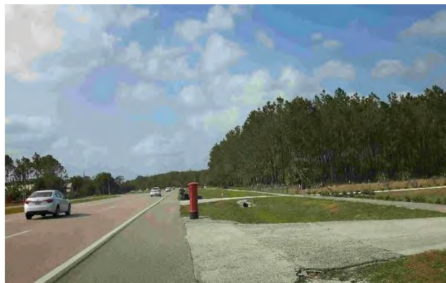
Drainage ditch and culverts along roadway and under driveways
