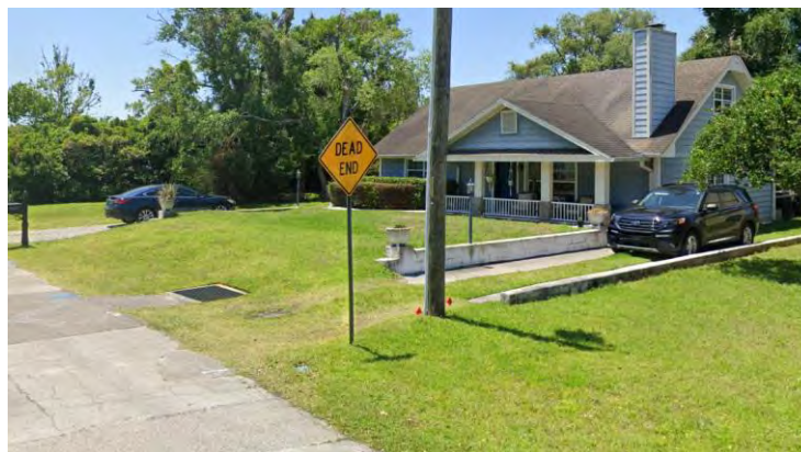
Grated drain in front lawn
