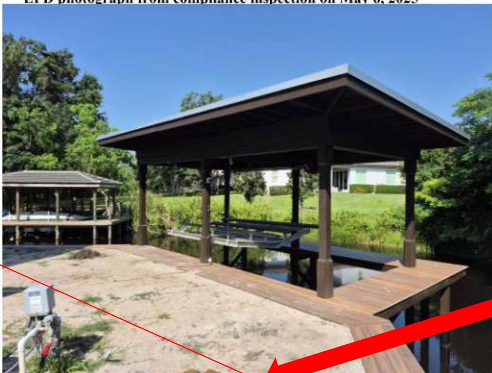
EPD photograph from compliance inspection on May 6, 2025
