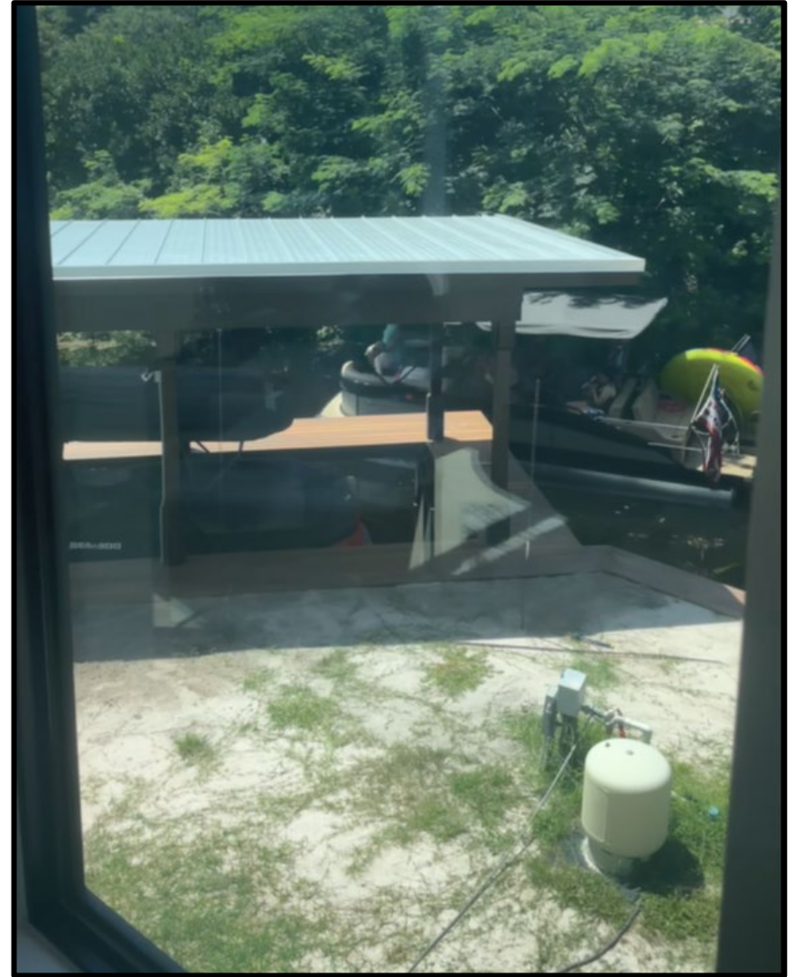
January 2026 - Photo of boat dock and seawall location as constructed.
