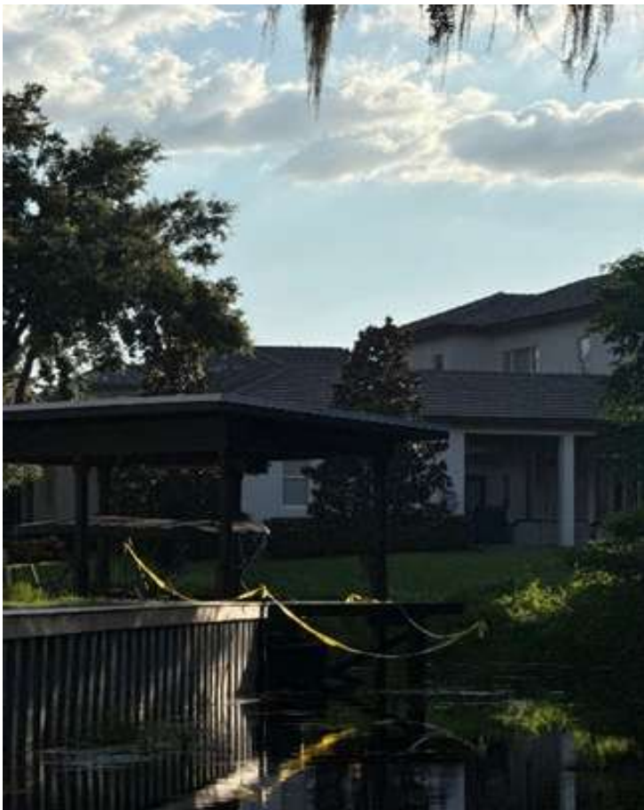
At dusk picture shows how difficult it is to see the corner of the dock protruding out into the canal.
