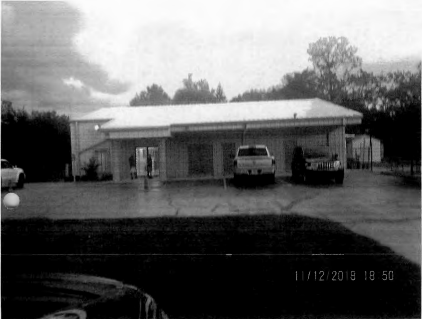
Existing Sanctuary Looking East
