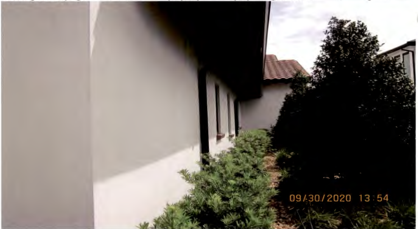
Potentially compliant location for zoning setbacks but unavailable due to window location, looking northeast
