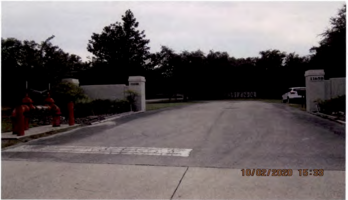
Decorative wall, viewed from front of property, looking south
