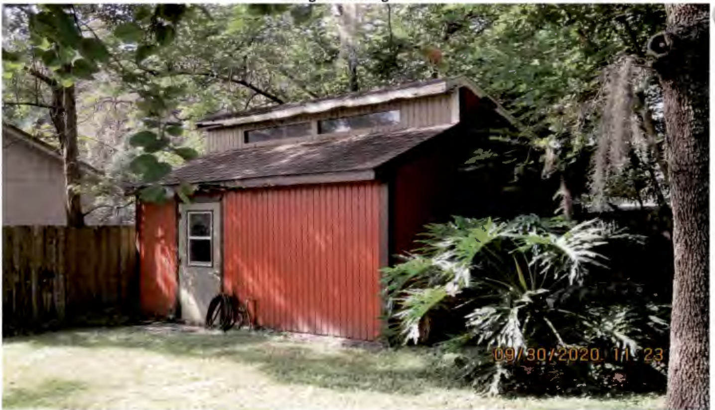
Shed looking southwest
