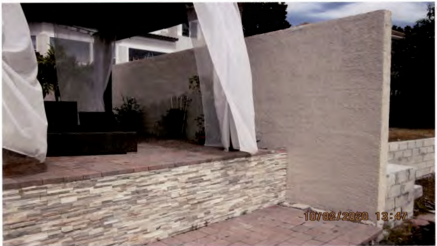
Wall within NHWE setback, looking north
