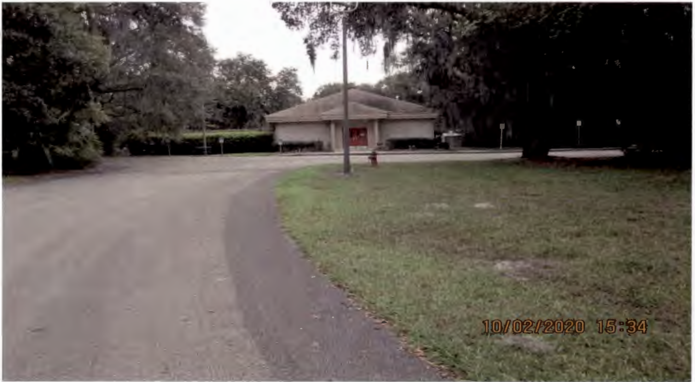
Front of sanctuary building, looking south
