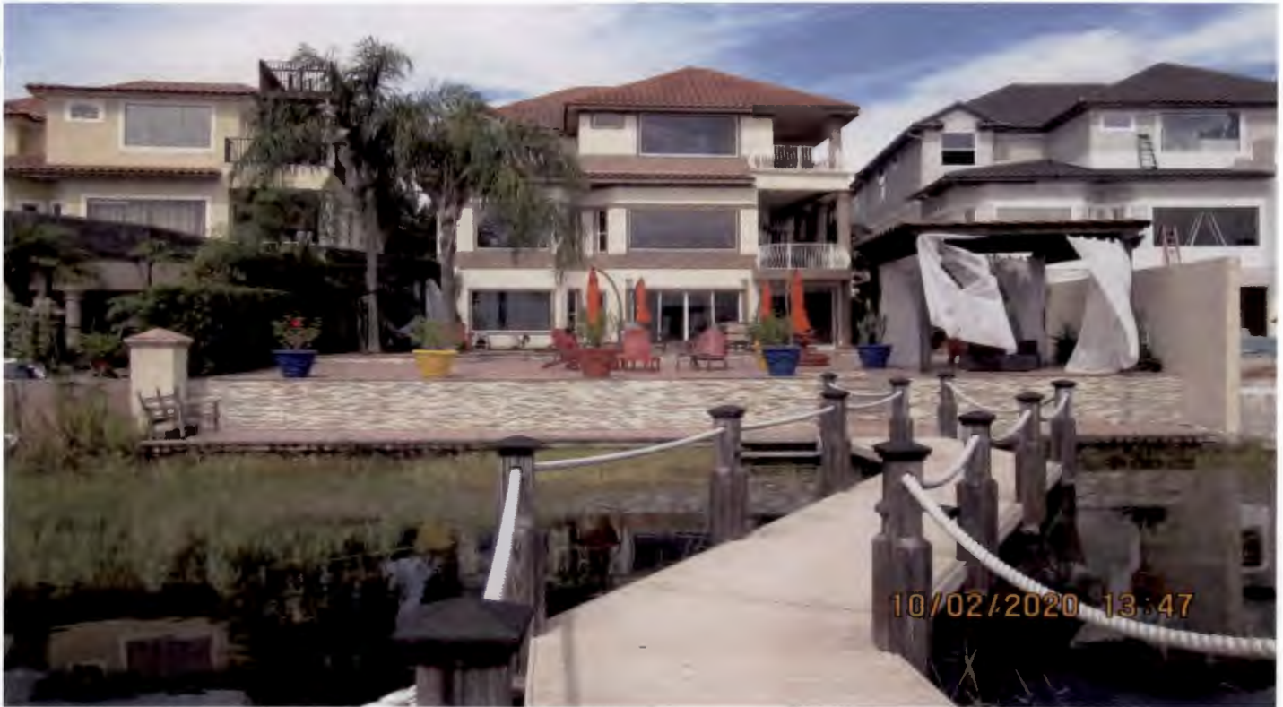
Rear, looking north
