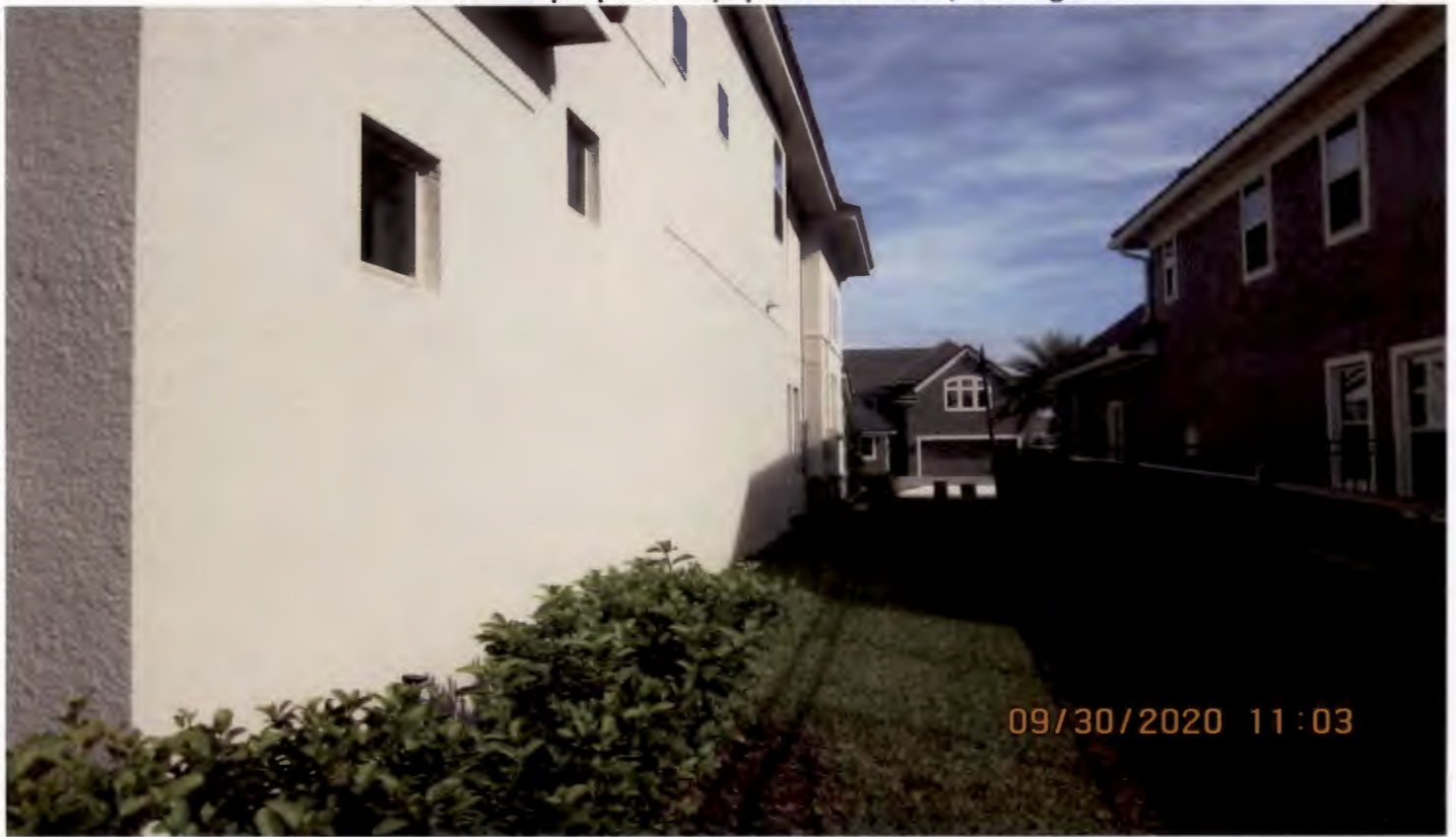
East side of house proposed equipment location, looking north
