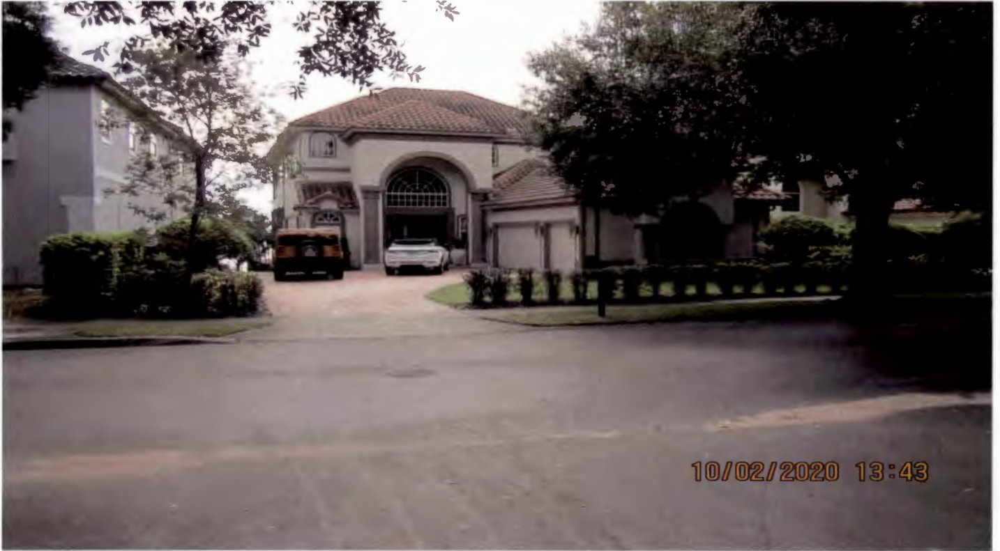
Front from Firenze Blvd., looking south
