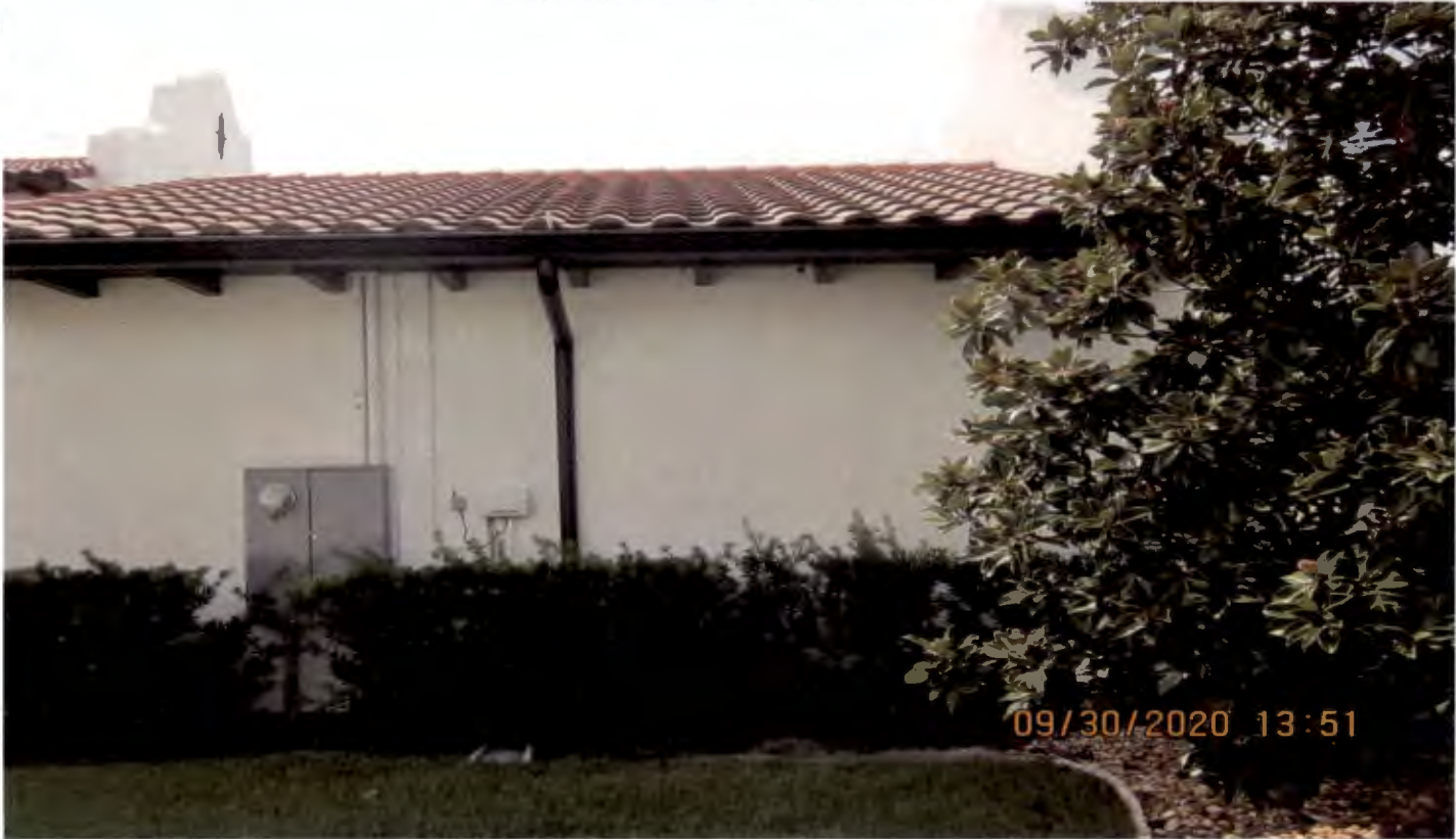
Approximate location for proposed generator
