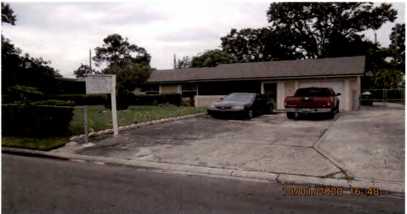
Nearest Community Residential Home at 4213 Chantelle Rd. facing north
