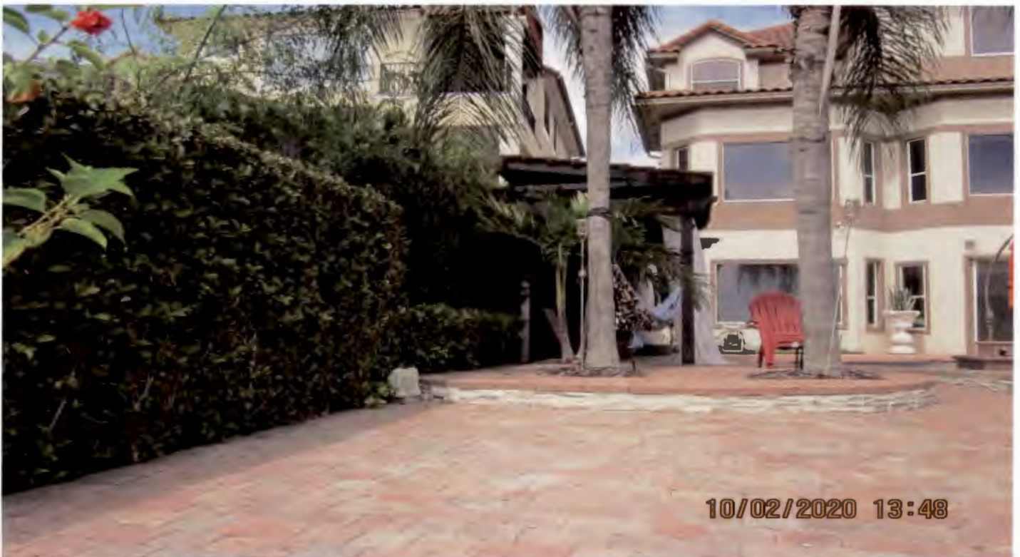
Pergola with 6 inch, and pool deck with zero west side setback, looking north
