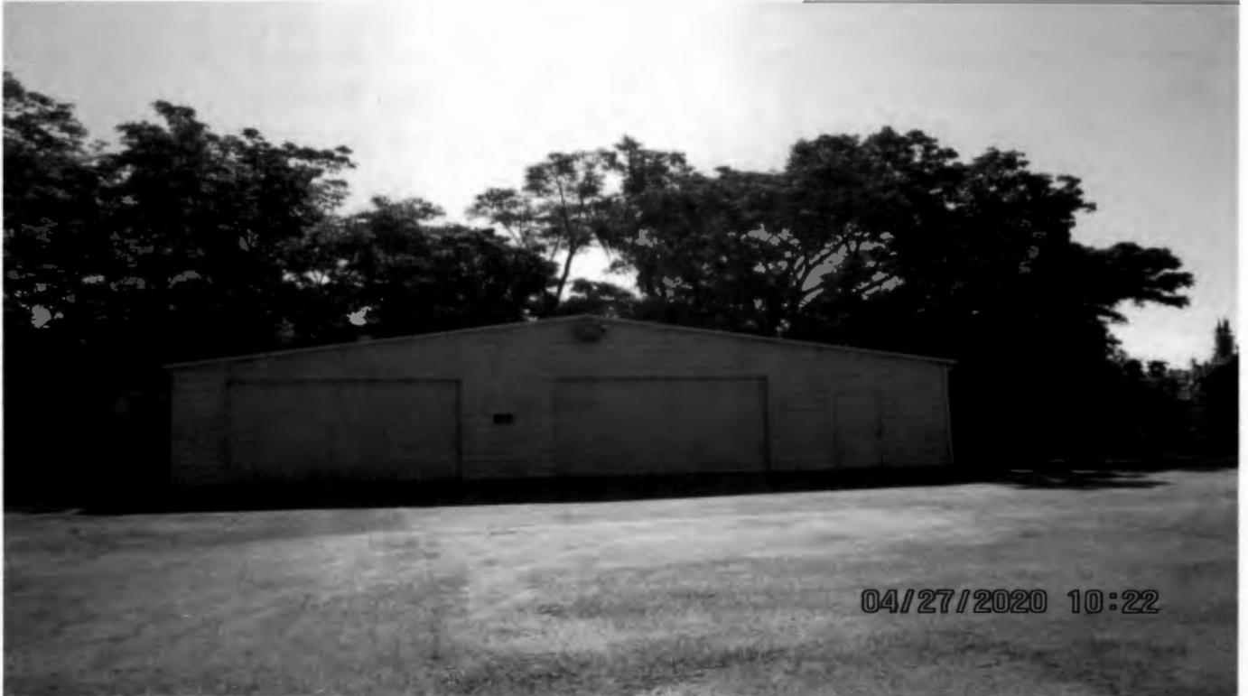
Structure in northeast corner of site looking east
