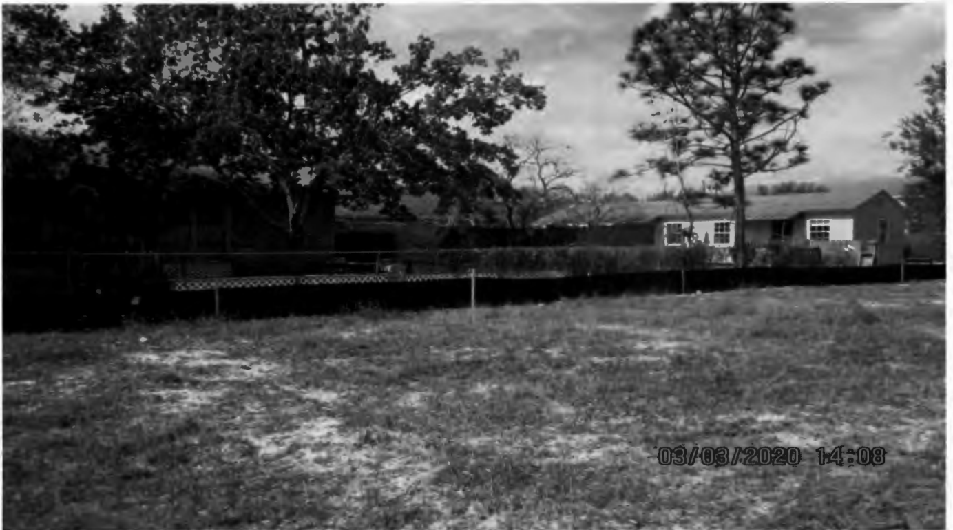
1069 sq. ft. bldg. to be removed. Location of new bldg. Viewed from rear
