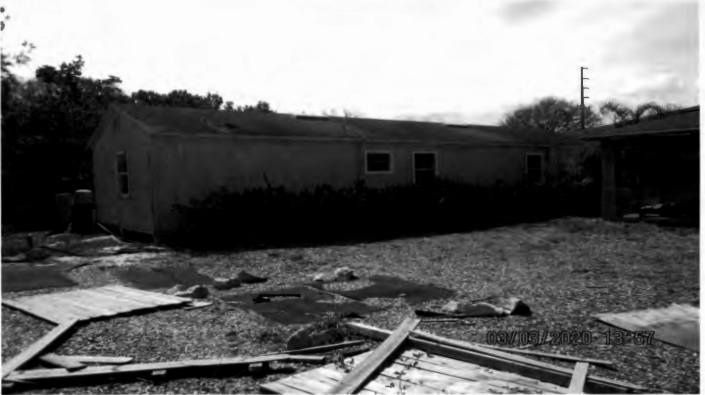
1069 sq. ft. bldg. to be removed. Location of new bldg.
