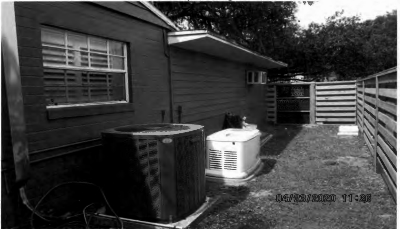
A/C pad and preferred generator location looking west
