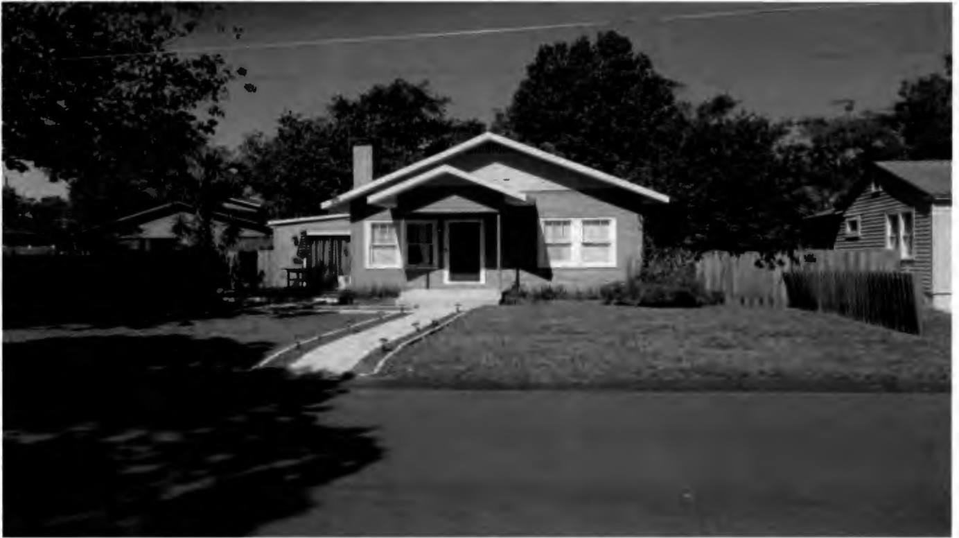
View of subject site from Newberry St.
