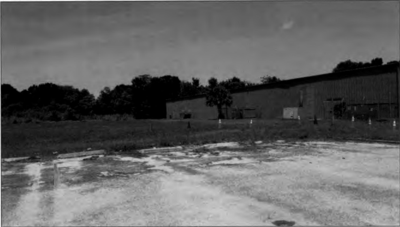
View facing west from existing parking area
