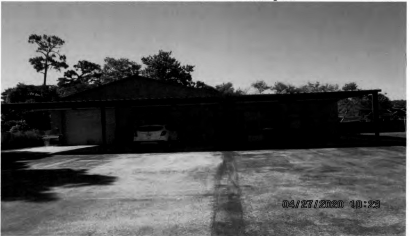
Structure in southeast corner of site looking south
