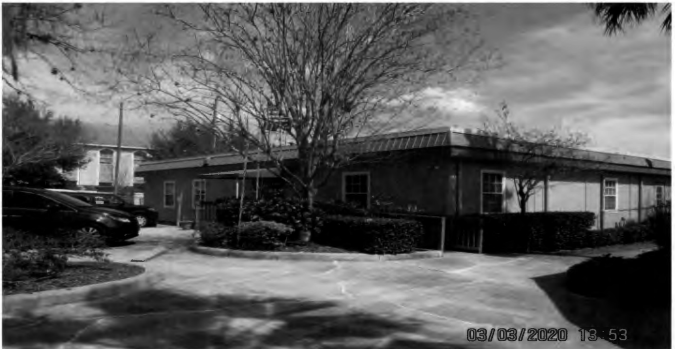
4528 sq. ft. bldg. to be removed
