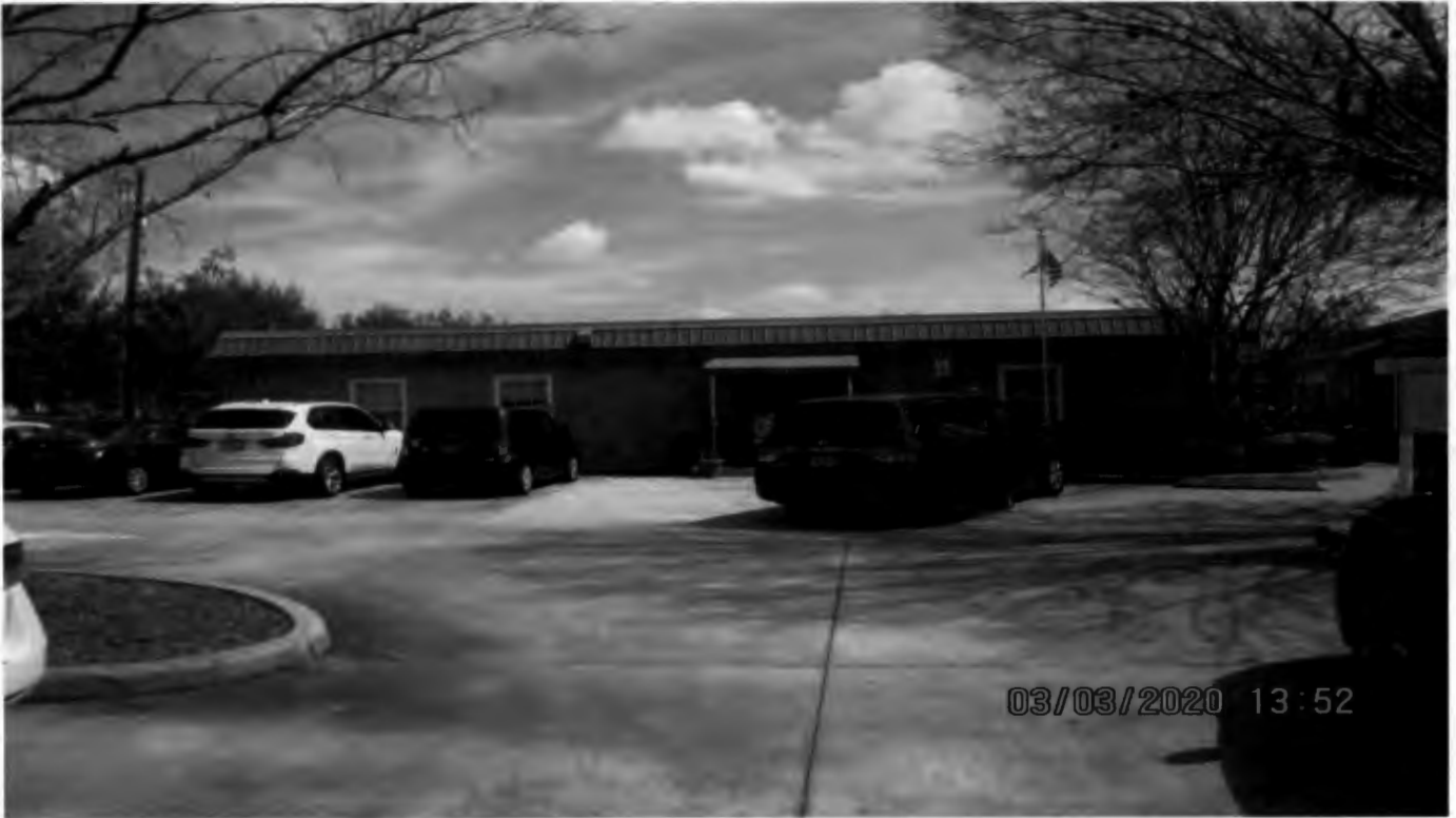
4528 sq. ft. bldg. to be removed
