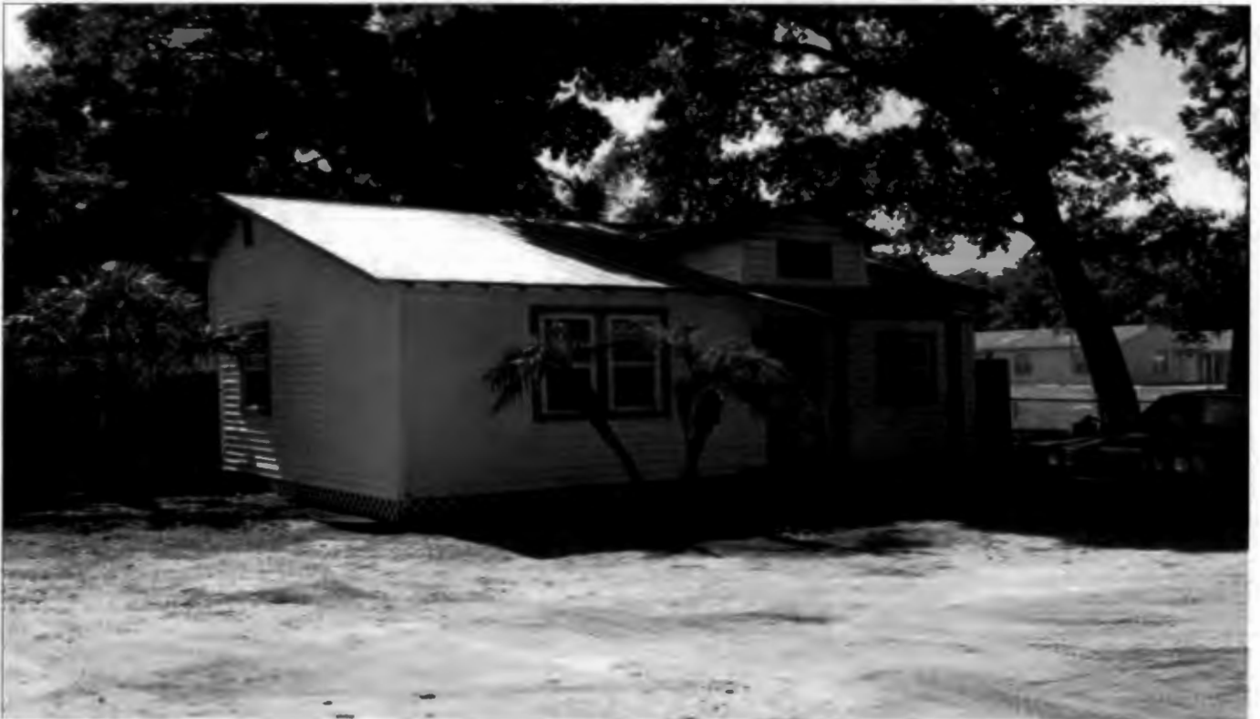
Subject property before new porch looking northwest
