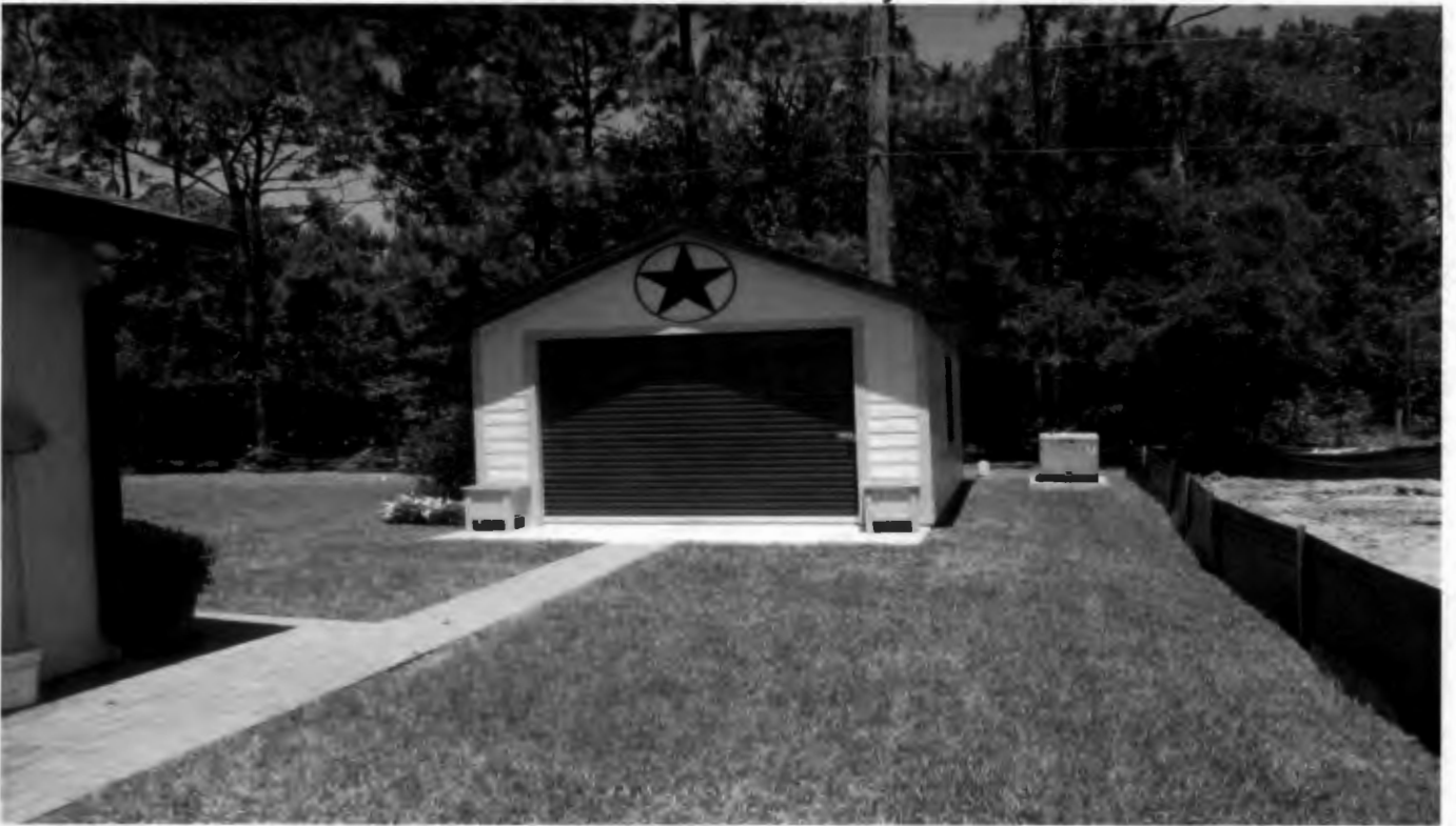
Shed from front
