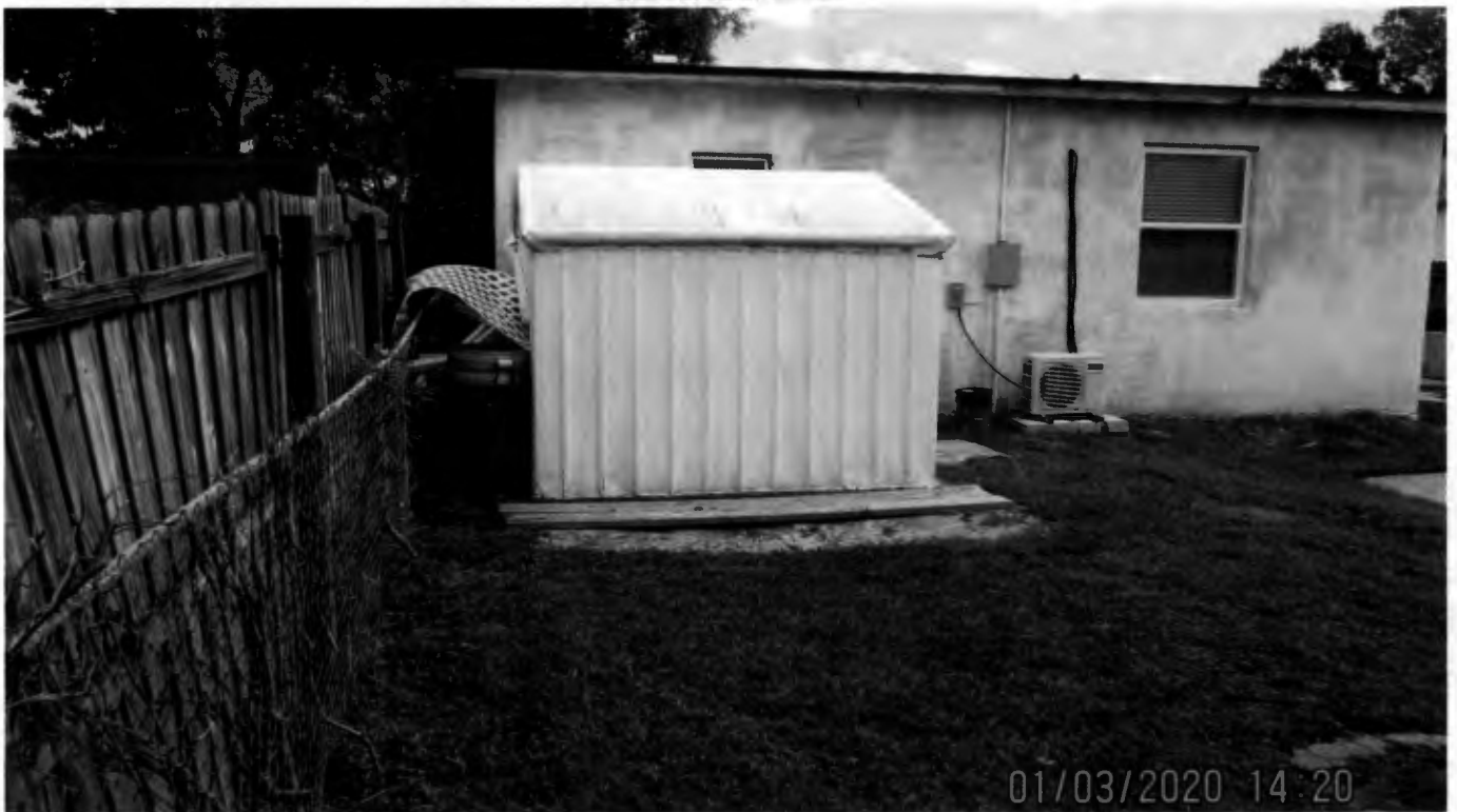
North rear setback. Existing metal shed to be removed.
