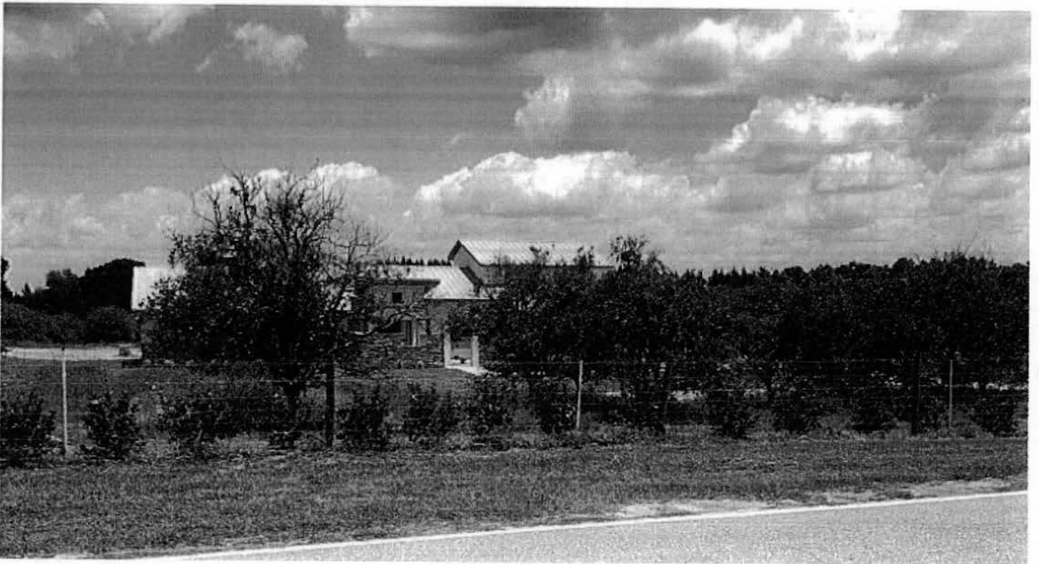
Single-family home to the north
