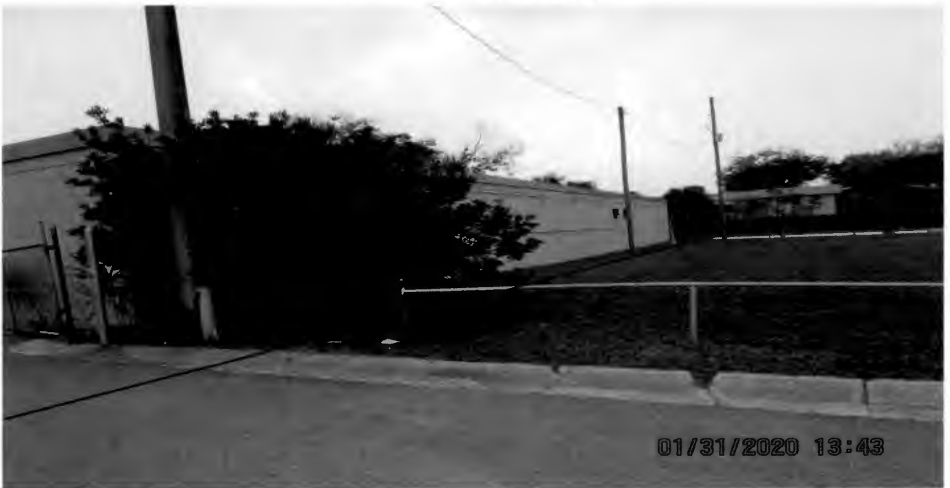
Variance #1; Bldg. G Proposed 2.92 ft. Side Setback In Lieu of 5 ft. Resulting From Creation of Proposed Lot 2 Proposed Property Line in Red
