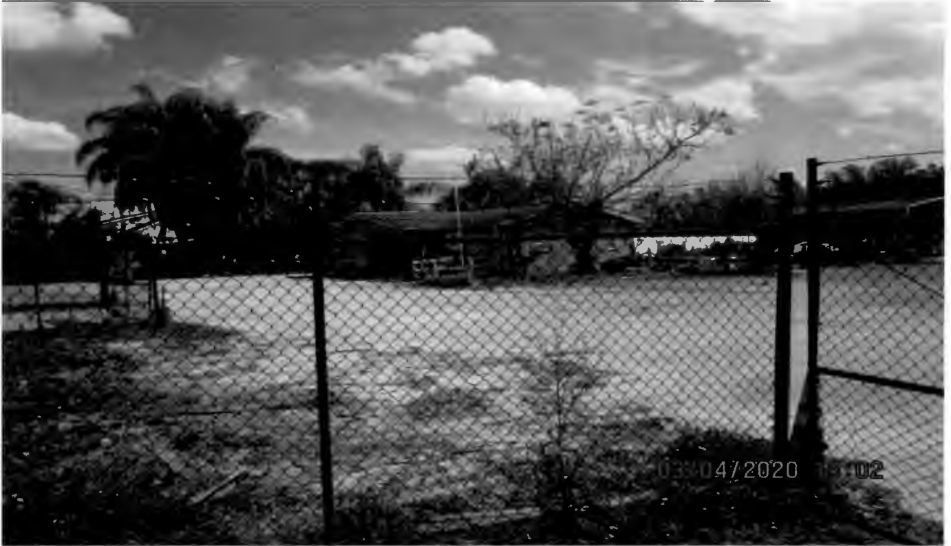
Existing office building for nursery, looking southeast
