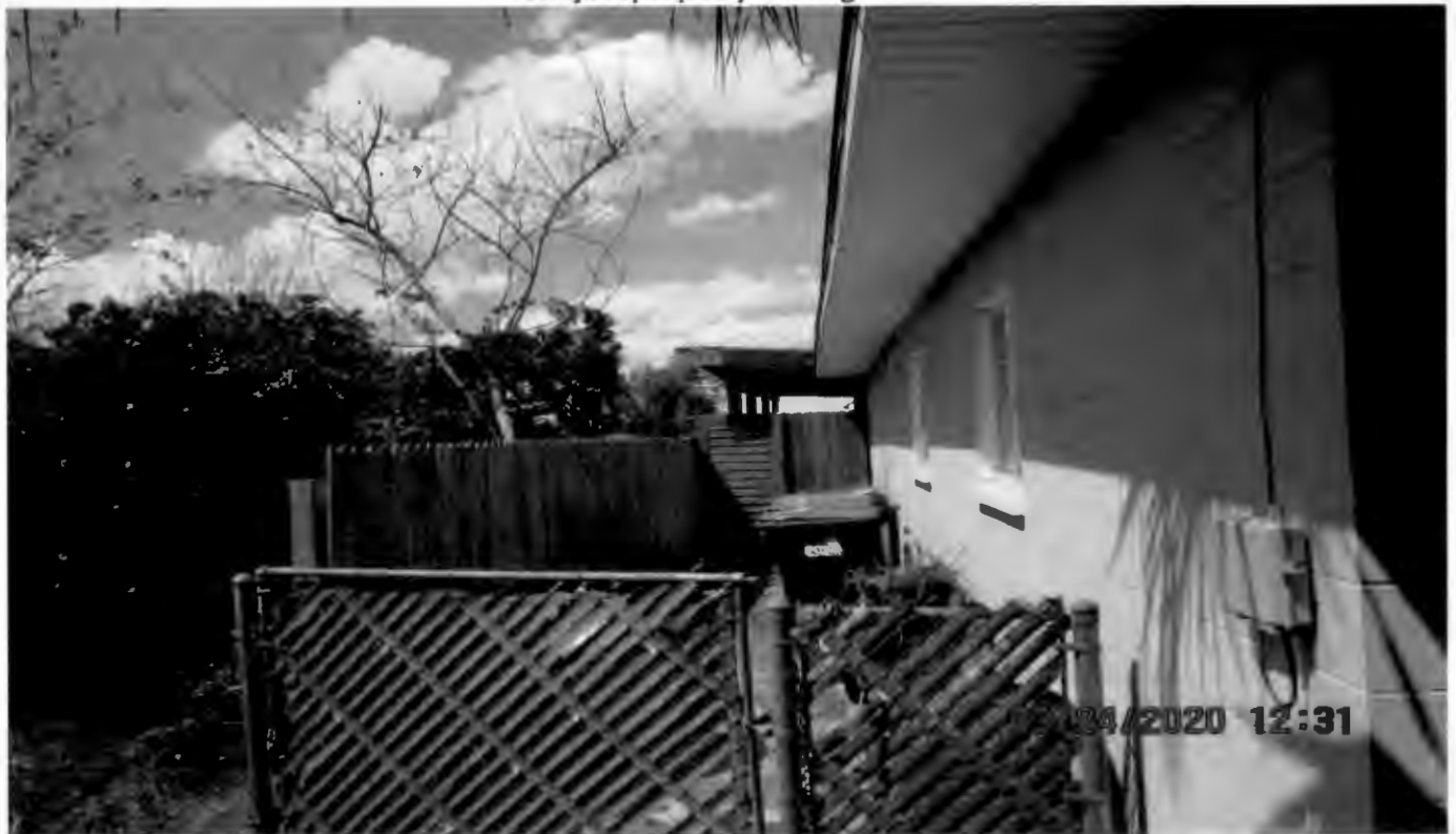
Roof of attached porch looking west
