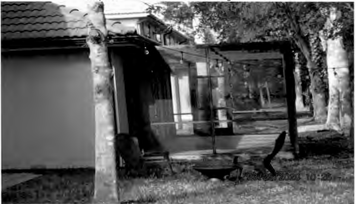
Existing screen enclosure on end unit of same building looking east
