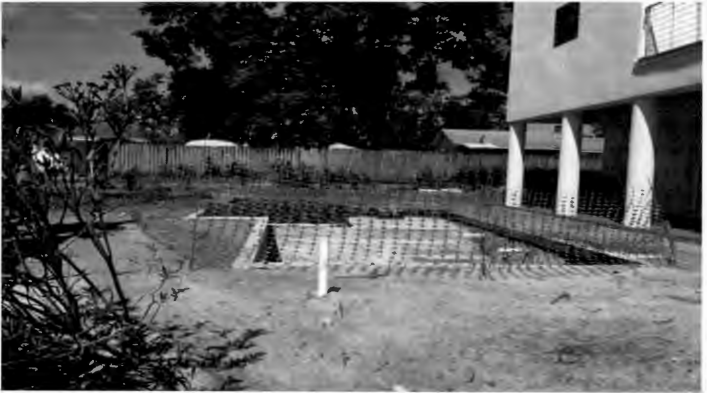
Subject pool currently under construction
