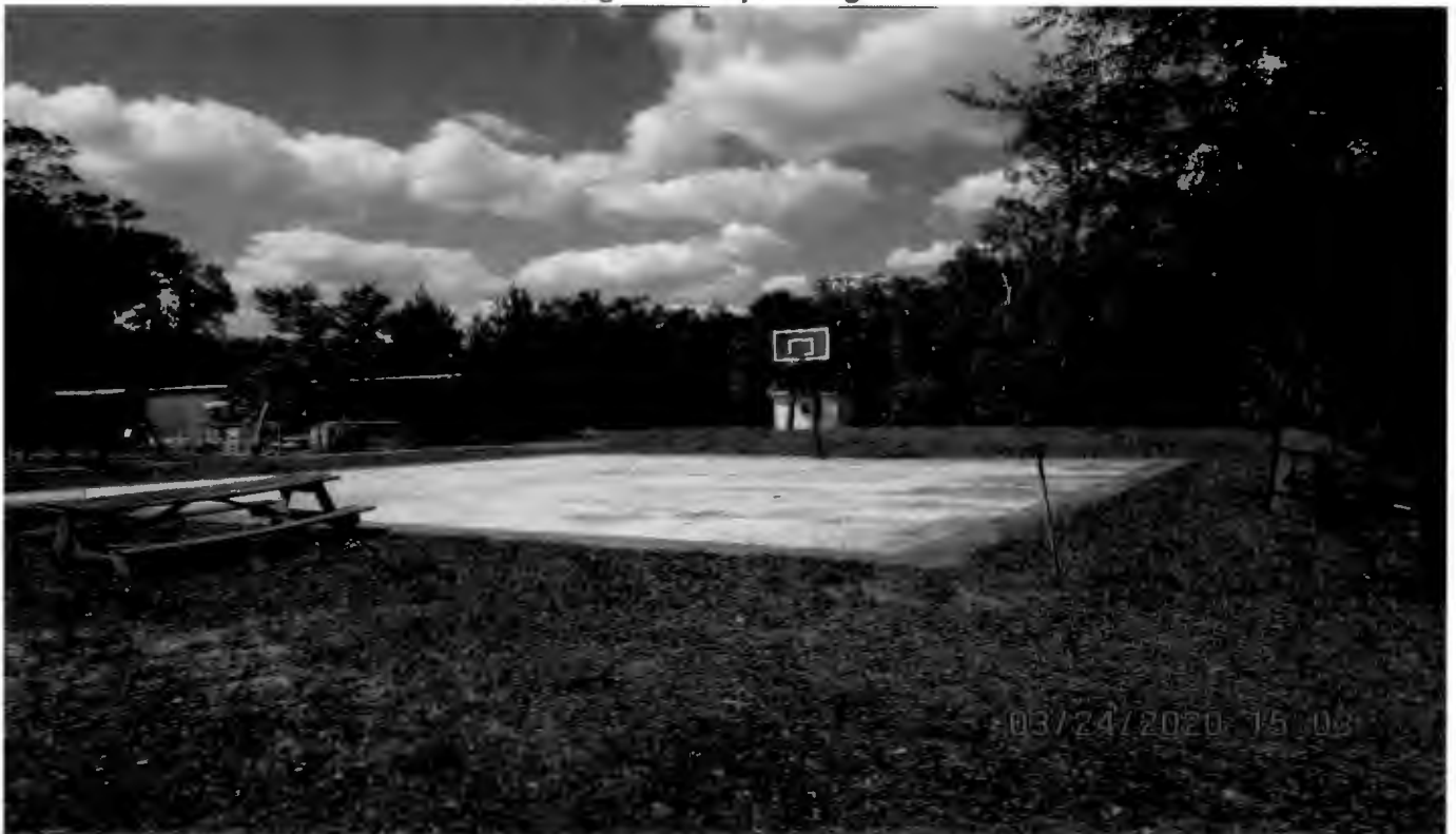
Existing basketball court looking northwest
