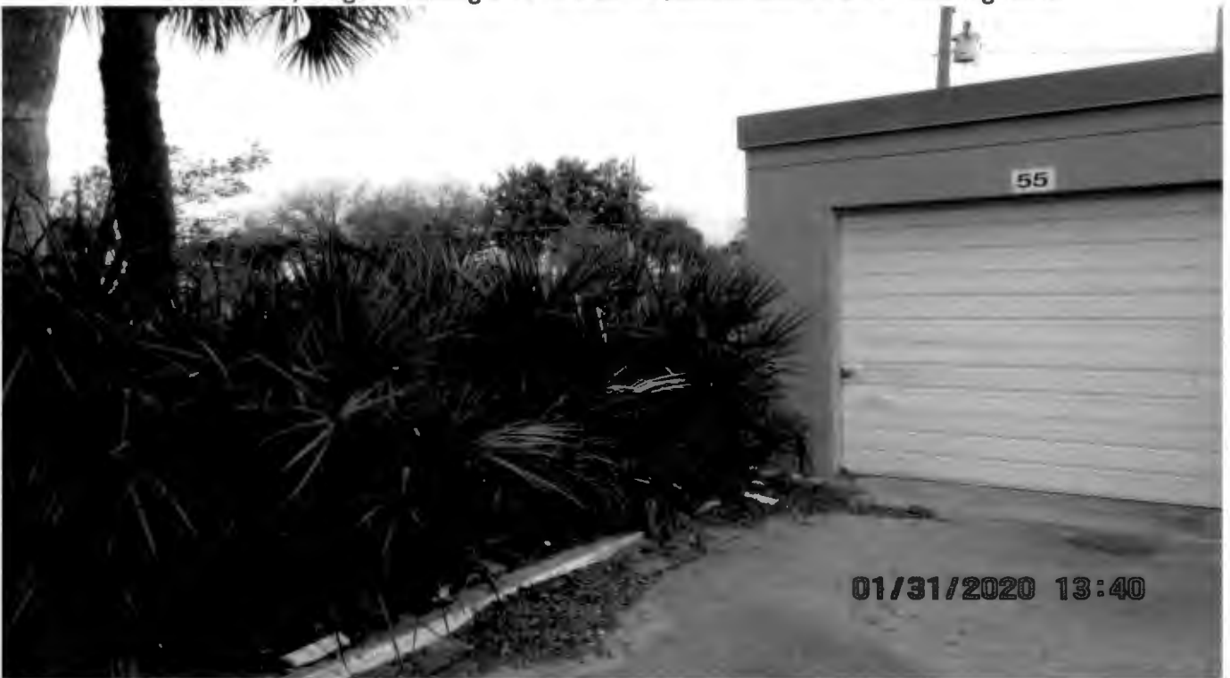
Variance #2; Bldg. G Existing 8.67 ft. Rear Setback in Lieu of 15 ft. Looking North
