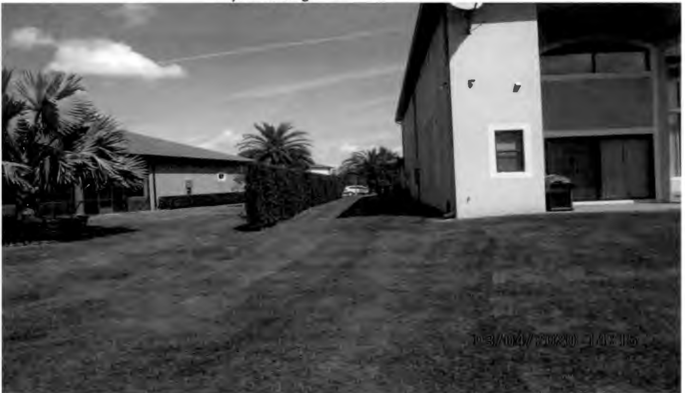
West side yard which was to have been 10 ft. wide rather than 20 ft.
