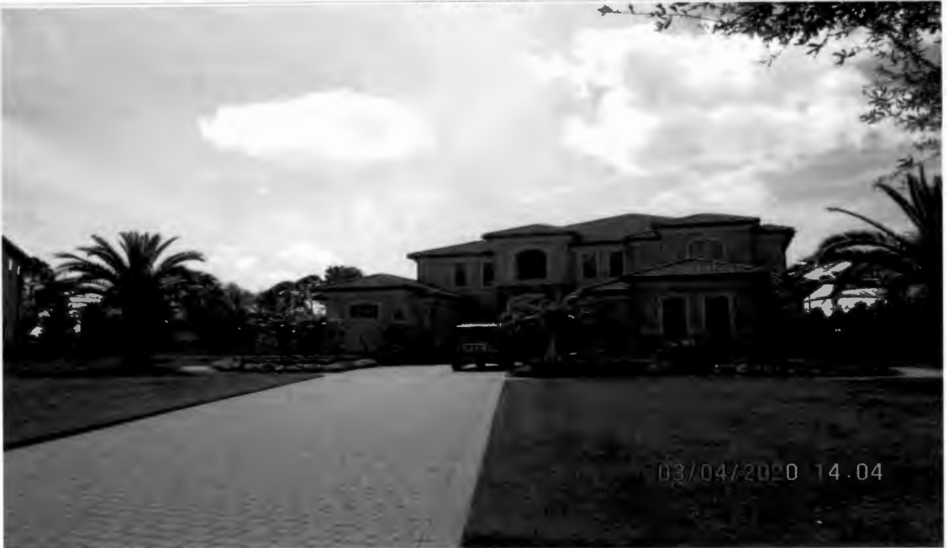
Subject property looking southwest
