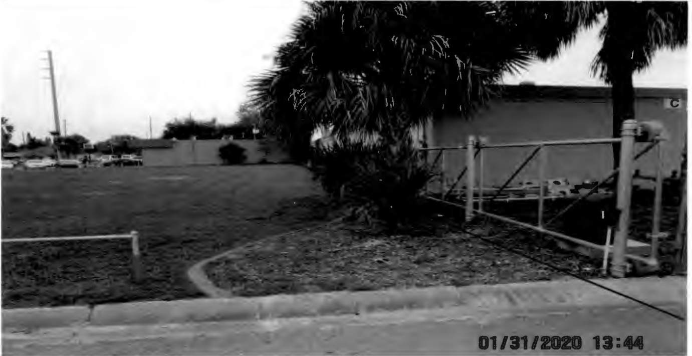
Variance #3; Bldg. F Proposed 3.86 ft. Side Setback In Lieu of 5 ft. Resulting From Creation of Proposed Lot 2 Proposed Property Line in Red
