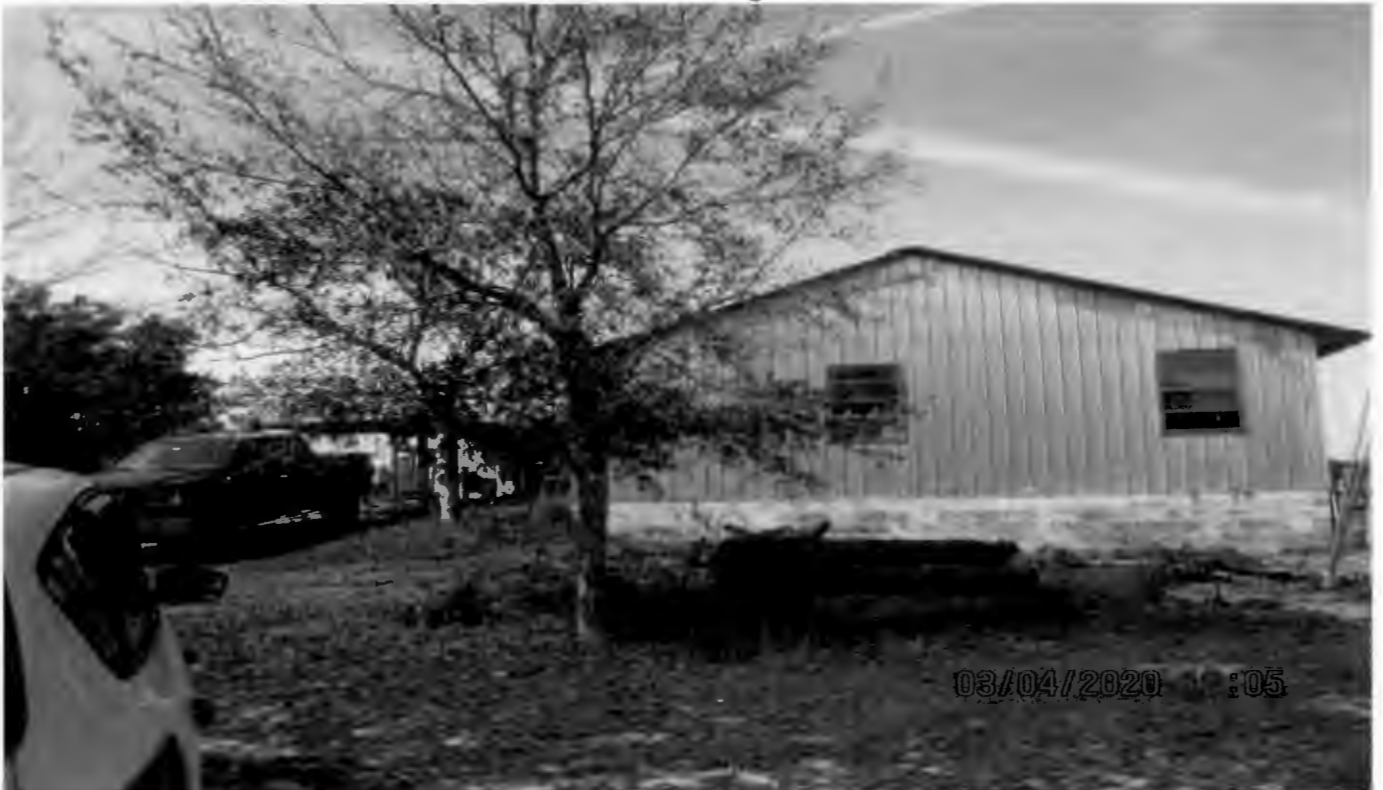
Existing garage to be removed, looking west
