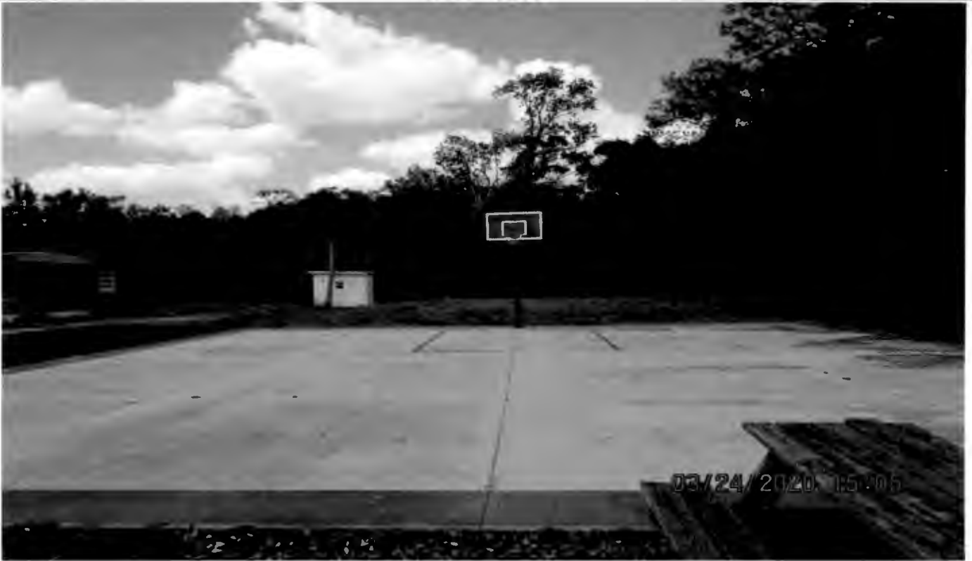
Basketball court looking north, unpermitted shed to left
