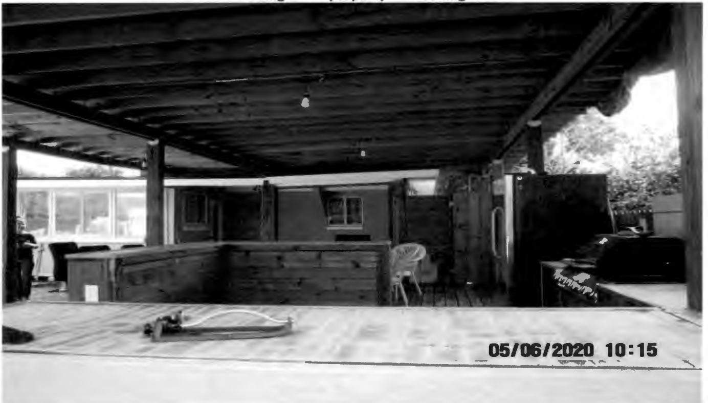
Porch looking east
