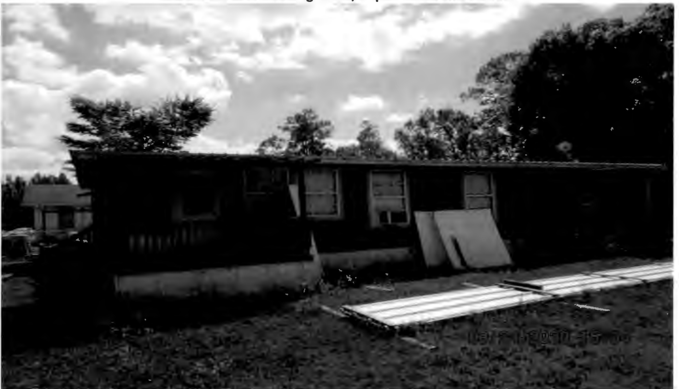
Former night watchman's quarters and parsonage looking south
