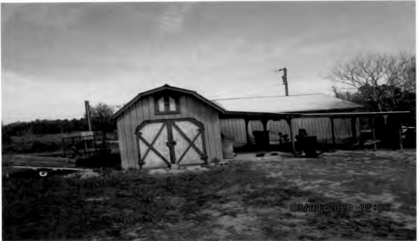
Garage, shed and, lean-to structures to be removed, looking north
