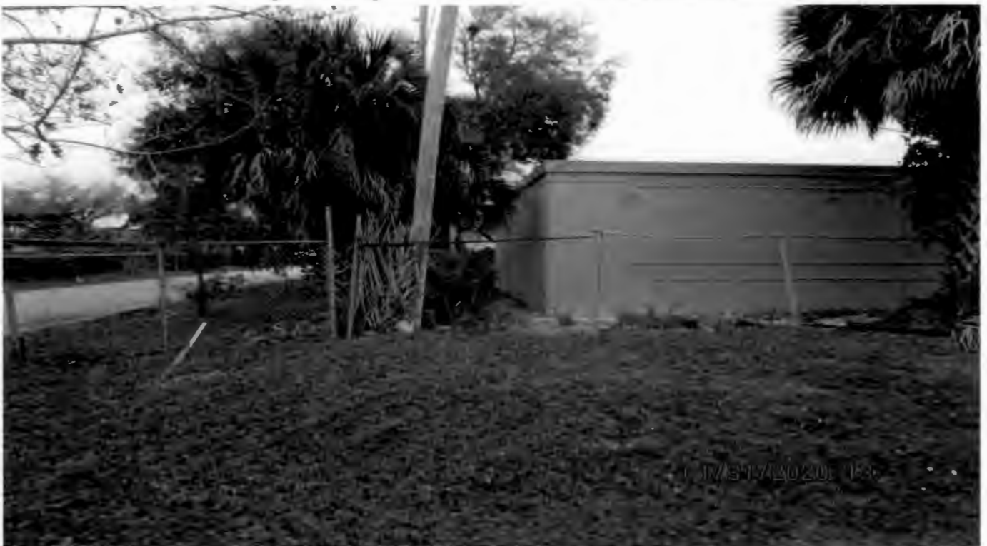
Variance #5; Bldg. H Existing 10.04 ft. Rear Setback in Lieu of 15 ft. Looking North
