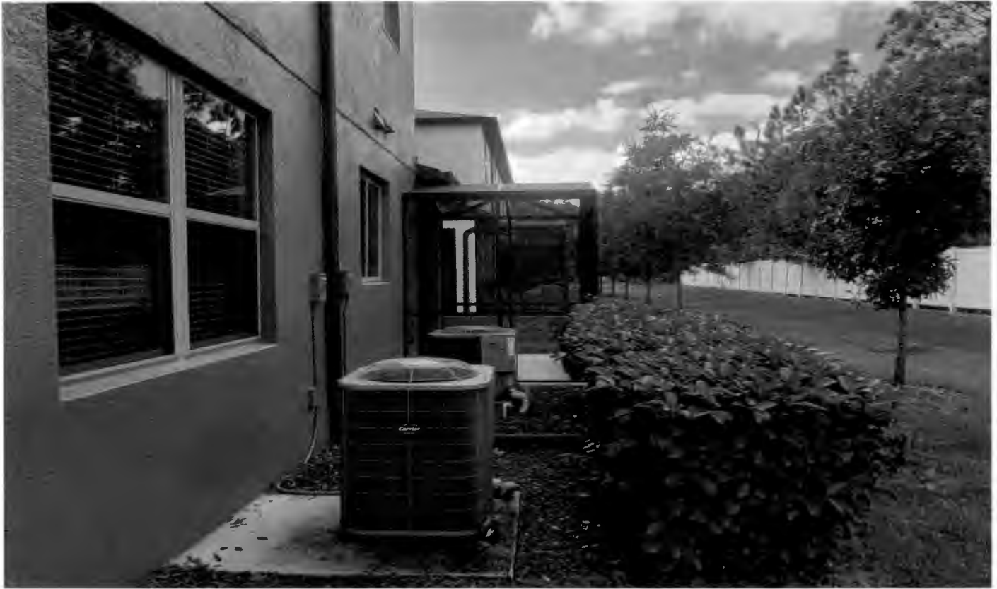
Facing west towards AC units and adjacent screen enclosure
