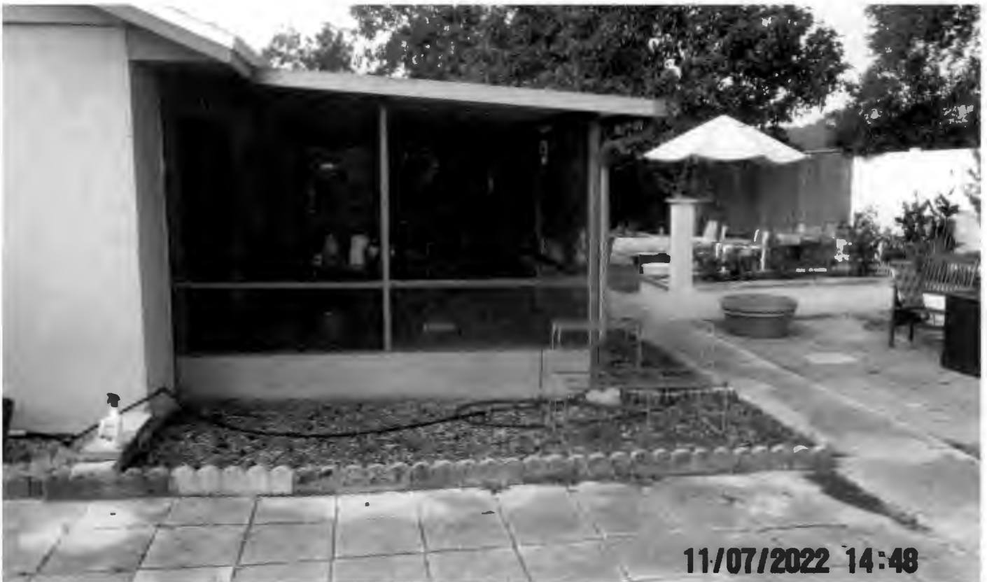
Existing screenroom facing west
