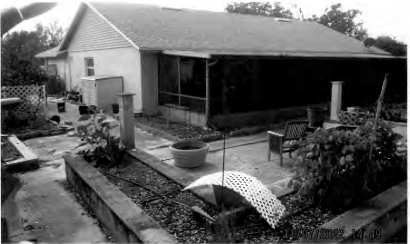
Existing screenroom facing south
