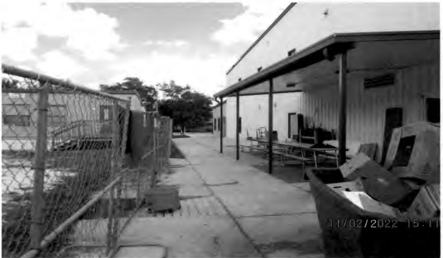
Rear main building, facing east towards the existing covered patio, the proposed patio will be behind
