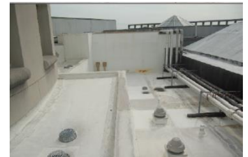
Examples of TPO roof beyond useful life
