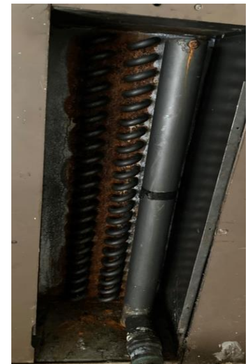
AHU coil is rusted and at end of useful life
