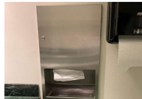
AHU access through bathroom towel dispenser
