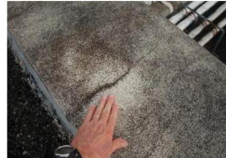
Examples of Bitumen roof beyond useful life
