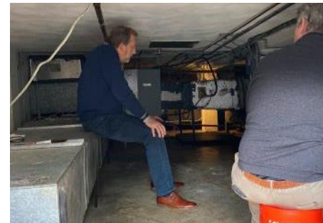
Doghouse mechanical room too small to maintain/repair AHUs
