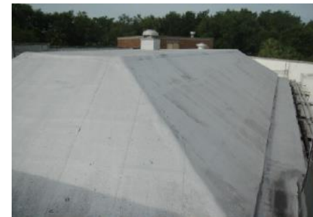
Examples of TPO roof beyond useful life
