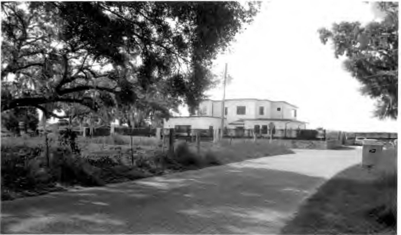
Facing southwest from Siplin Rd. towards Ellerbee St. and front of subject property
