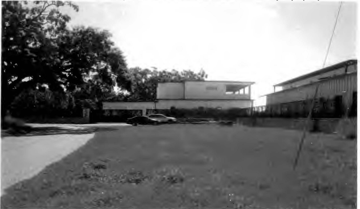
Facing east towards street side of subject property
