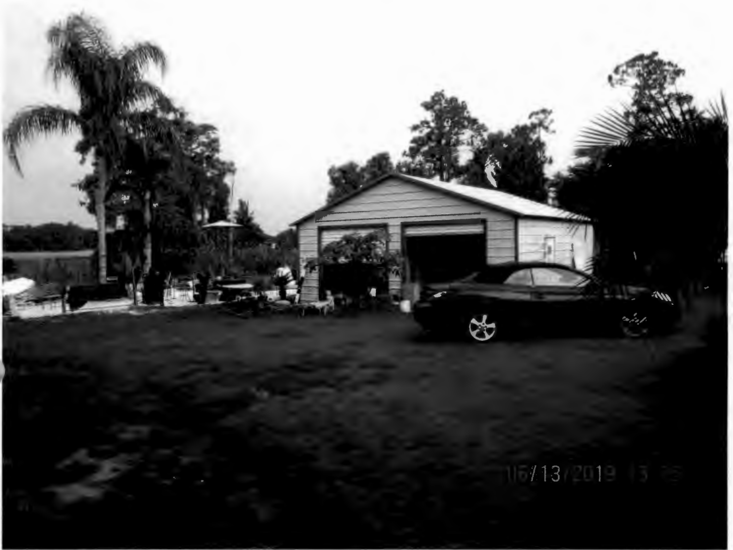
600 Sq. Ft. Shed Looking Southeast
