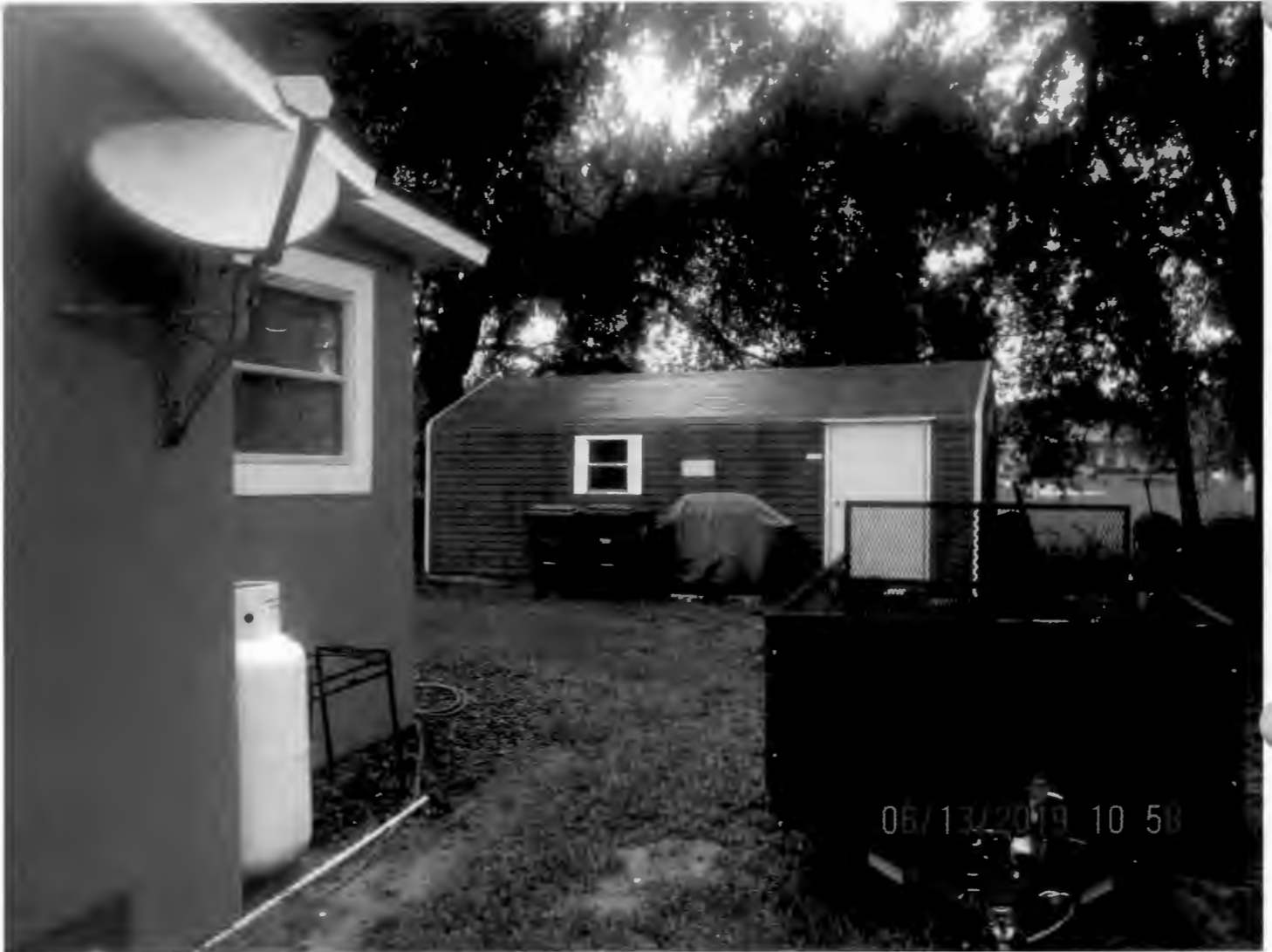
Subject Shed Looking East
