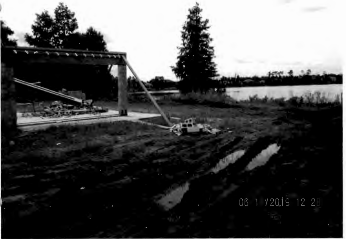
Side area of construction
