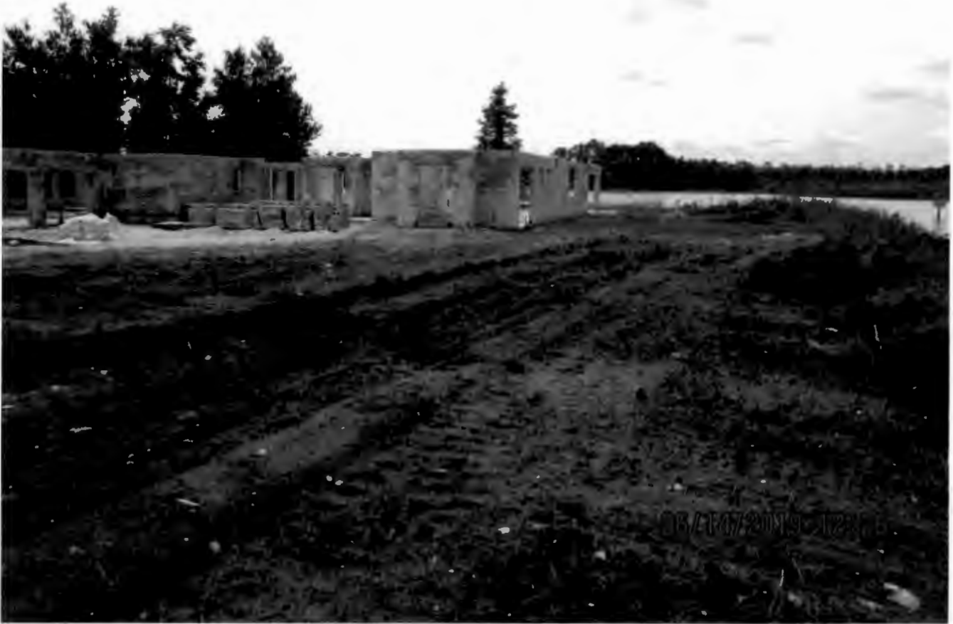
West side looking south
