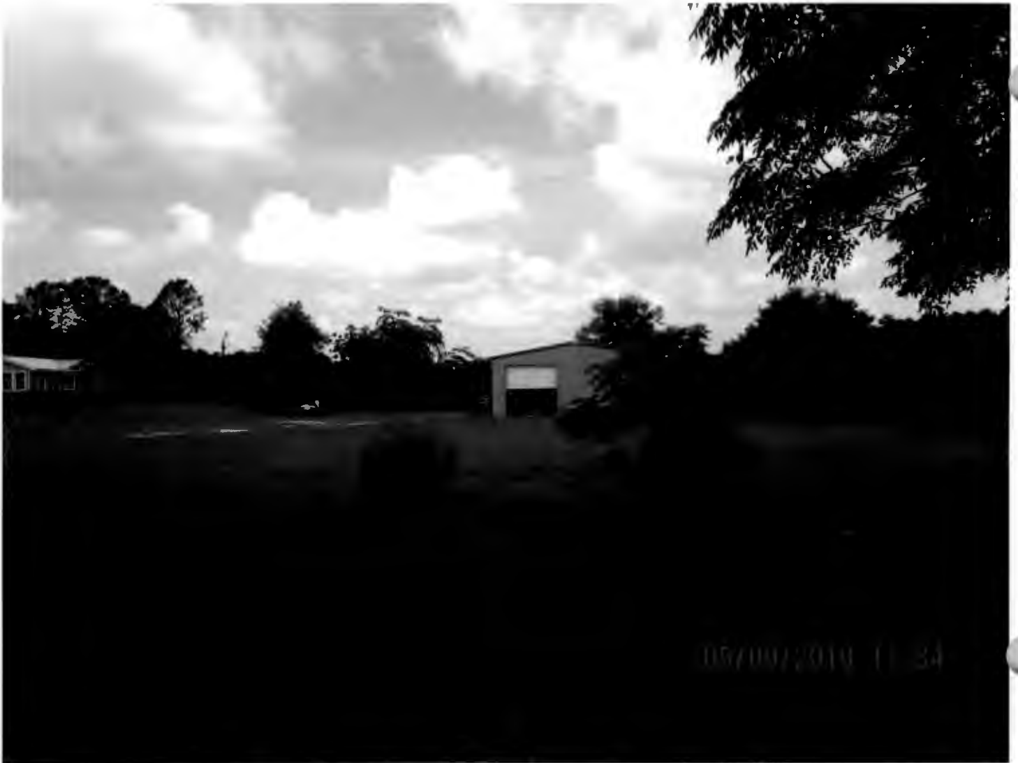
View of Structure from Right-of-Way Looking West
