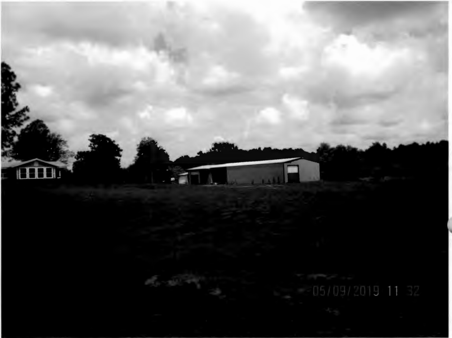
Subject Structure Looking Northwest
