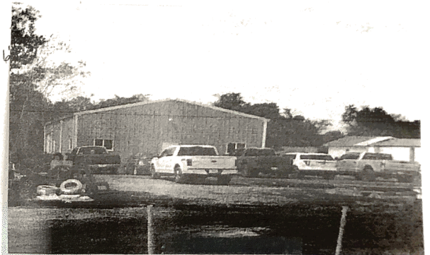
BLDG "C" (3,000 SF) - Built without a building permit by Applicant
