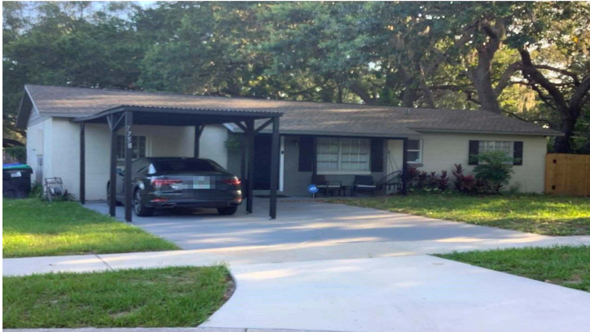
7758 GROVERIDGE CT, UN-INCORPORATED, FL 32810 6/13/2023 8:02 AM
