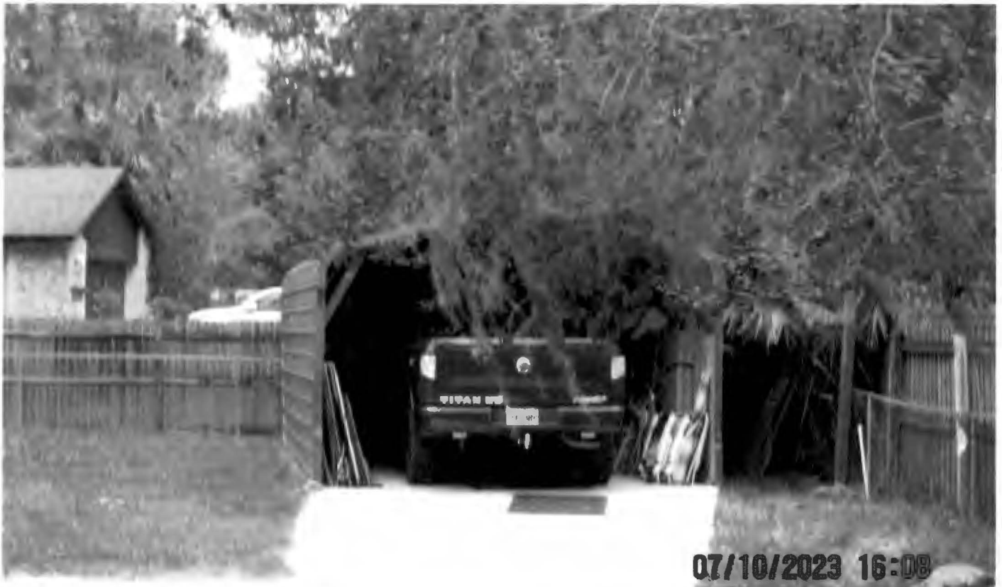
Accessory structure with a 6 ft. front setback facing north
