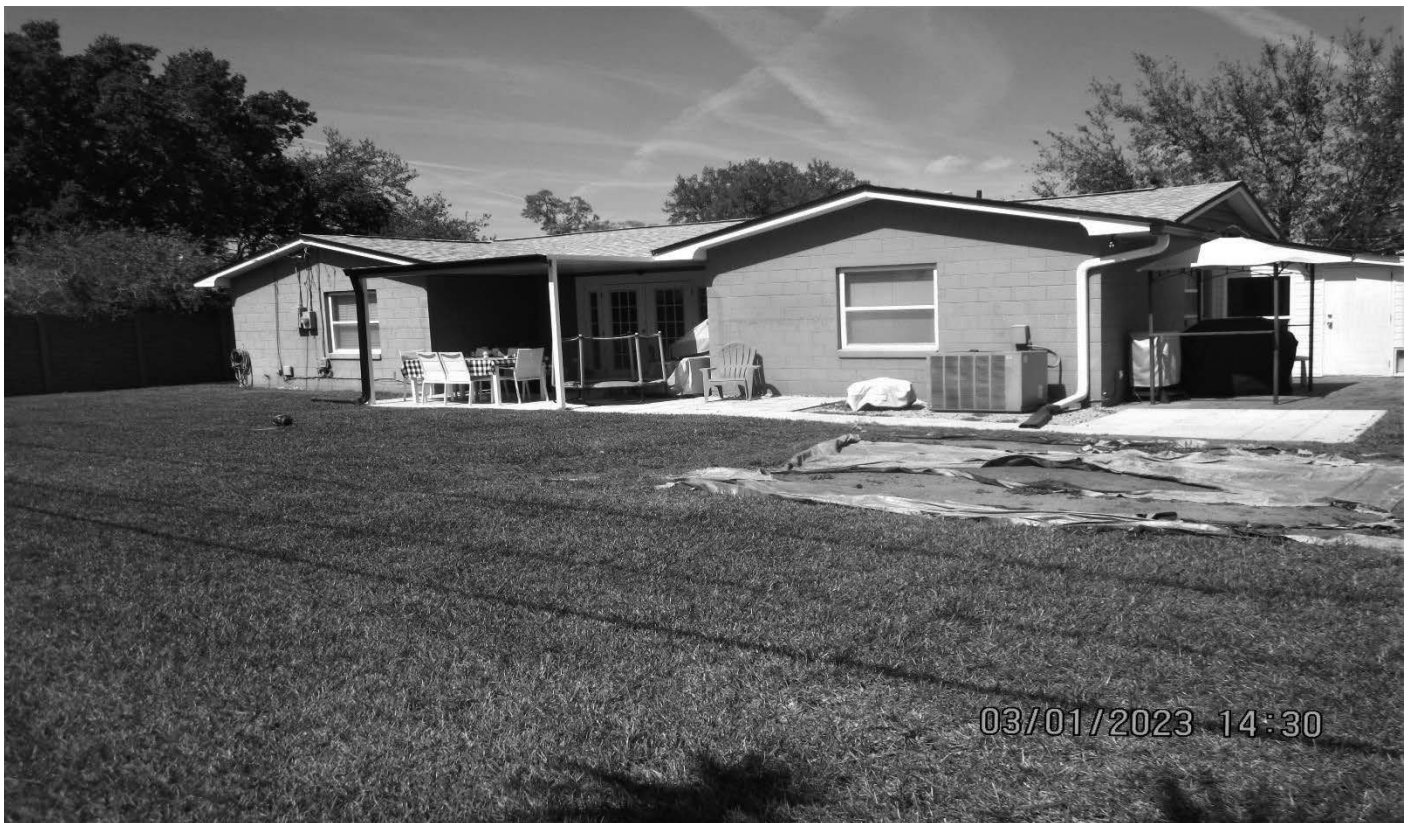
Rear yard, facing northwest towards rear of residence
