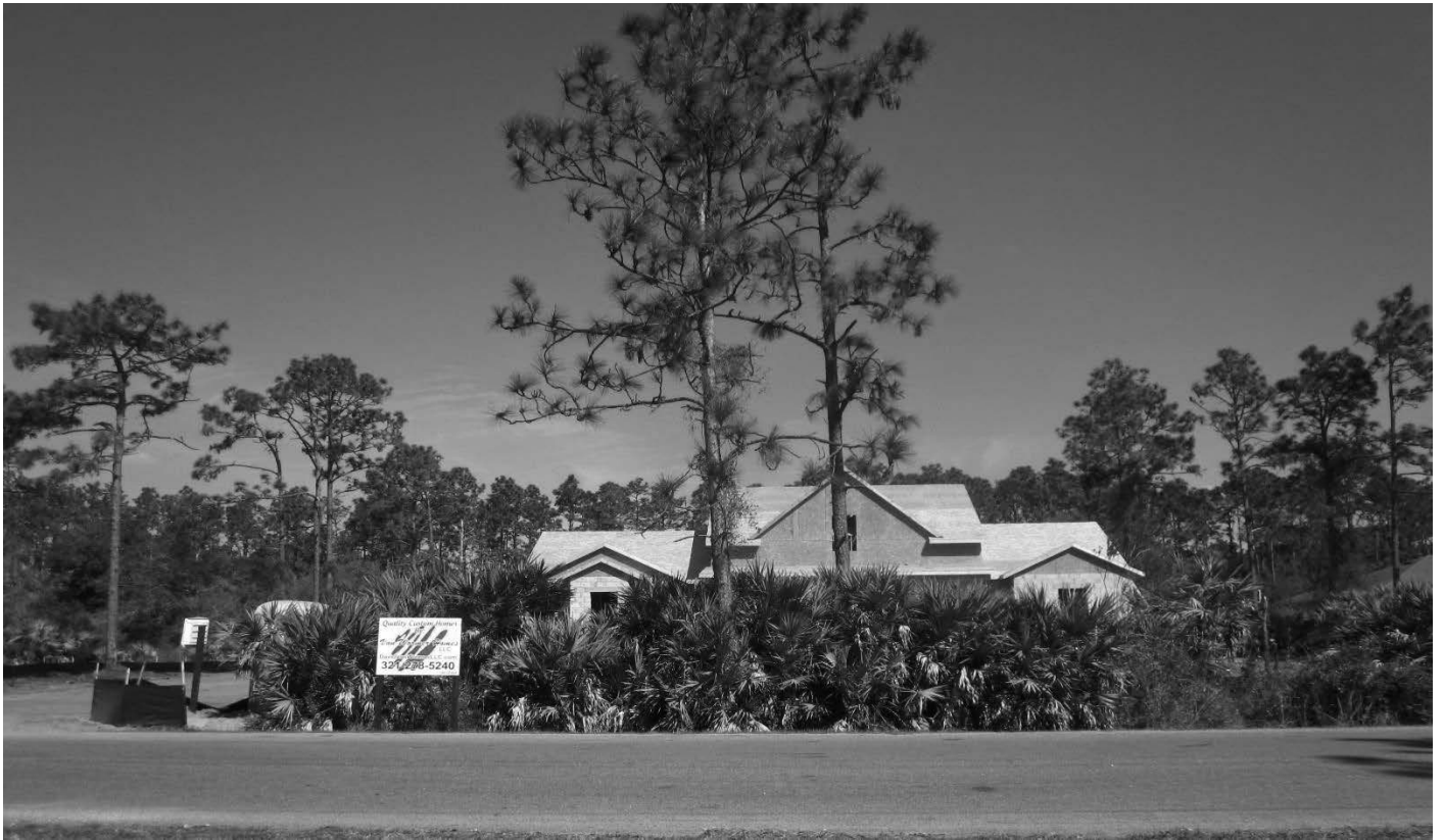
Facing north from Quinella St. towards front of subject property
