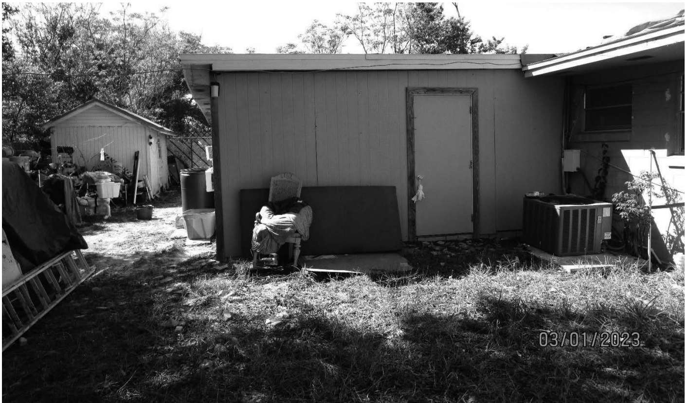
Addition and shed facing west
