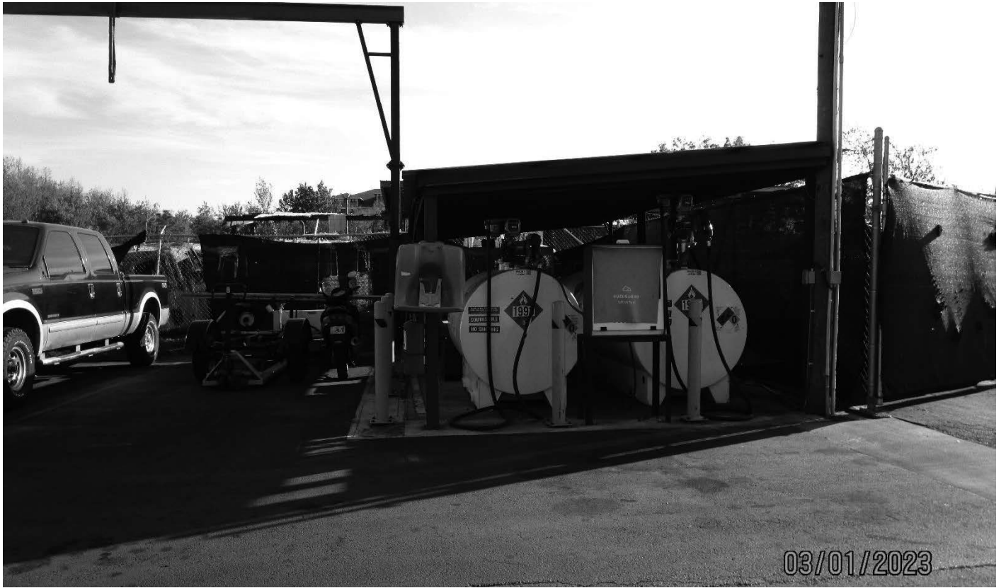
Building #5 to be removed facing south
