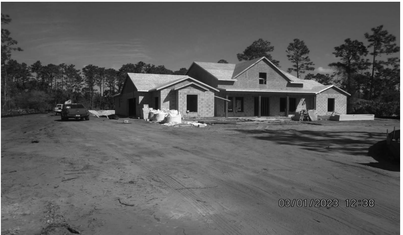
Facing northeast towards partially constructed primary residence
