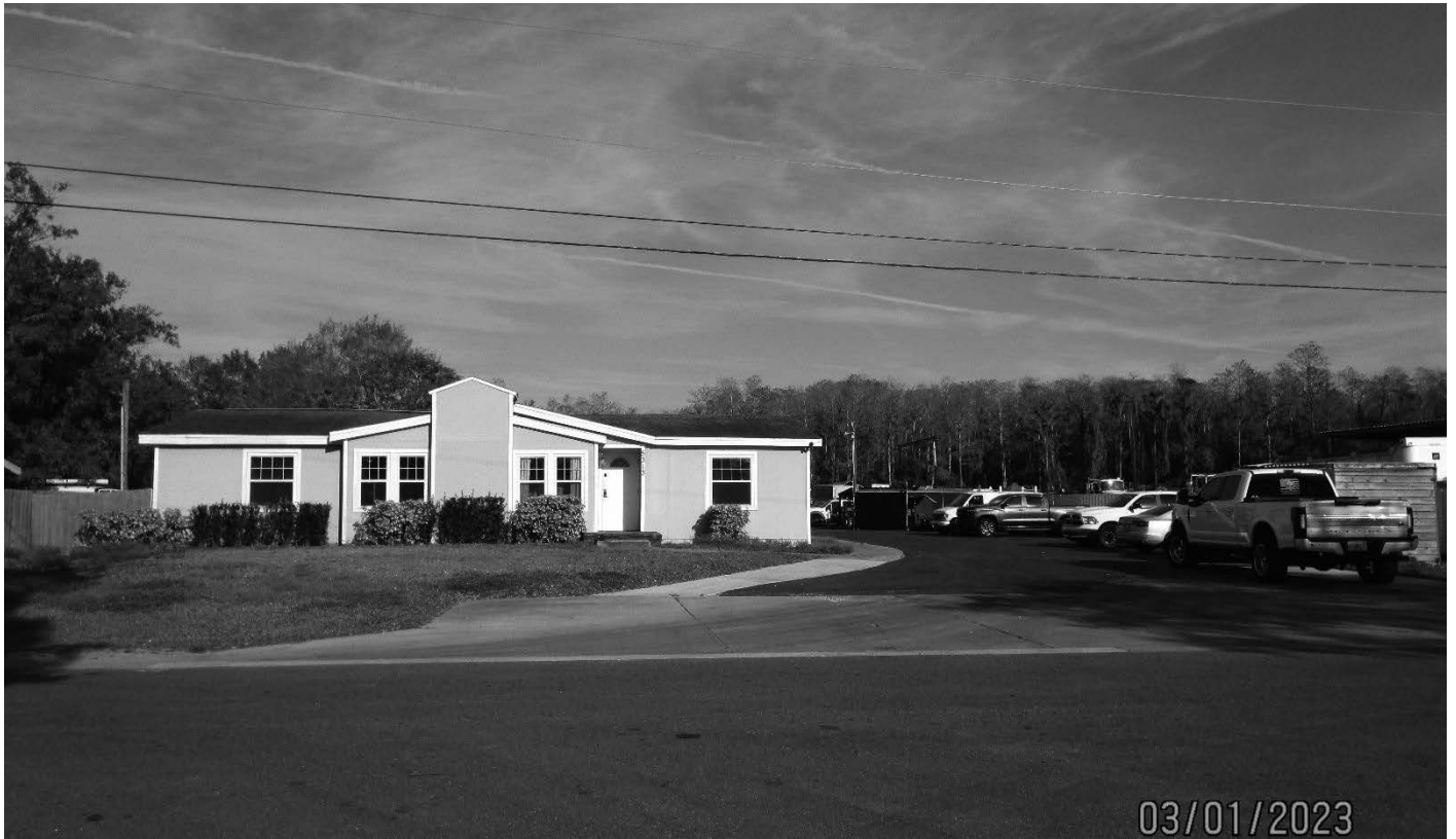
From Patch Rd. facing E towards Building #1 with side setback, Variance #2 and front setback, Variance #3
