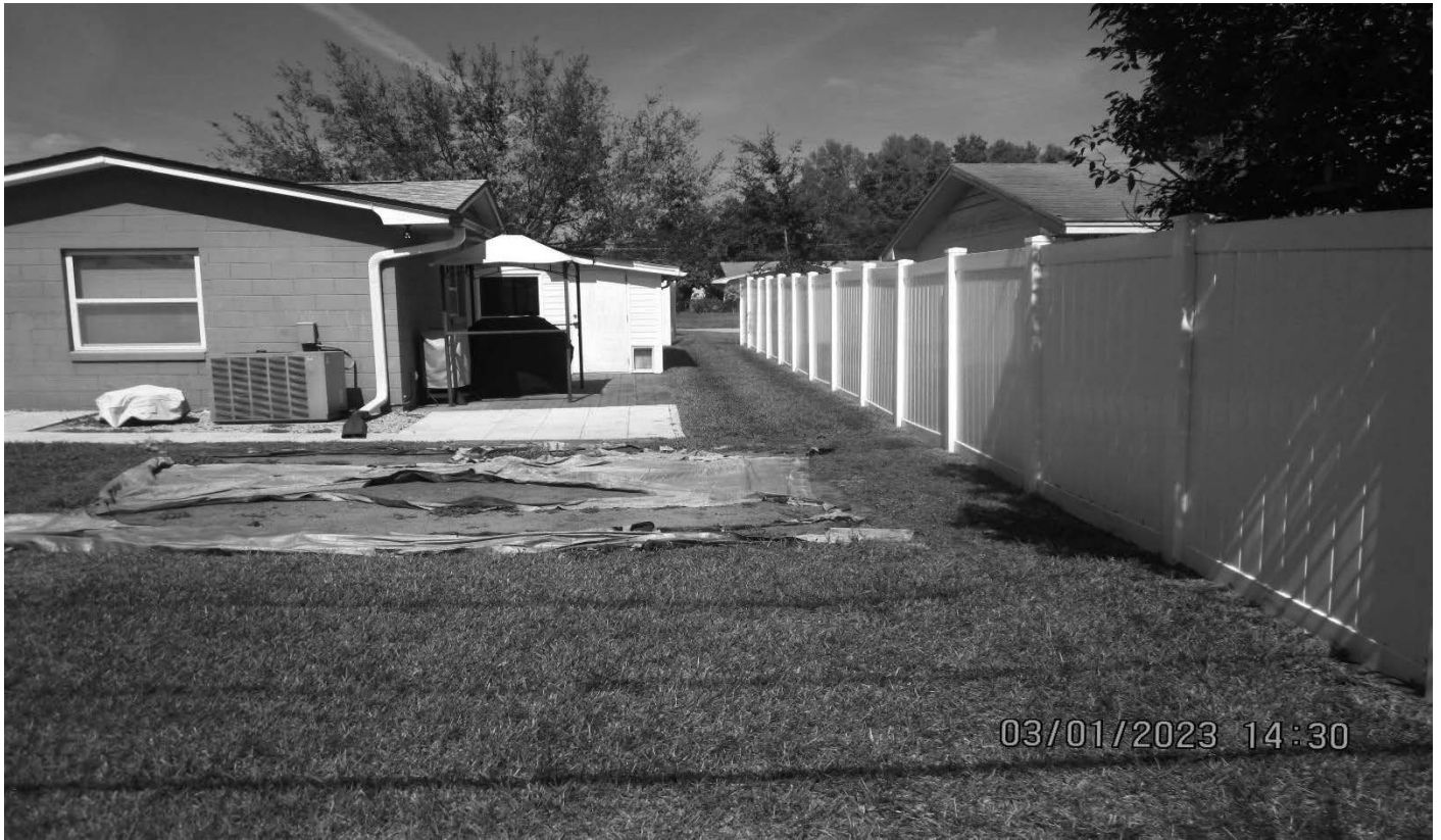
Rear yard, facing north towards proposed addition location to line-up with existing residence
