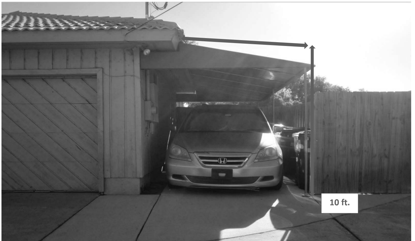
Facing east from Ohio St. towards front of carport
