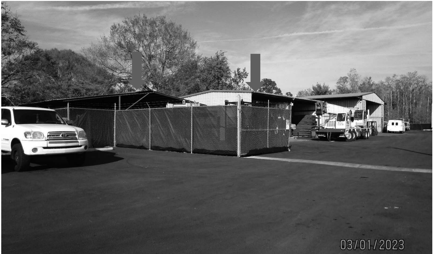
Buildings #3 and #4 to be removed facing east
