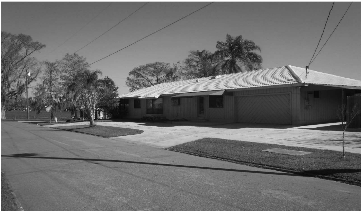
Facing north from Ohio St. towards side of property and carport
