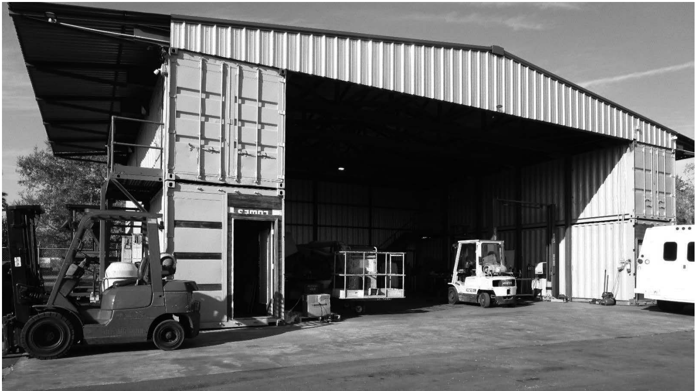
Facing north towards Building #2 to remain
