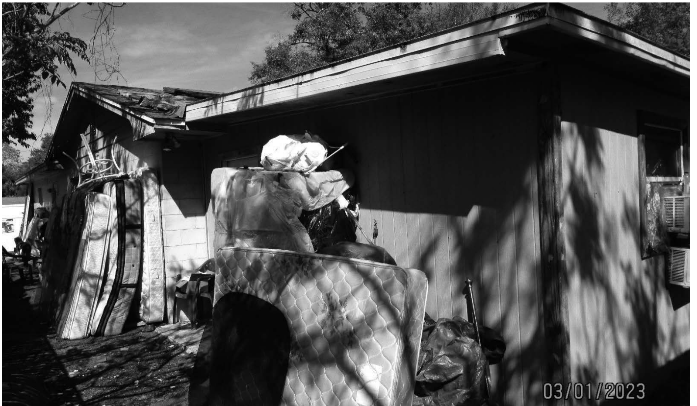
Addition facing east
