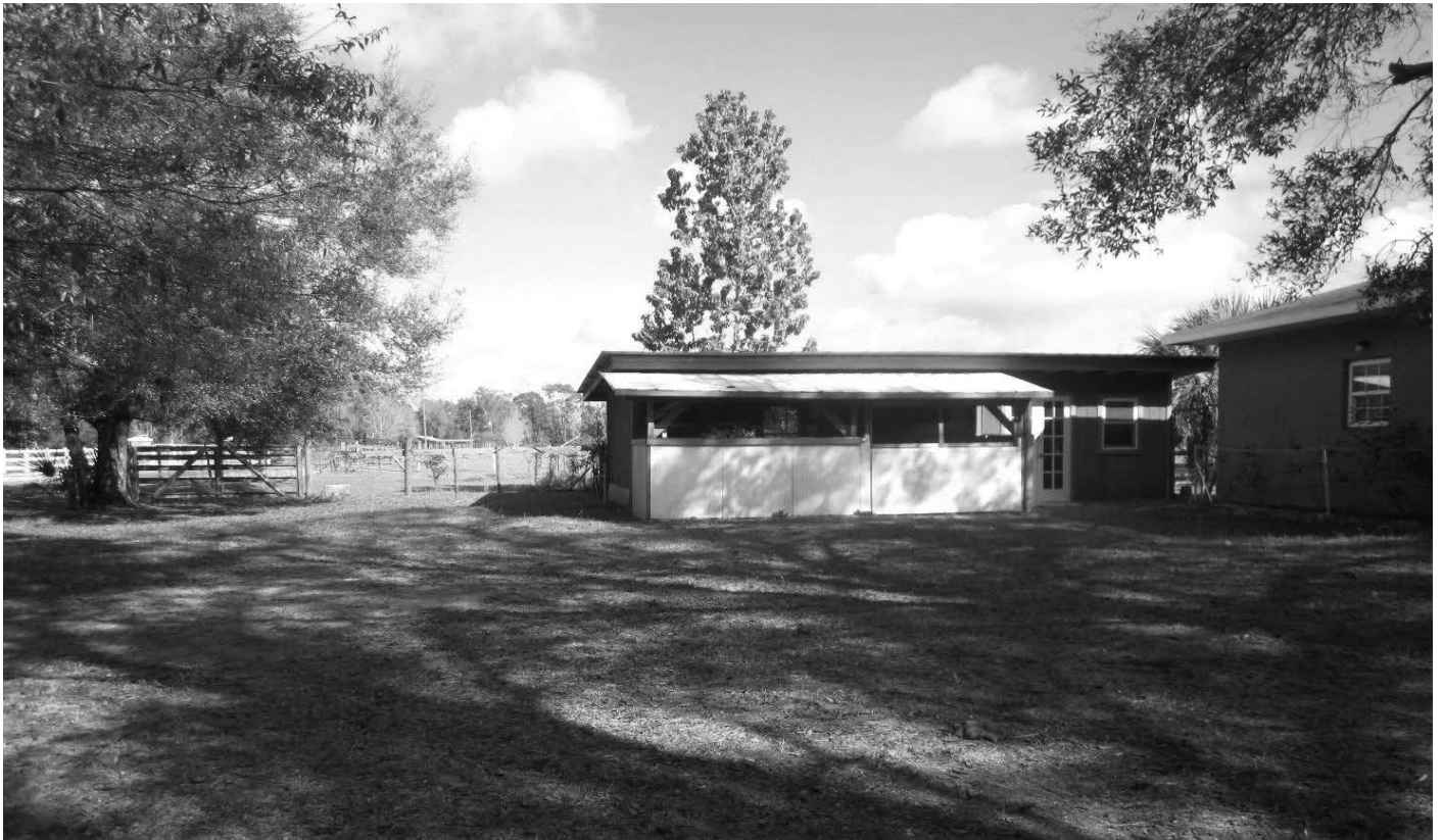
Side yard, facing north towards existing Shed #1
