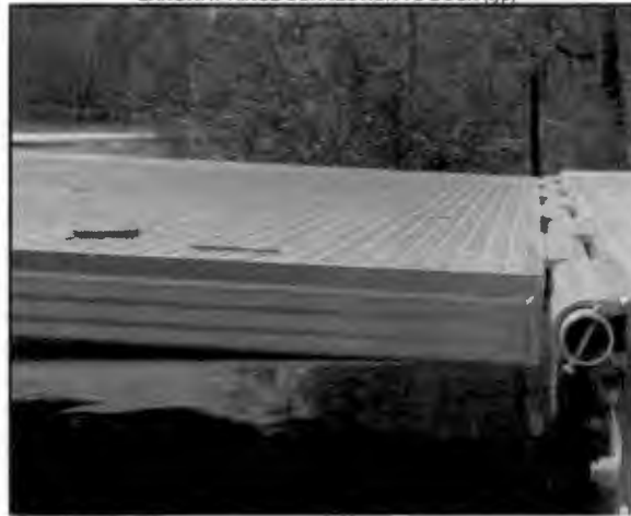
GANGWAY HINGE CONNECTION TO DOCK (typ)
