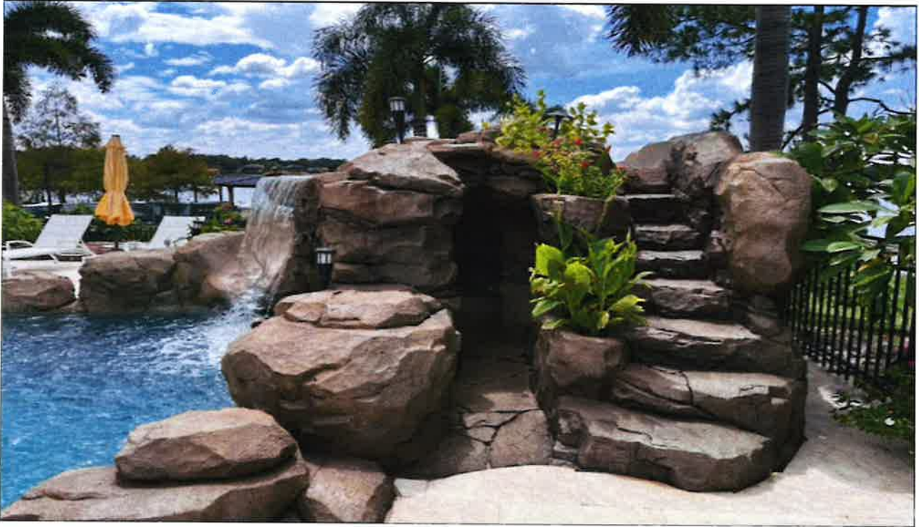
Unpermitted accessory structure, part of the pool deck, facing west
