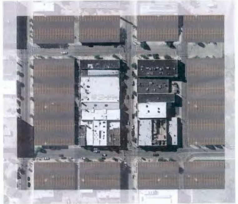
This is what one block of charming Old Town Pocatello, Idaho would look like if it had to follow modern day parking requirements. See more examples here.
