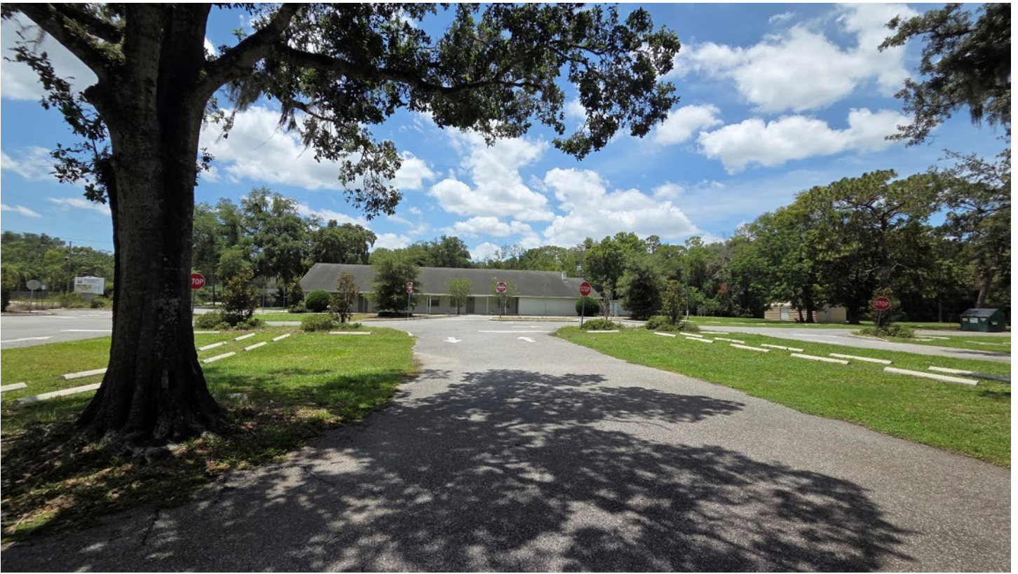
Parking area, facing south showing paved drive aisles with grass parking
