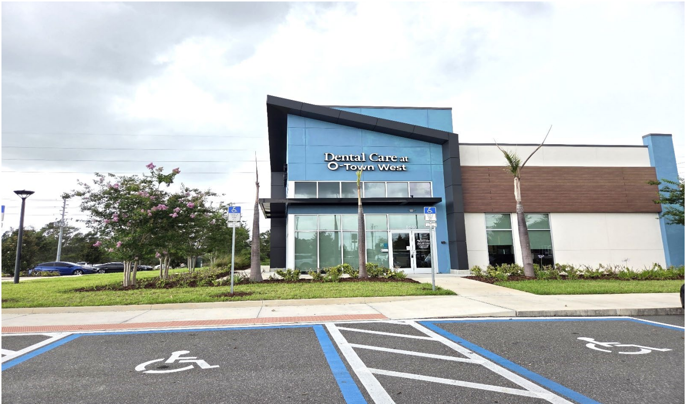
Facing west towards the dental office main entrance
