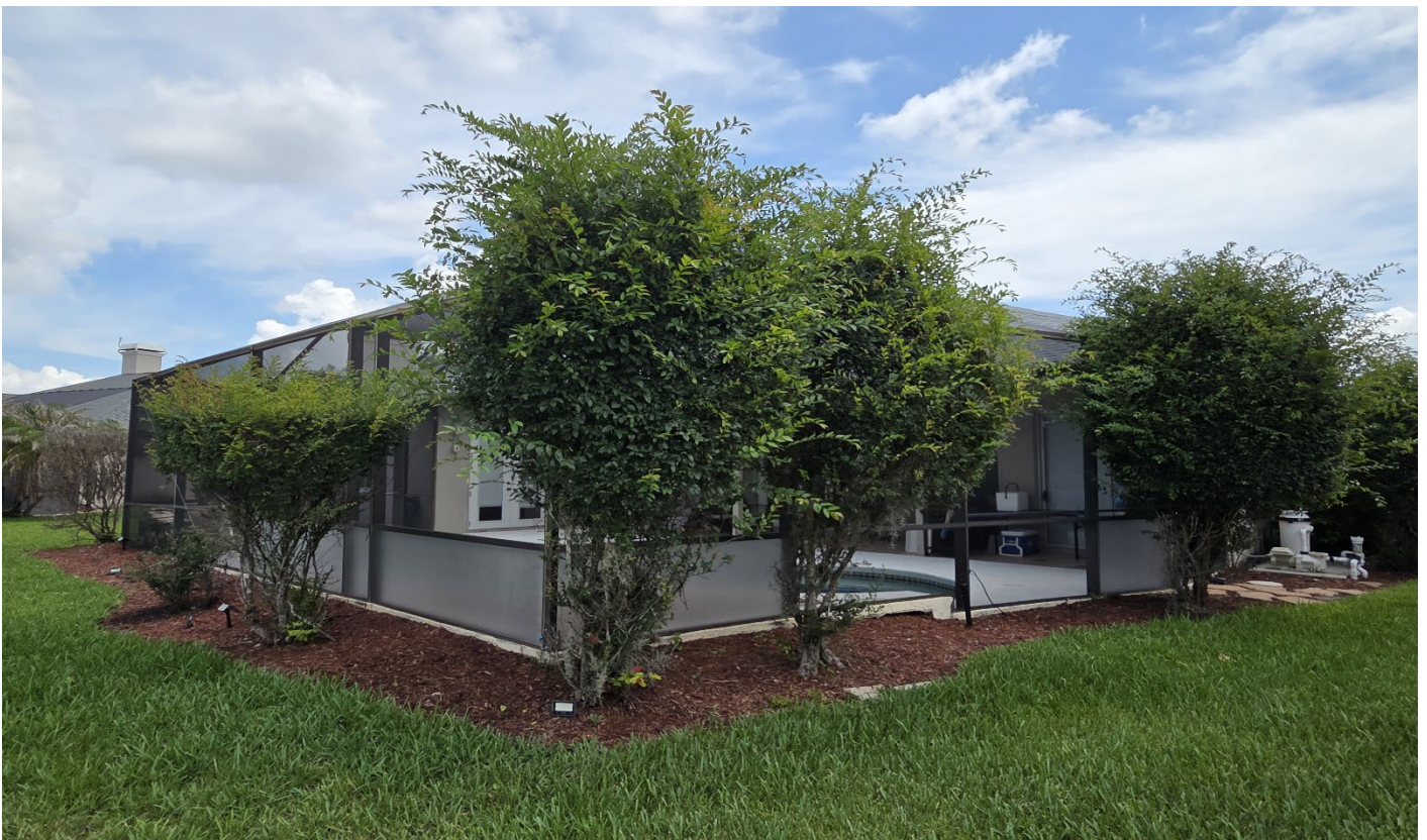
Rear yard, facing north towards the screen enclosure
