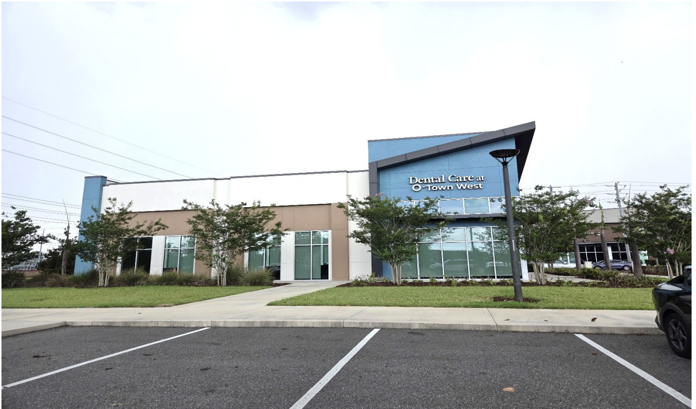
Facing north towards existing dental office
