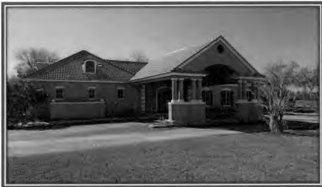
View looking south at the former Eastwood golf course clubhouse. (Photo No. 2)
