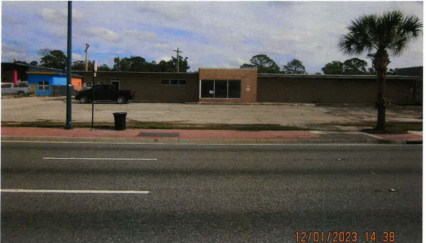
Property from S. Orange Blossom Trl. facing east with existing building to be demolished
