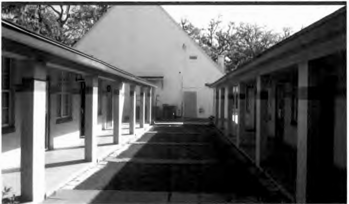
Courtyard, facing east towards classrooms and rear of chapel
