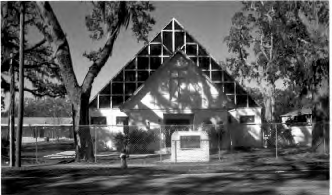
Facing west from Mott Ave. towards front of chapel
