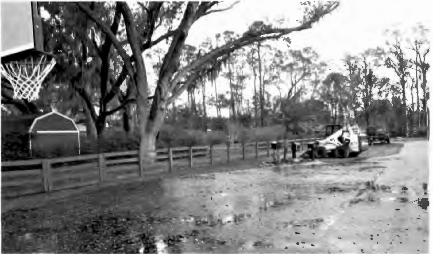
Facing northwest from Shady Oak St. east towards side of storage structure
