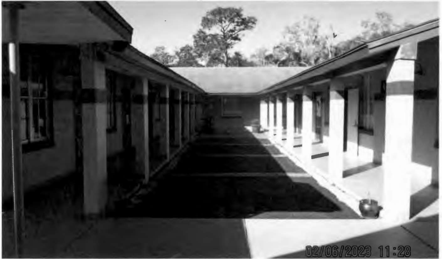
Courtyard, facing west towards classrooms
