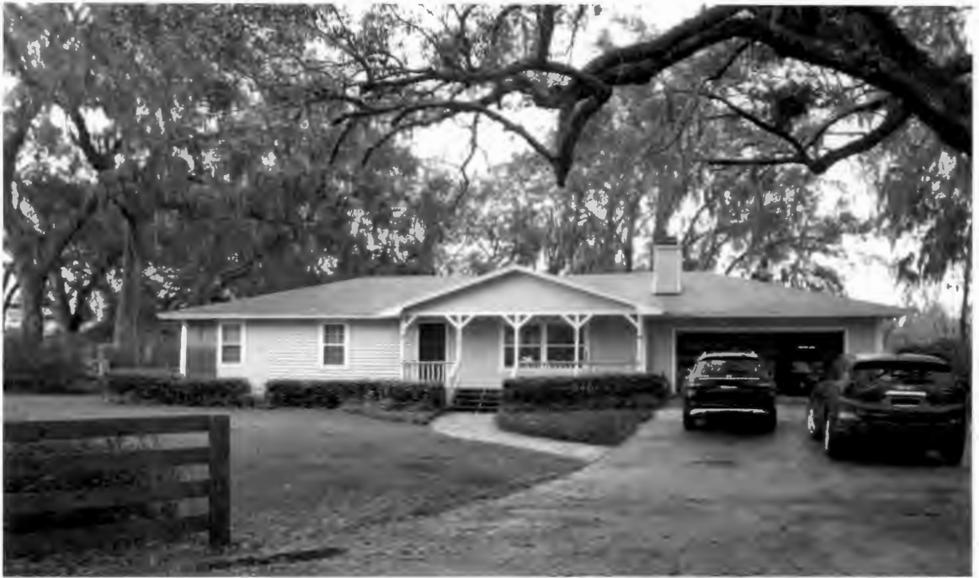
Facing south from Shady Oaks St. north towards front of residence
