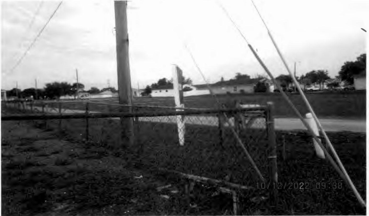
Facing northwest from southeast property line towards sanctuary expansion from S. Goldenrod Rd.
