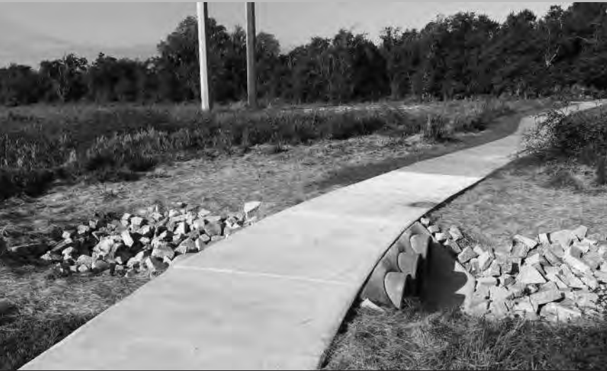
Sidewalk Repairs at Fishhawk Ranch CDD
