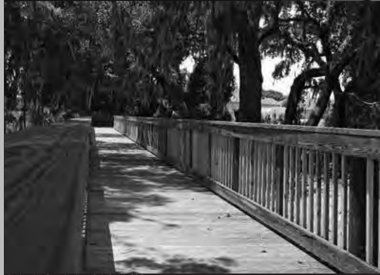
Pedestrian Boardwalk at Oak Creek CDD
