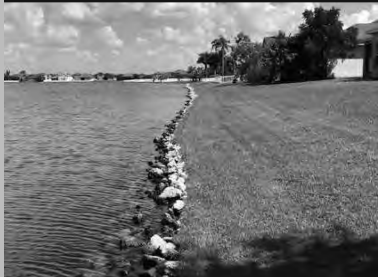
Pond Bank Restoration at Mira Lago CDD
