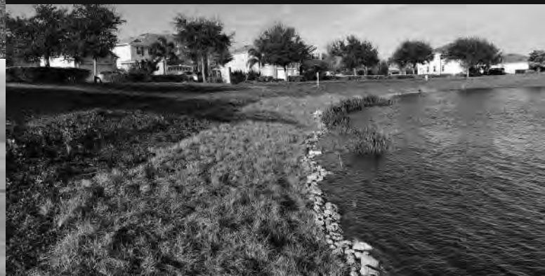
Pond Restoration at Harbour Isles CDD
