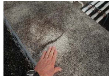
Examples of Bitumen roof beyond useful life
