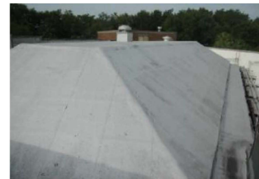
Examples of TPO roof beyond useful life
