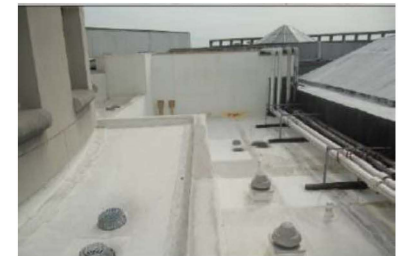
Examples of TPO roof beyond useful life
