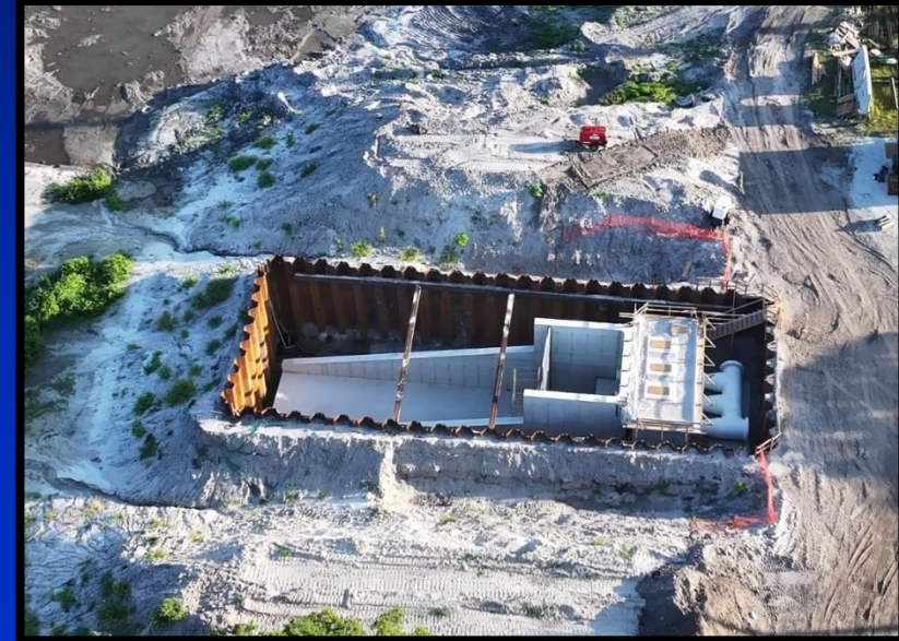
Photo 10 - Pump Station Concrete Structure
