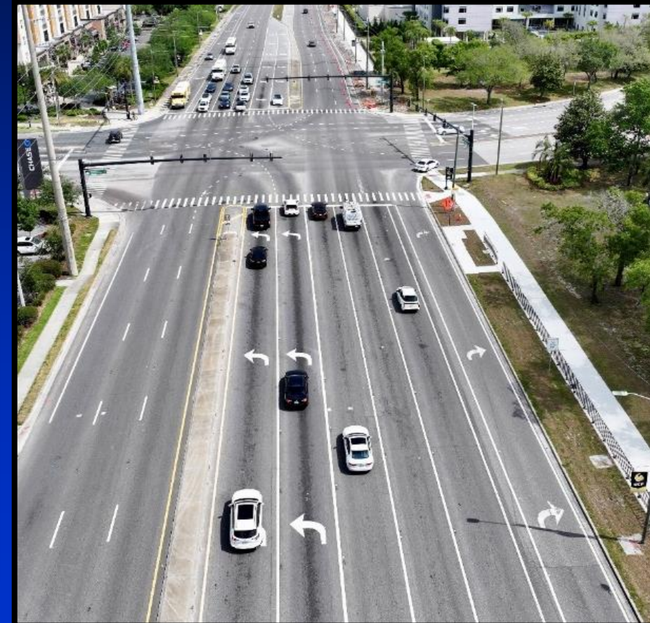
Pedestrian Fencing installed along Alafaya Trail at University Boulevard
