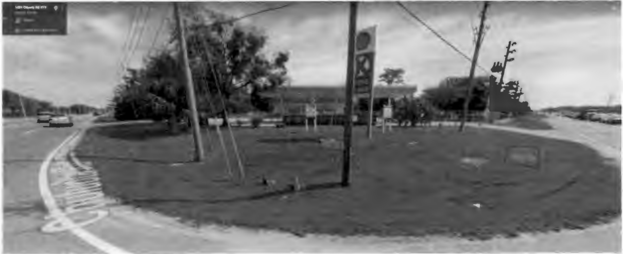
Existing inlet on east side of Chuluota Road drains into FDOT SR 50 ROW
