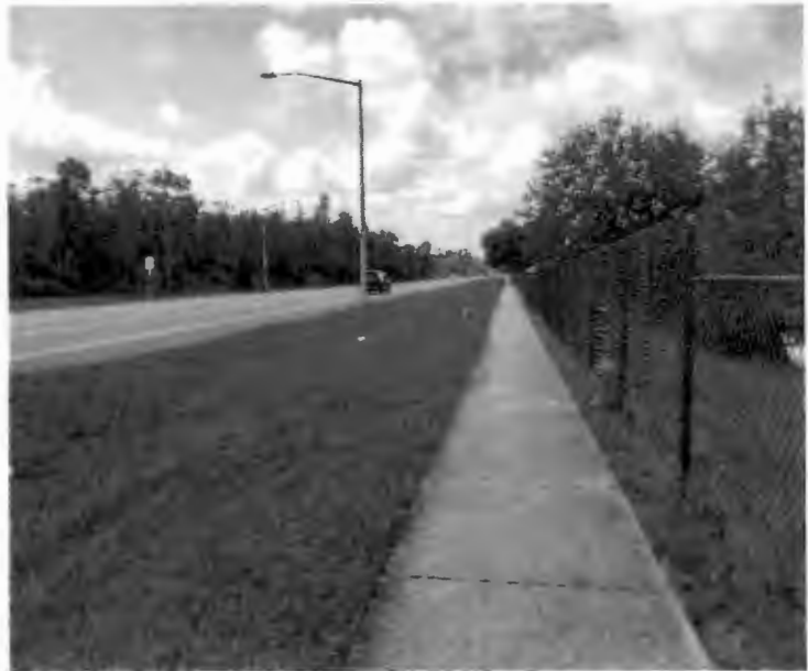
Roadside ditch facing south
