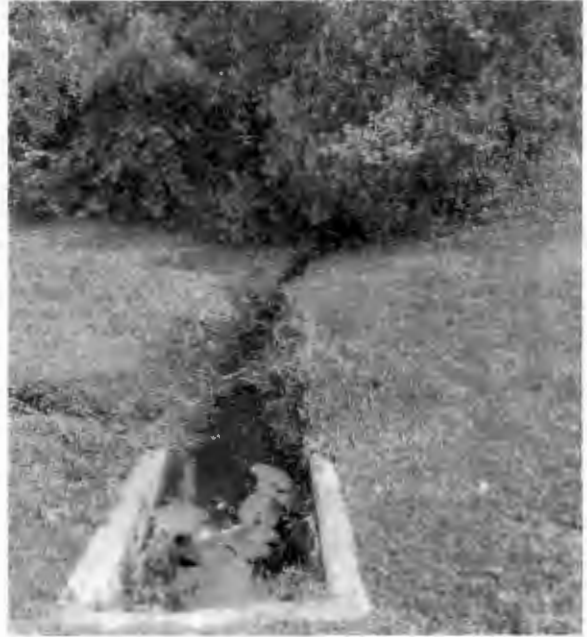
Existing side drain under Corner Lake Drive which conveys runoff from Basin 2B to Basin 3
