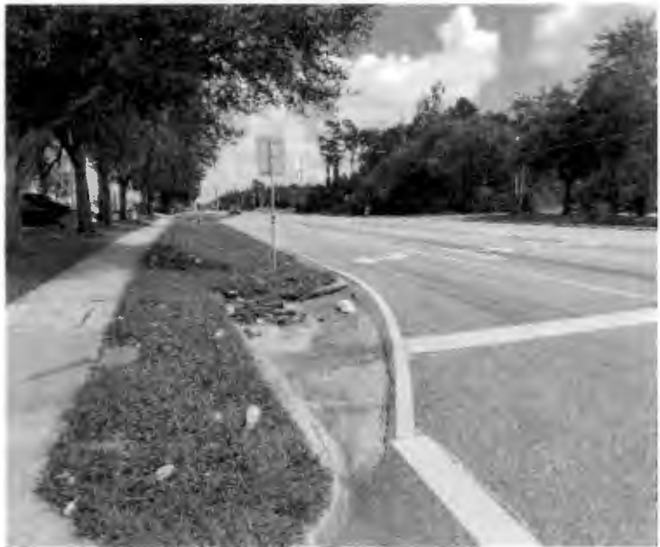
Existing inlet drains west into FDOT SR 50 ROW
