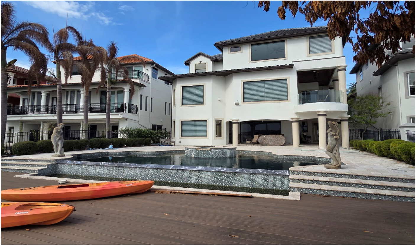
Rear yard, facing north towards pool area
