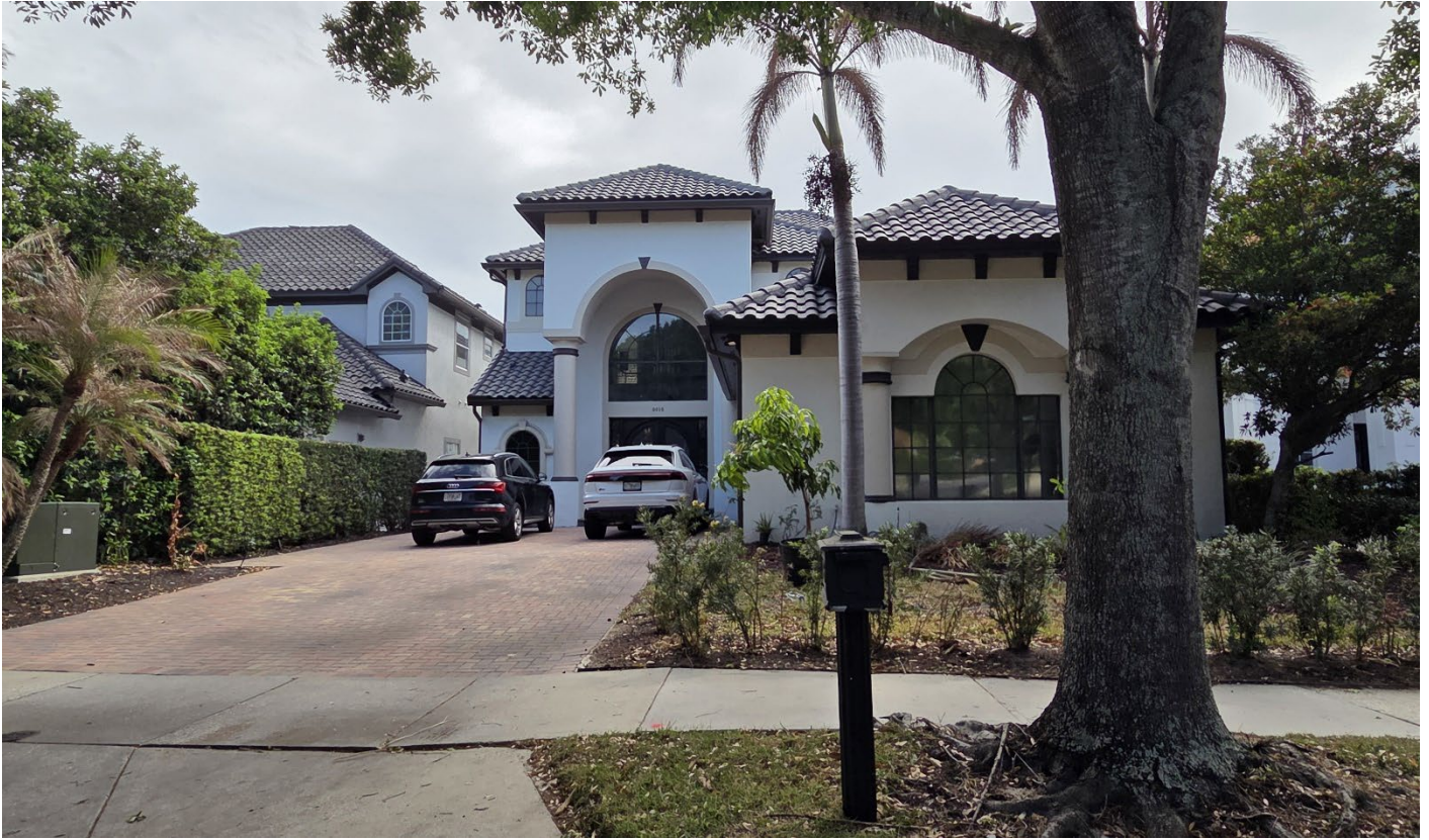
Facing south towards front of subject property
