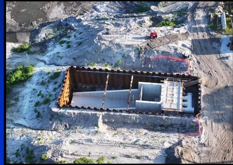
*Photo 10 - Pump Station Concrete Structure*
