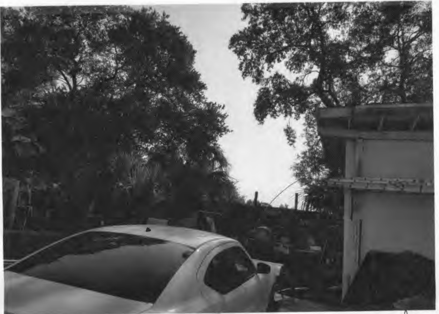
After Demo is done Left Side of Shead.
