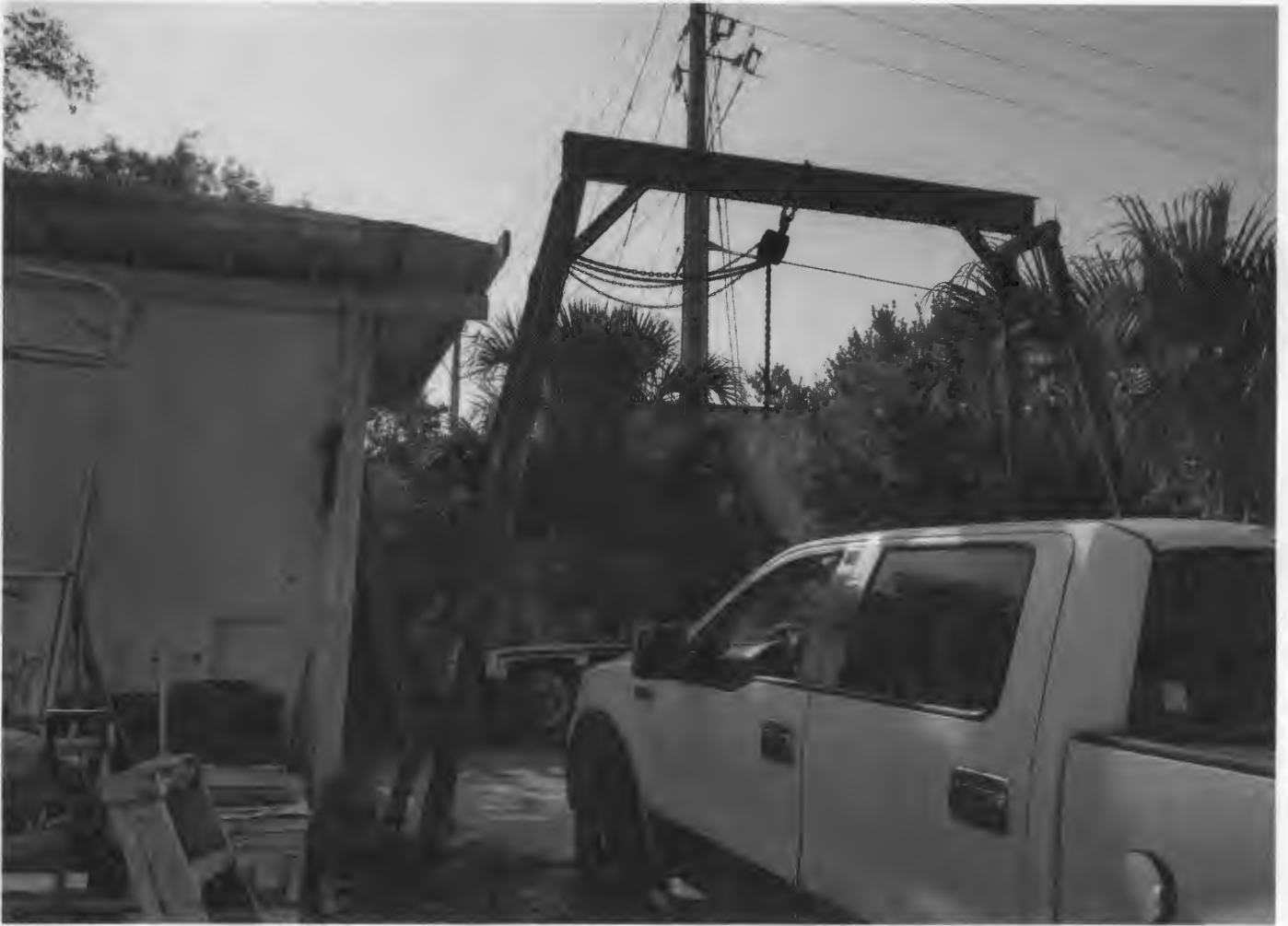
After Demo is done. Right Side of Shead
